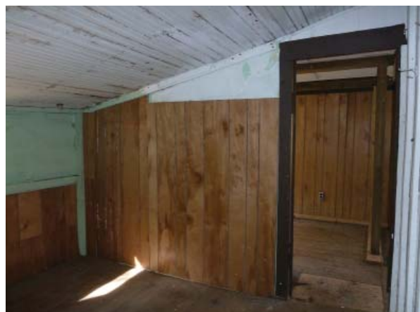
Figure 84. Northwest oblique of Storage Room (Room 106).
