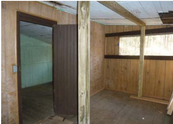
Figure 80. Southwest oblique of Northwest Bedroom (Room 105).
