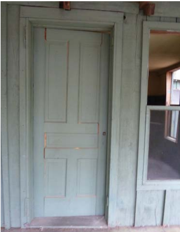
Figure 59. North door of front elevation.
