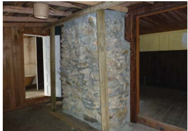
Figure 67. Living Room Extension (Room 101) looking northwest.
