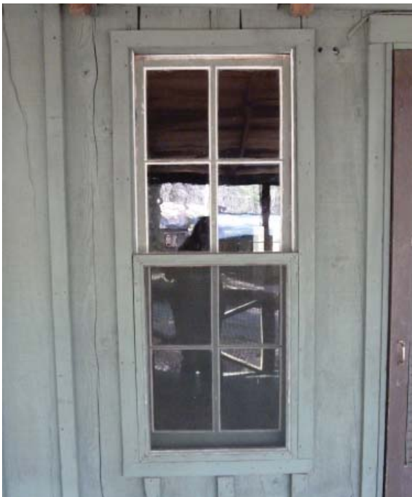
Figure 62. Typical original window on the east elevation.
