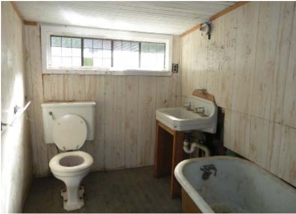
Figure 96. Bathroom (Room 109) looking south.
