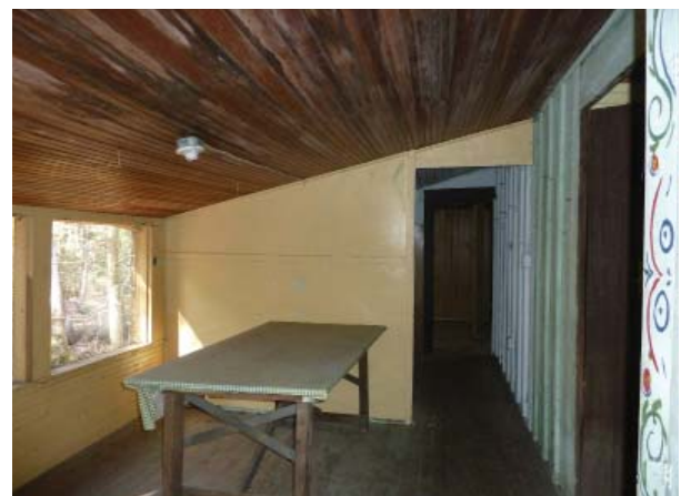
Figure 87. Dining Room (Room 107) looking north.
