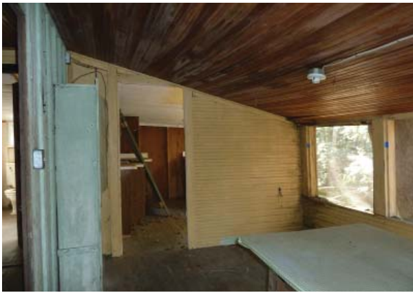
Figure 88. Dining Room (Room 107) looking south.
