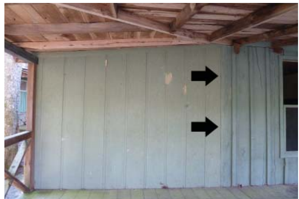
Figure 44. Seam in cladding of east elevation.
