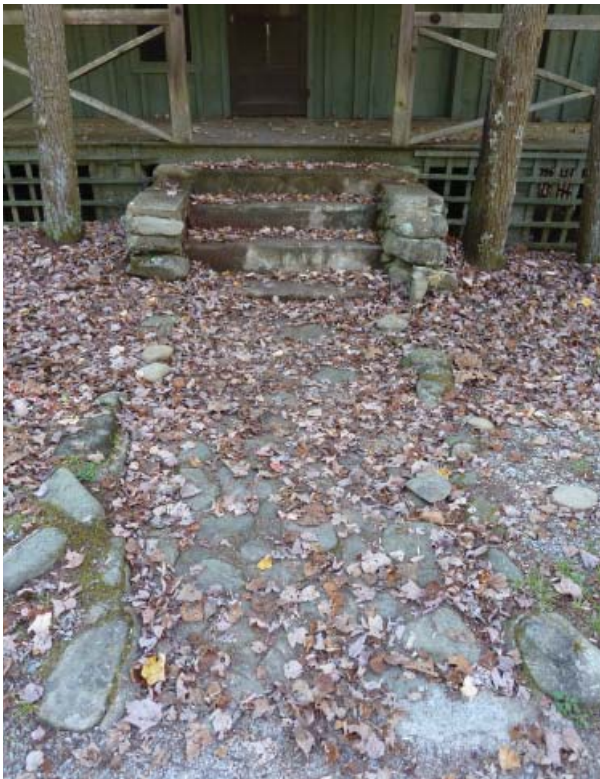
Figure 38. Front walkway and steps to Creekmore Cabin.
