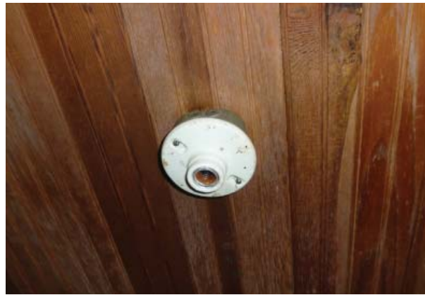
Figure 49. Typical ceramic lamp base mounted on ceiling.
