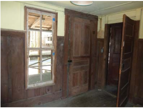
Figure 76. Southeast oblique of Northeast Bedroom (Room 103).
