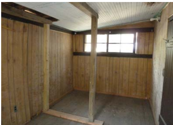
Figure 81. Northeast oblique of Northwest Bedroom (Room 105).
