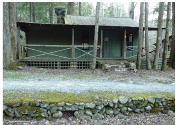
Figure 37. River stone retaining wall and gravel walkway in front of Creekmore Cabin.
