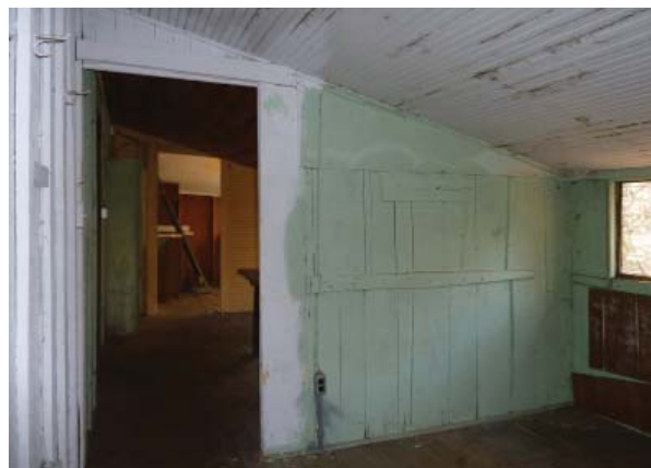
Figure 85. Southwest oblique of Storage Room (Room 106).
