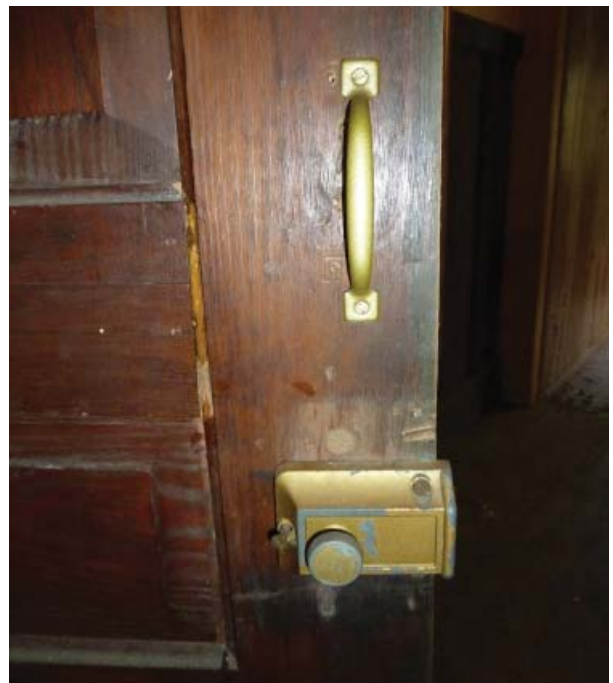
Figure 73. Hardware on the east exterior door.
