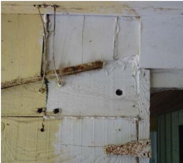
Figure 94. Ceramic tubes for early knob-and-tube wiring.
