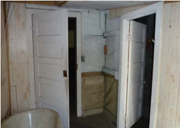
Figure 97. Northeast oblique of Bathroom (Room 109).
