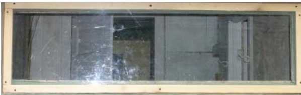
Figure 26b. A clear sheet of replacement glass was installed after the Van Gilder leaded window was stolen from the cabin in 2014. Interior features of the bathroom are visible through the glass in this image. (Oppermann, June 2014)
