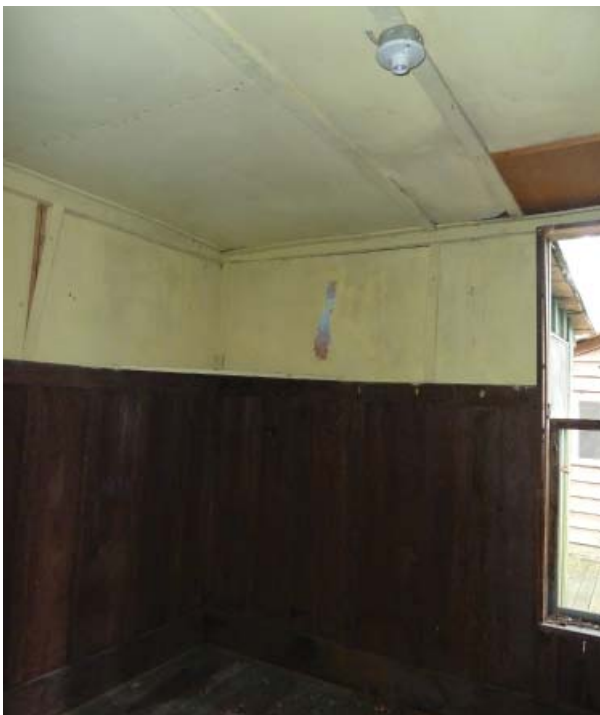
Figure 79. Northwest oblique of Middle Bedroom (Room 104).
