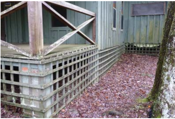
Figure 46. Lattice grid at foundation.
