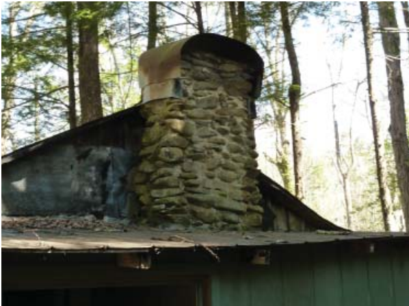
Figure 58. River stone chimney with tin cap.
