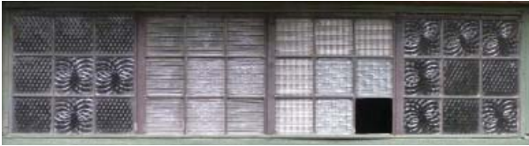
Figure 26a. Leaded glass window of clear patterned glass made for the cabin by owner Walter Van Gilder in the factory of his Van Gilder Glass Company. (Family collection)
