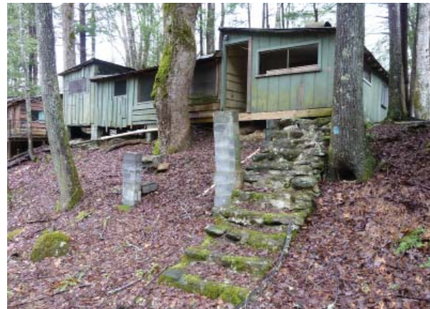
Figure 40. Southwest steps down to the backyard.
