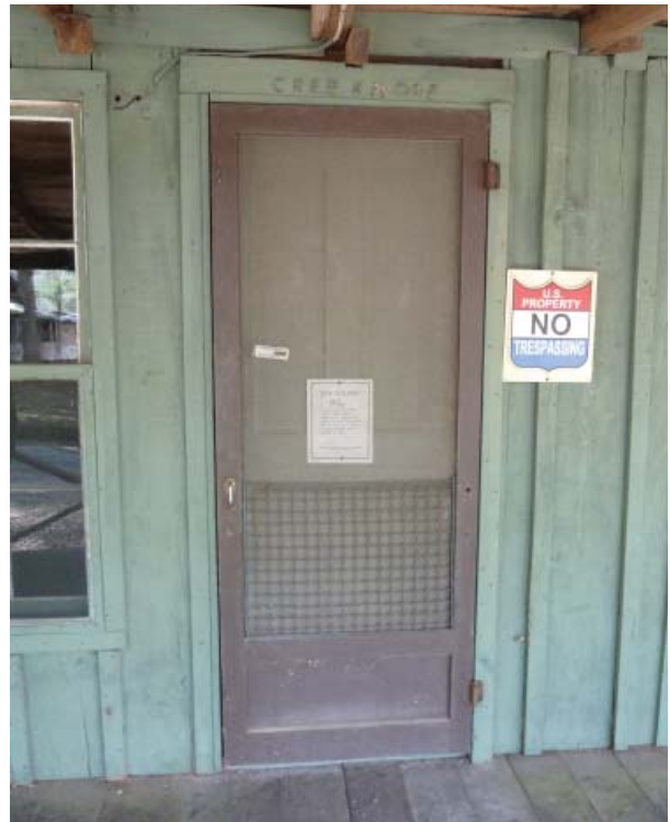
Figure 60. South doors of front elevation.
