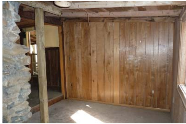
Figure 68. Living Room Extension (Room 101) looking northeast.
