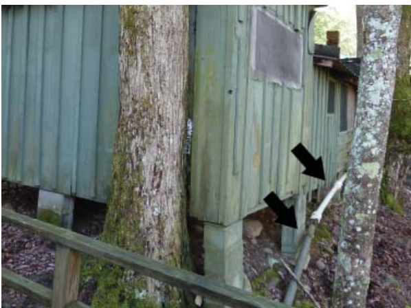
Figure 51. Water supply line that runs along the west elevation.
