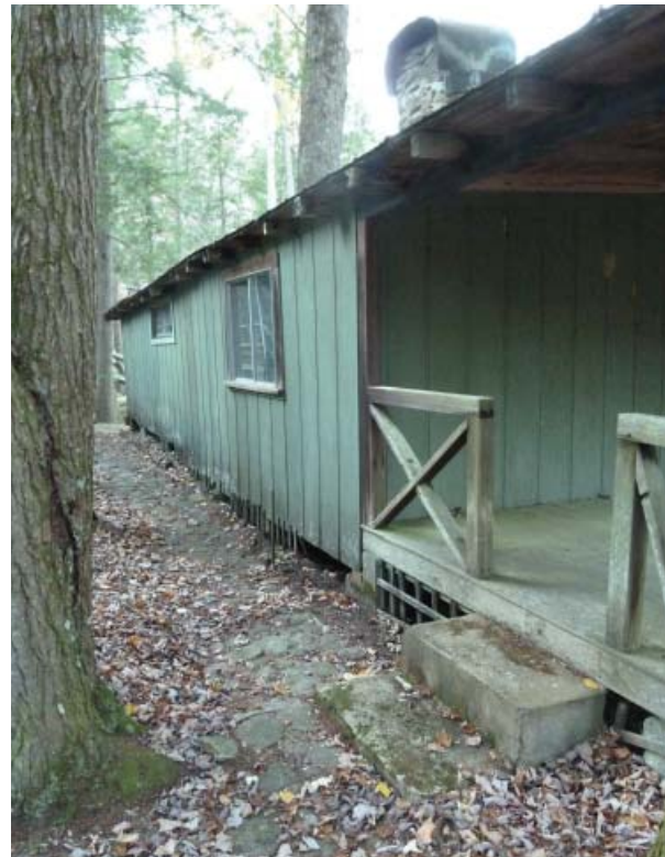
Figure 39. River stone walkway along south elevation and south porch steps.
