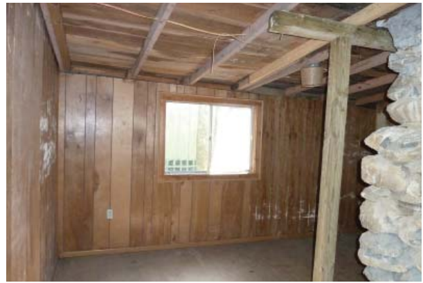
Figure 66. Living Room Extension (Room 101) looking south.
