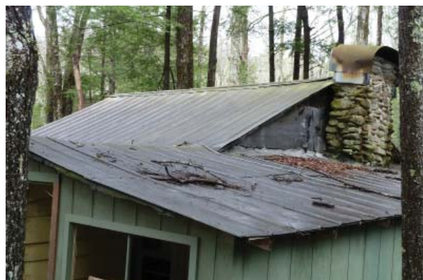
Figure 57. Metal roof of main block and south extension.
