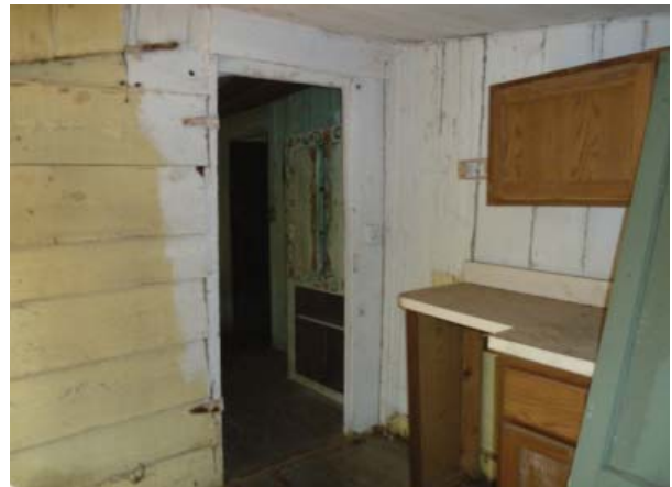
Figure 92. Northeast oblique of Kitchen (Room 108).
