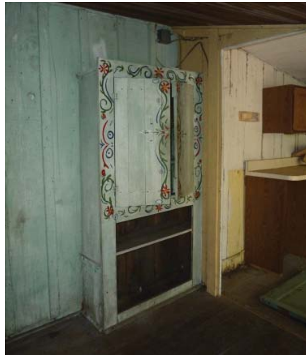
Figure 90. Cabinet in southeast corner of Dining Room (Room 107).
