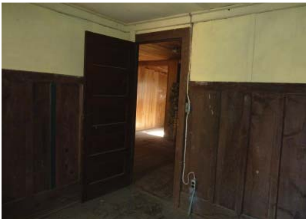
Figure 78. Southeast oblique of Middle Bedroom (Room 104).
