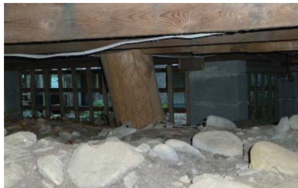
Figure 45. Typical unmilled foundation post and modern CMU pier.
