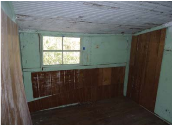
Figure 86. West elevation of Storage Room (Room 106).
