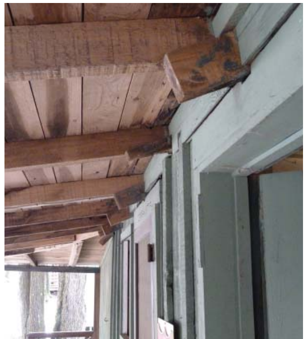
Figure 47. Front porch with overhanging roof rafters of the main block.
