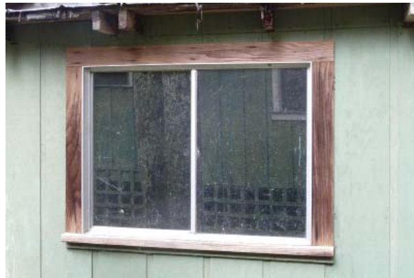
Figure 64. Modern aluminum window on the south elevation.
