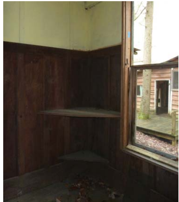
Figure 77. Wood shelves in the northwest corner of the Northeast Bedroom (Room 103).
