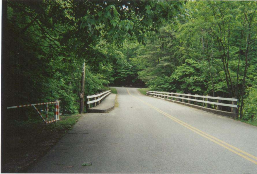
Figure 5. Elkmont Campground Road over Little River
