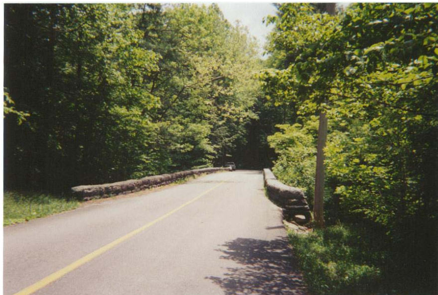
Figure 4. Elkmont Road over Little River
