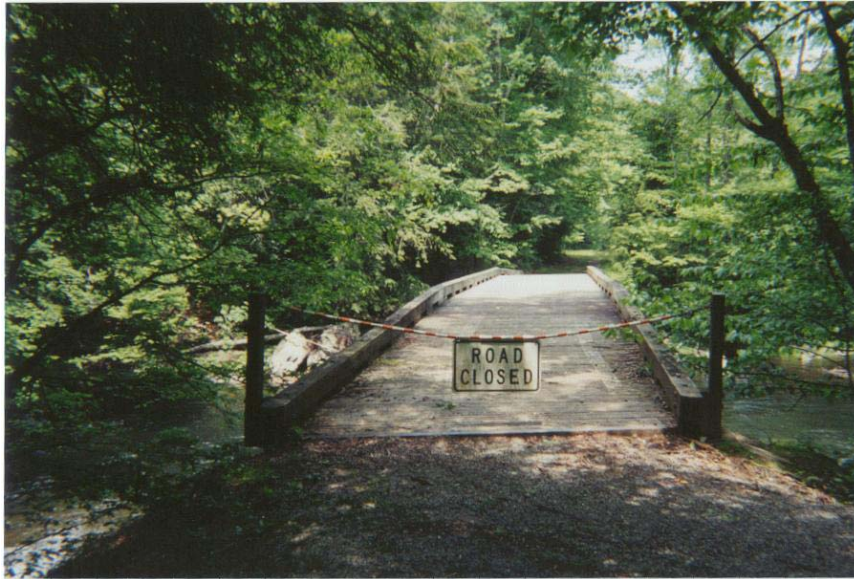
Figure 7. Bridge on Abandoned Road over Little River
