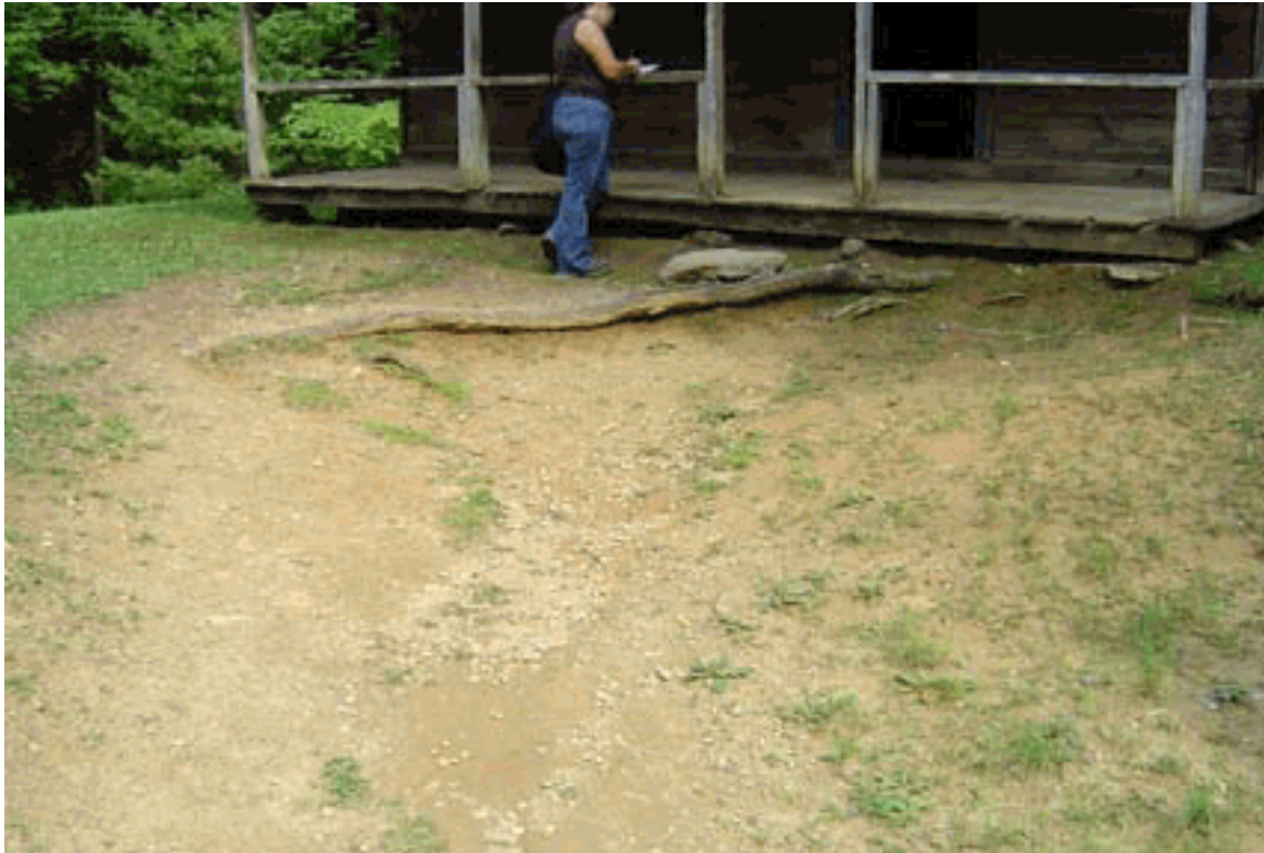
Visitor use is causing erosion along the pathway to the house, including portions of the house foundation (2006).
