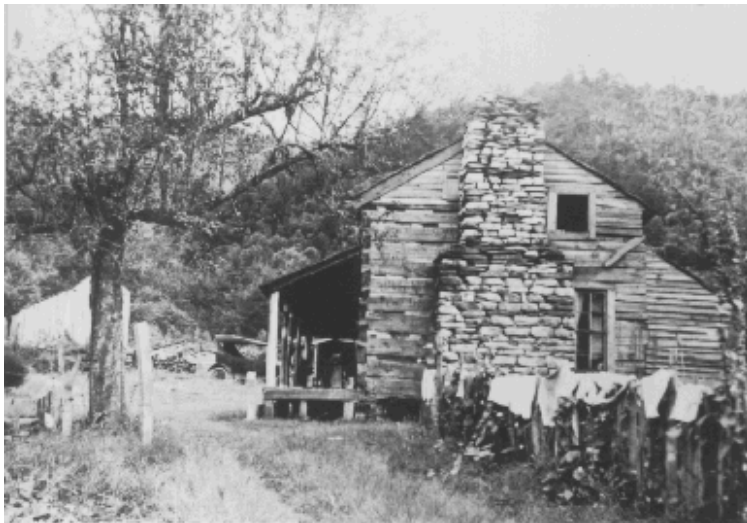
Figure 2. 1930s view of the John Oliver Homestead (from the south)
