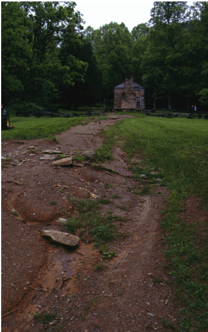
Eroded volunteer path, looking north (2000).
