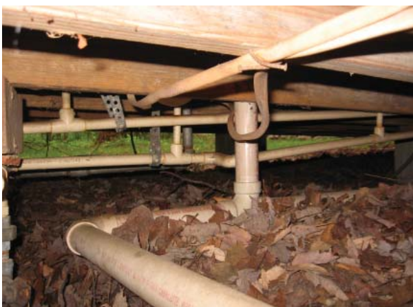
Figure 13, Floor structure and plumbing under Kitchen.
