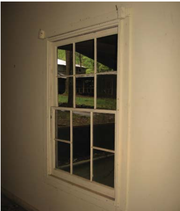
Figure 30, Double-hung window at west wall of Room 101.
