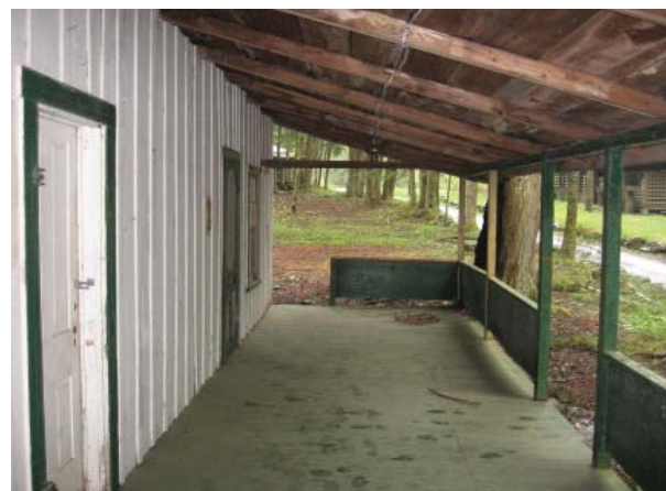
Figure 14, Front Porch, view toward south.
