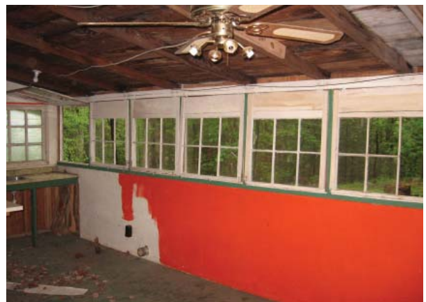
Figure 40, Kitchen, Room 103, view toward east wall.
