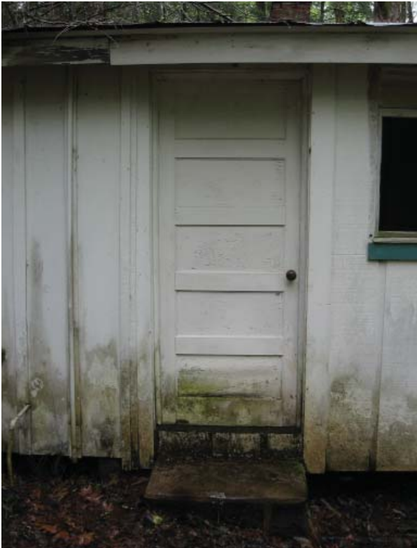
Figure 21 , Five-panel door to Room 103.
