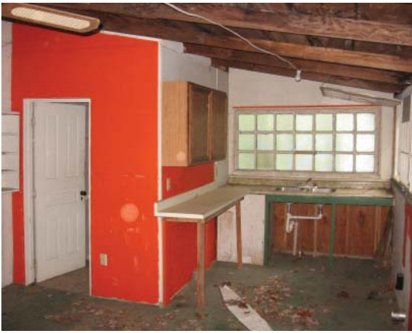
Figure 38, Kitchen, Room 103, view toward north.
