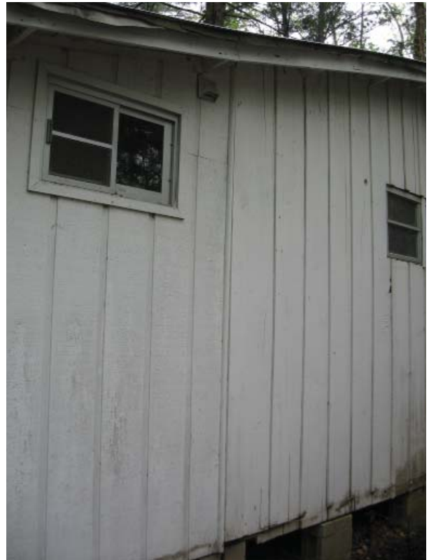
Figure 17, North wall of cabin at juncture of original vertical board siding and modern plywood siding.
