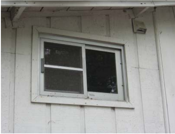
Figure 24 , Aluminum replacement window at north wall of bathroom, Room 103A.
