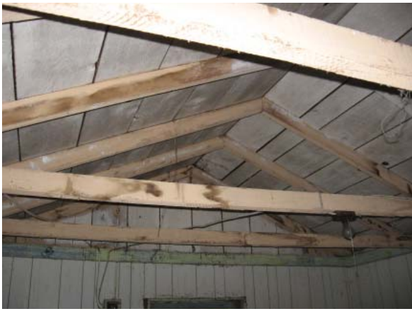
Figure 52, Exposed roof framing in Room 101.
