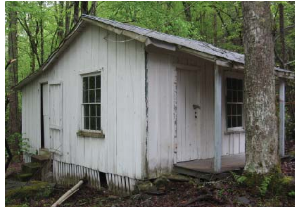
Figure 48 , Northwest oblique. Note use of vertical wood slat underpinning.
