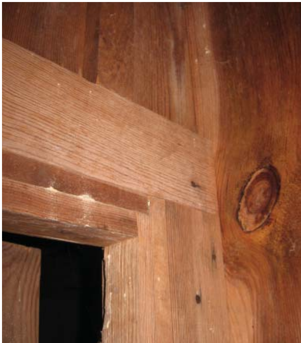
Figure 63 , Detail of casing at interior door.
