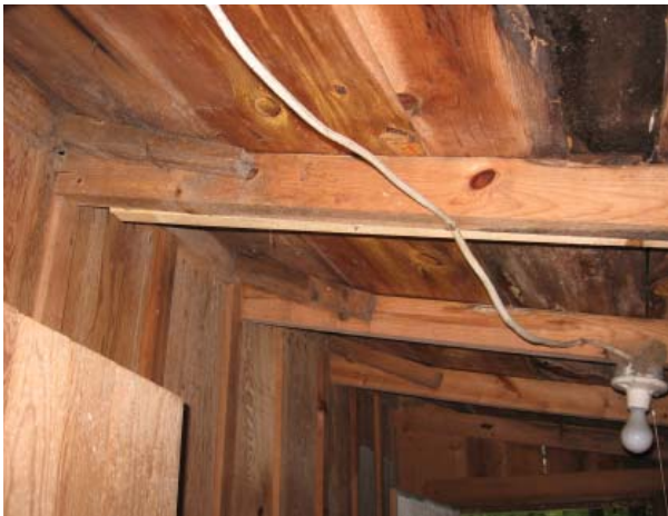
Figure 53, Exposed roof framing in Room 103, bedroom.
