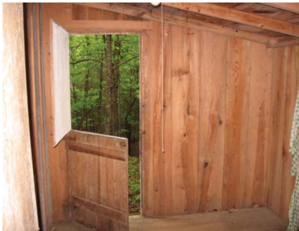
Figure 65, Bedroom, 103, view toward north.
