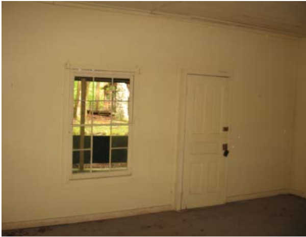
Figure 27, Room 101, view toward west wall.
