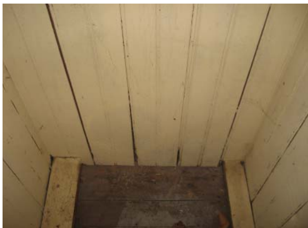
Figure 33, Closet 101A, view toward west. Note beaded board walls.
