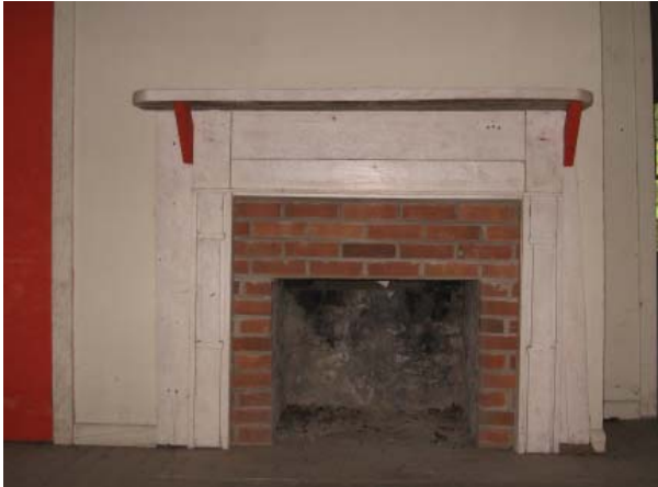
Figure 36, Fireplace at Room 102.
