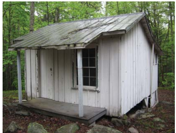
Figure 46 , Mayo Cabin Servants' Quarters, southwest oblique.
