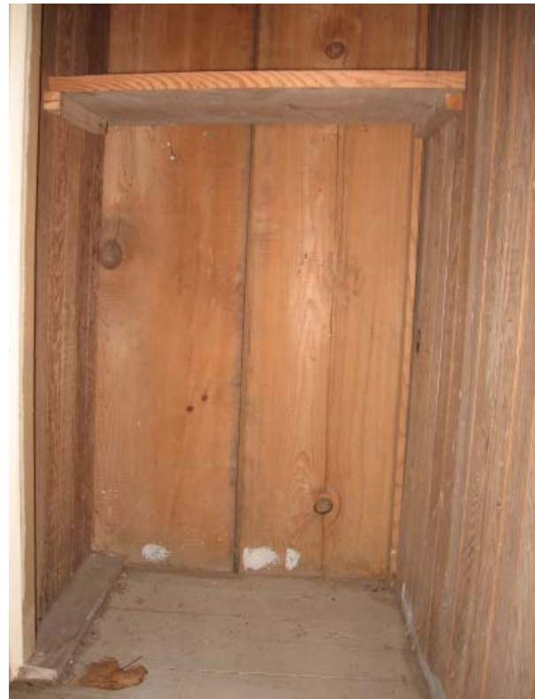
Figure 37, Closet 102A, view toward east. Note exposed vertical board wall.
