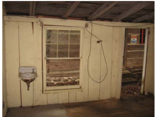
Figure 42, Room 104 view toward east wall.
