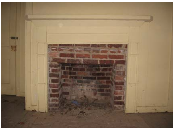
Figure 32, Fireplace at Room 101.
