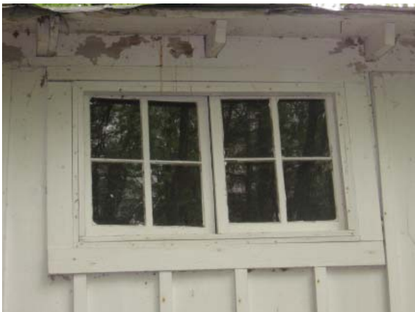
Figure 58, Paired casement windows at Room 103.
