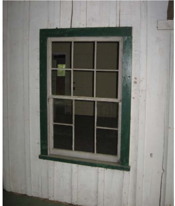
Figure 22 , Double-hung sash at Front Porch.
