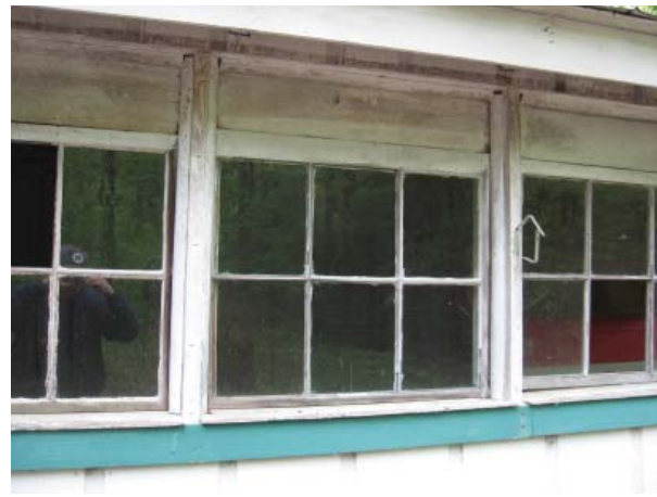
Figure 26 , Awning windows at east wall of Room 103.
