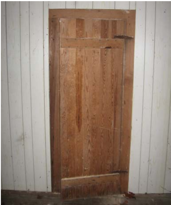
Figure 61, Door from Room 101 to Room 102.
