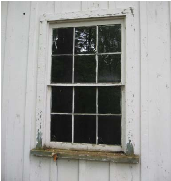
Figure 57, Double-hung window at north wall of Room 101.
