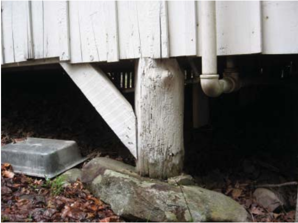
Figure 49 , Detail of locust pier bearing on rock at south wall.
