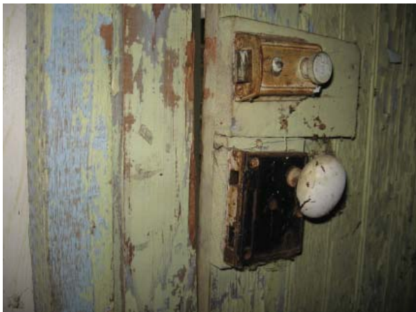
Figure 67 , Cast-iron rim lock with steel knobs at front entrance door.
