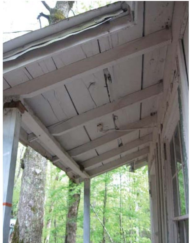
Figure 51 , Roof framing at Front Porch.
