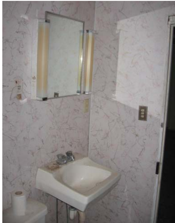
Figure 41, Bathroom, Room 103A, view toward southeast.
