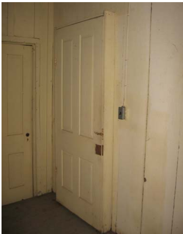
Figure 43, Room 104, door to Room 103.
