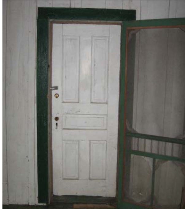
Figure 19 , Five-panel door with screen door at Front Porch to Room 101.
