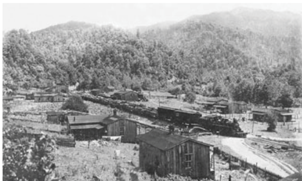
Figure 10 , Undated photograph of log train in Elkmont. (Little River Lumber & Railroad Museum)
