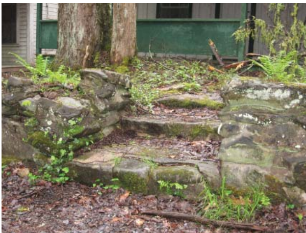
Figure 4, Stone steps leading from road to stone walk.
