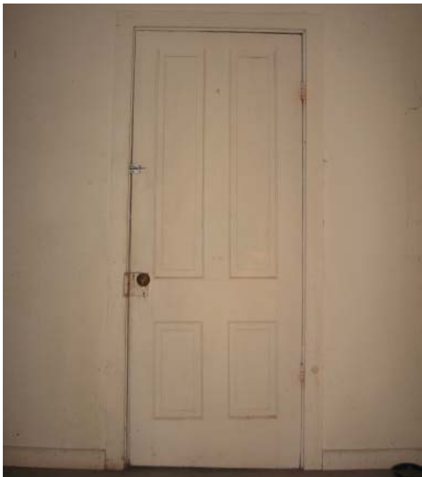
Figure 35, Room 102, door D9.
