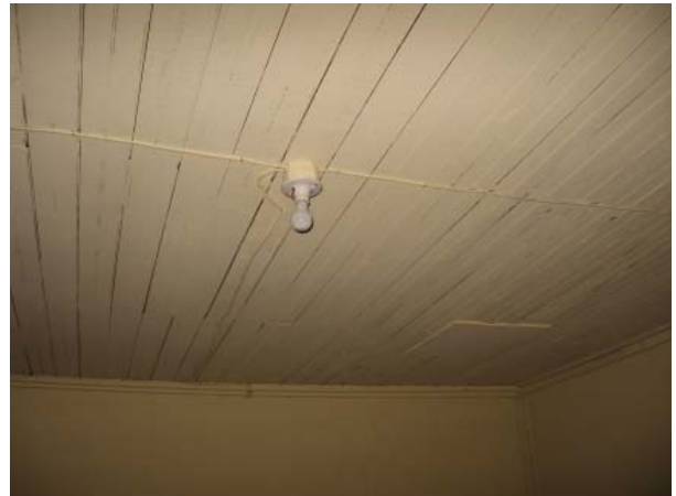
Figure 31, Beaded board ceiling at Room 101.
