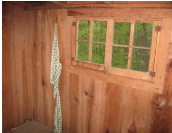
Figure 66, Bedroom, 103, view toward east.
