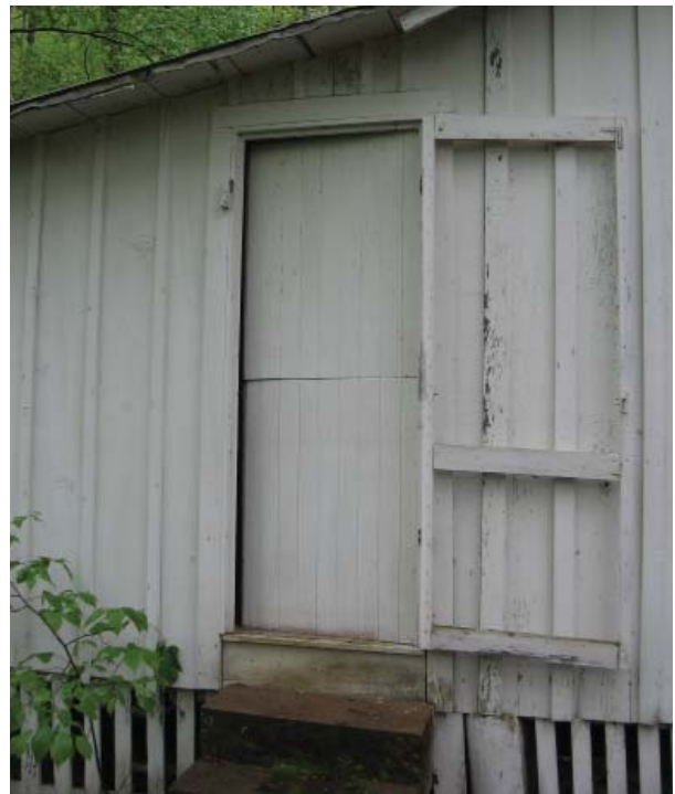
Figure 56, Dutch door opening into Room 103.
