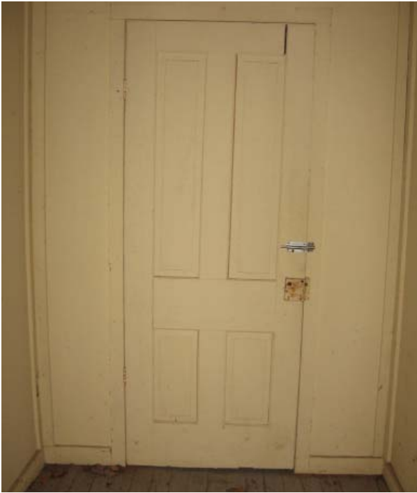
Figure 29, Room 101, door leading to Room 102.
