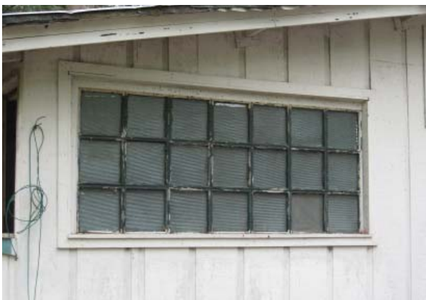
Figure 25 , Fixed sash window at north wall of Kitchen.
