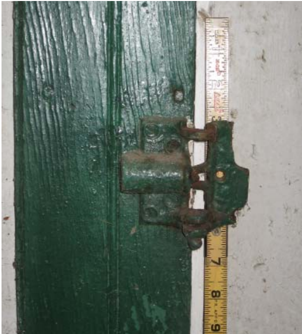
Figure 18 , Beaded board door casing at door to Room 102. Note patented cast-iron spring hinge.
