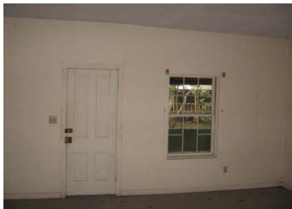
Figure 34, Room 102, view toward west wall.
