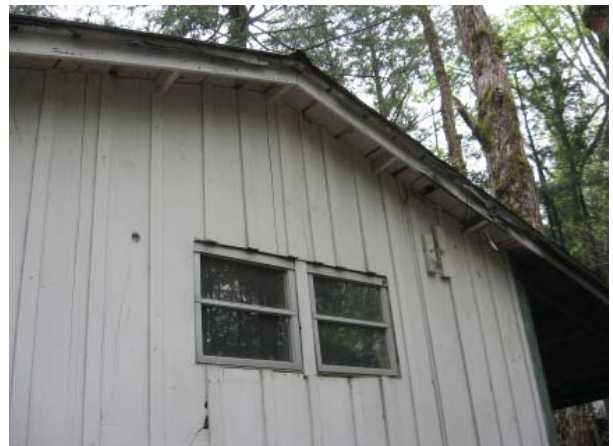
Figure 23 , Aluminum replacement windows at north wall of Room 102.
