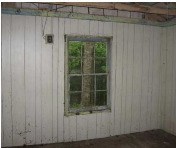
Figure 59, Room 101, view toward north.
