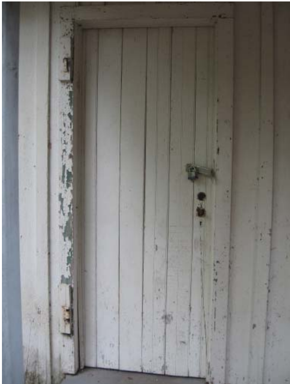
Figure 55, Front door from porch into Room 101.
