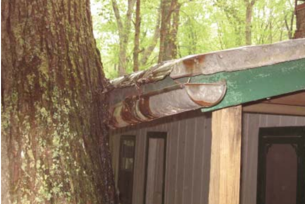
Figure 15, Half-round gutter section at south end of Front Porch.
