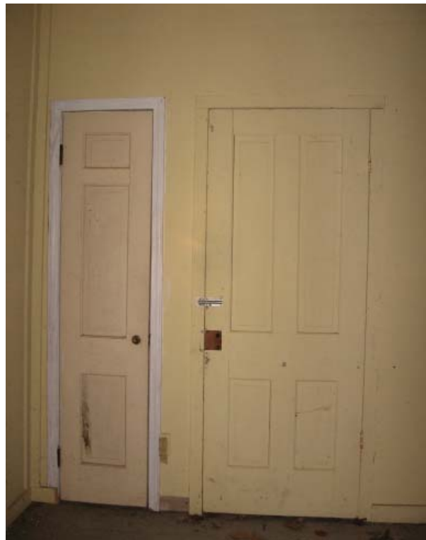
Figure 28, Room 101, doors leading to Room 103 (left) and 104 (right).
