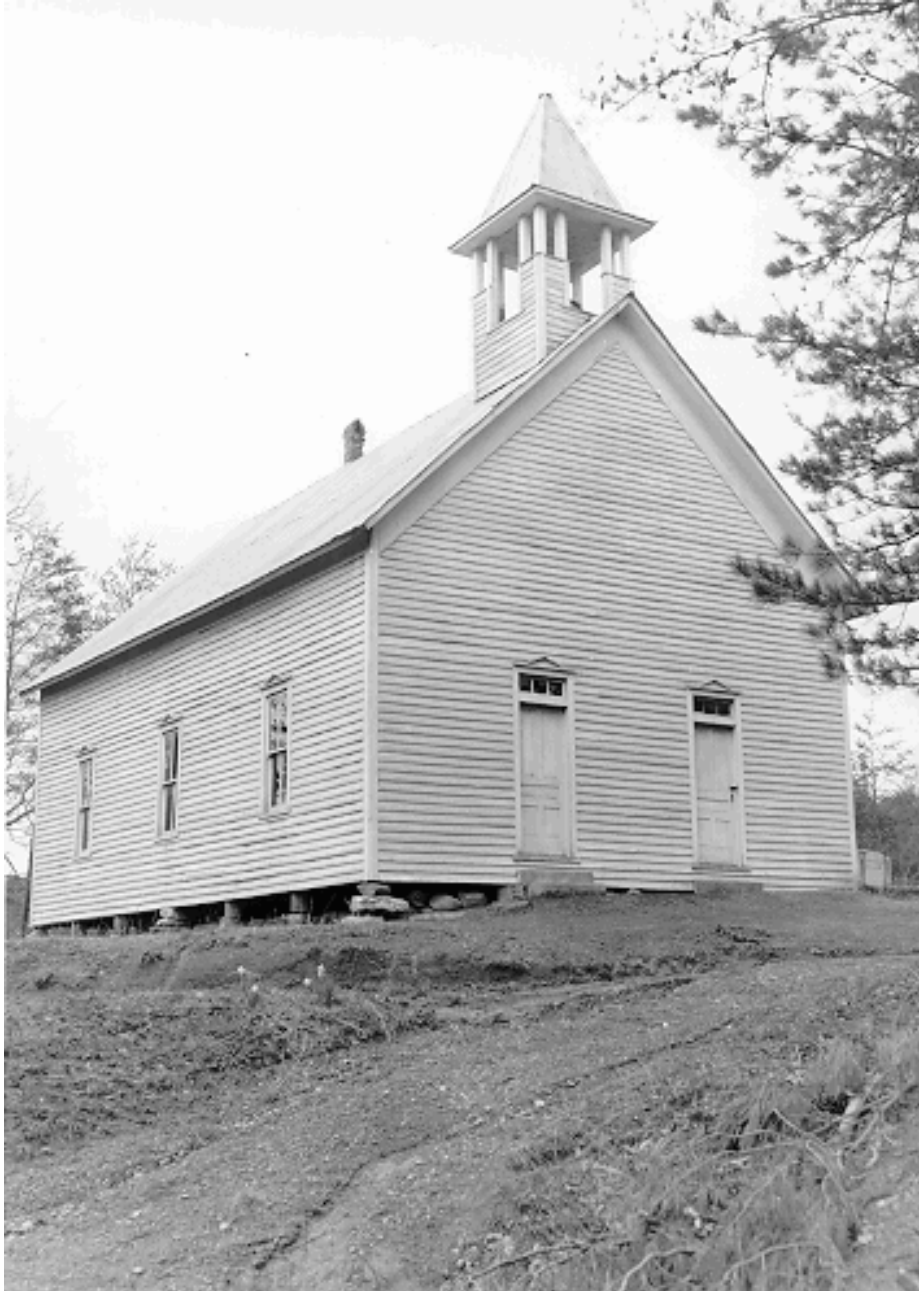
Figure 1. 1953 view of Cades Cove Methodist Church
