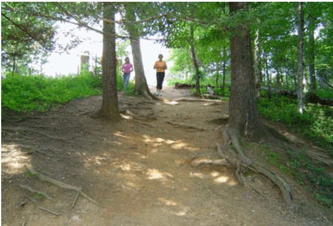
Volunteer pathway from parking lot to church. Note the significant level of erosion and exposed roots (2006).
