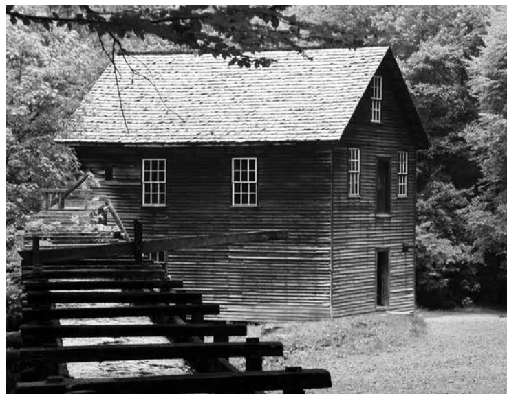
Mingus Mill was built in 1886 and is still grinding corn on its original stones. A turbine and the waters of Mingus Creek provide the power.
