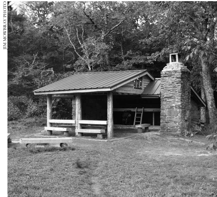
Primitive backcountry shelters like this one at Double Springs Gap are located along the Appalachian Trail and near the summit of Mt. Le Conte. Reservations are required for all campers in the backcountry.
