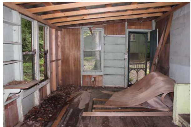
Figure 51: Room 109 looking south toward exterior door.
