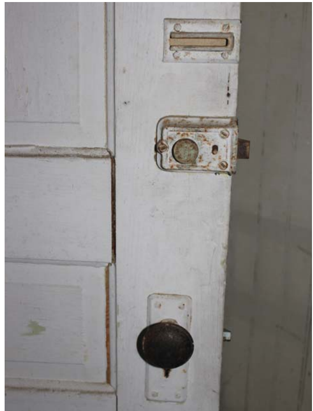
Figure 29: Front entrance door hardware.
