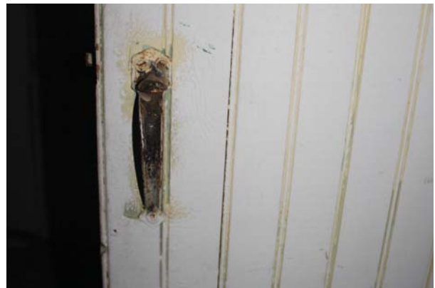
Figure 34: Room 102 door hardware, hallway side.
