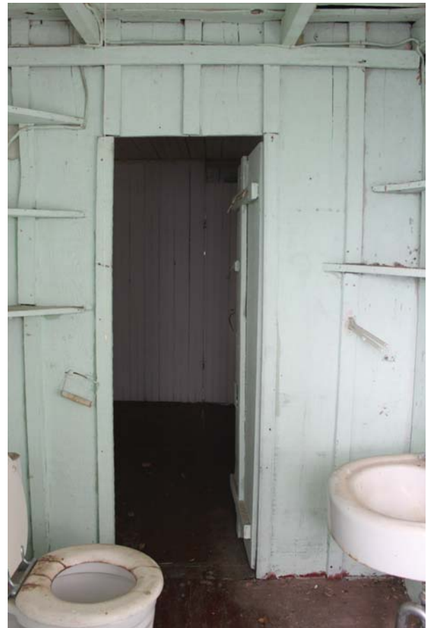
Figure 43: Room 105 looking north.
