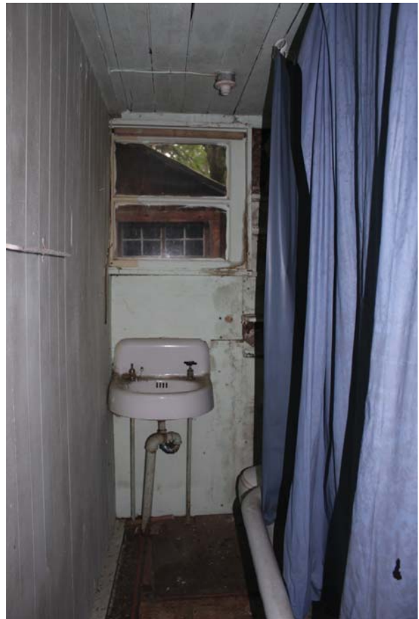
Figure 39: Room 104 bathroom, note window shared with Room 103.
