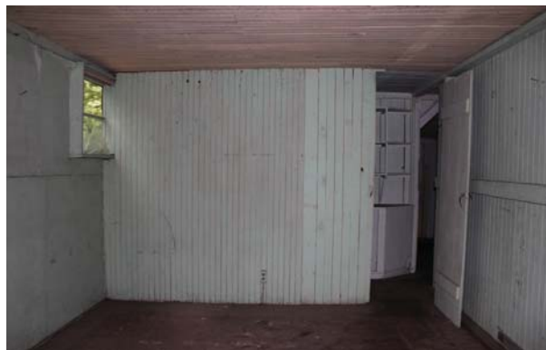
Figure 38: Room 103 looking east.
