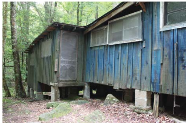
Figure 19: Rear entrance stoop at north side elevation.
