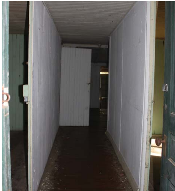
Figure 28: Room 101 - hallway - looking from front entrance door toward rear hallway.
