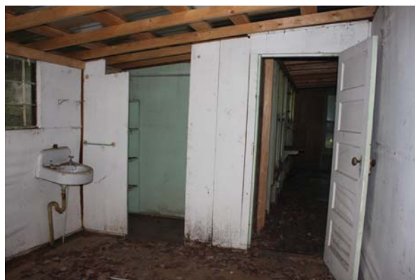
Figure 56: Room 111 looking toward closet and doorway.
