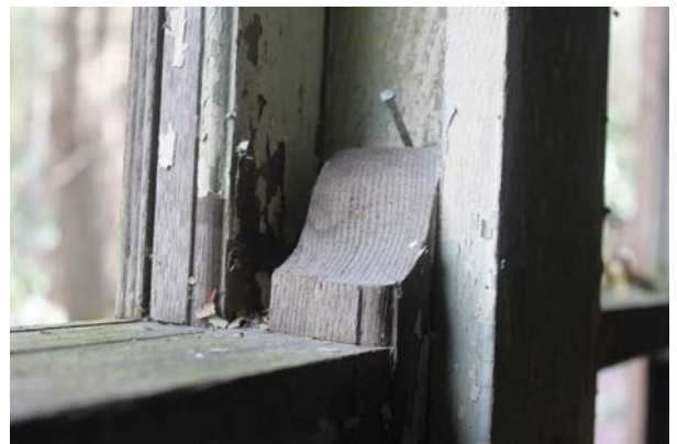
Figure 26: Decorative wood lug on double-hung windows in Room 109.
