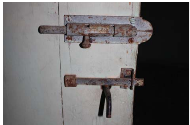
Figure 35: Room 102 door hardware, Room 102 side.
