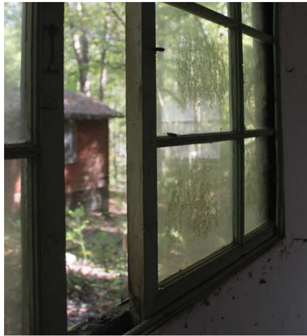
Figure 27: Sliding windows with wall pockets in Room 111.
