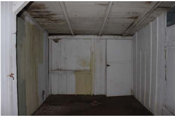
Figure 45: Room 107 looking east toward Room 109.
