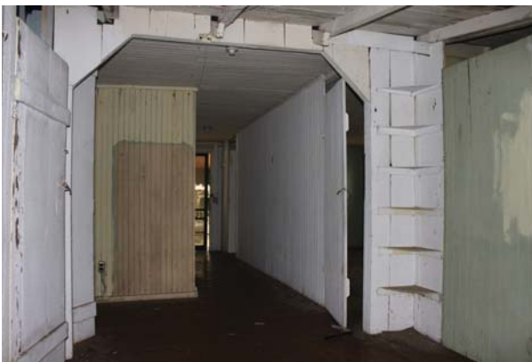
Figure 46: Room 107 looking west toward the hallway.
