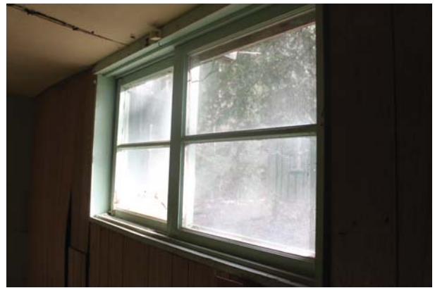
Figure 24: Sliding windows in Room 102.
