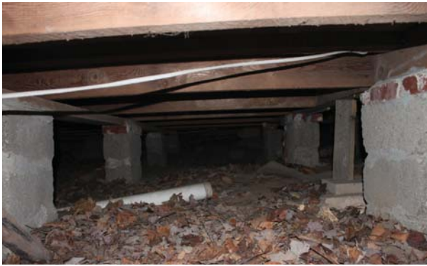
Figure 13: Foundation CMU piers and floor framing under Room 103.
