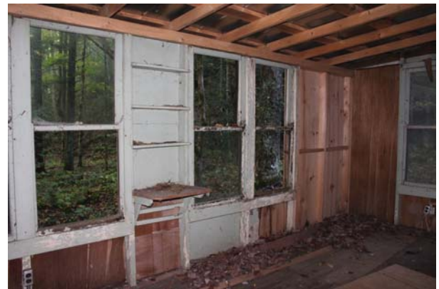
Figure 25: Double-hung windows in Room 109.
