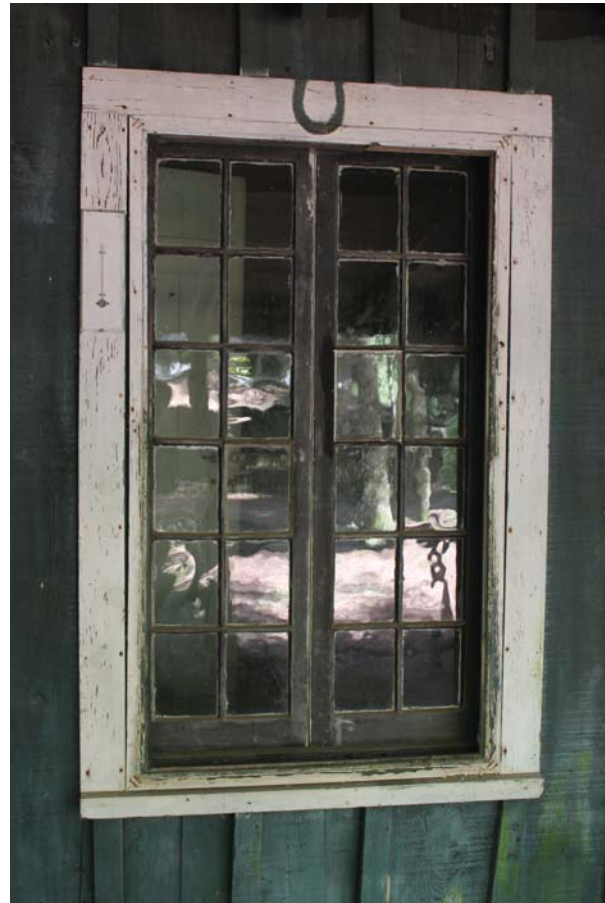
Figure 23: Casement window on west front elevation.
