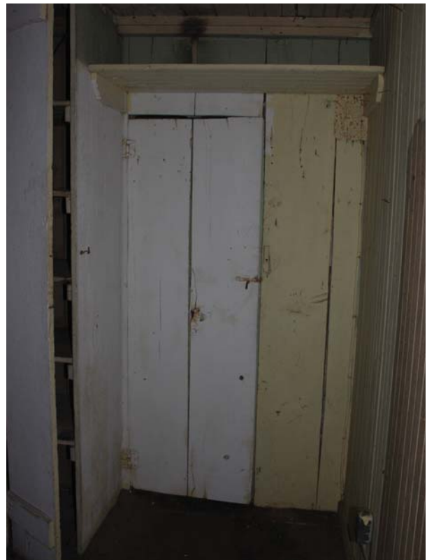
Figure 30: Room 101a - rear hallway - looking toward Room 105.
