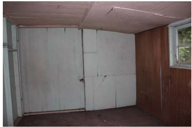
Figure 33: Room 102 looking east.
