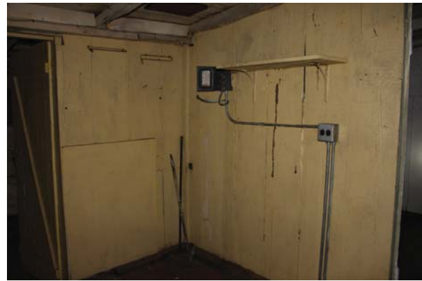
Figure 49: Room 108 location of hot water heater.
