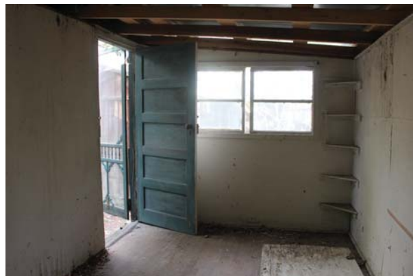
Figure 53: North end of Room 110 with exterior entrance door.
