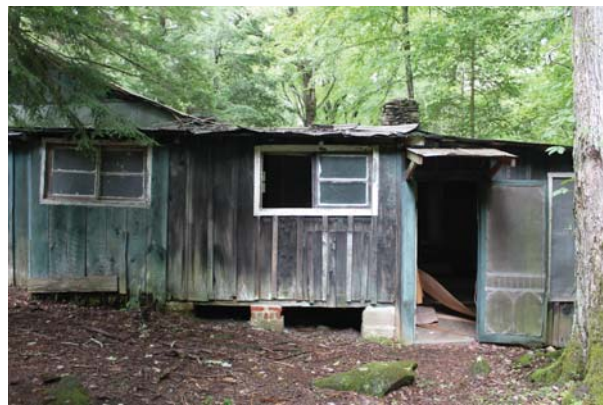
Figure 18: Rear entrance stoop on south side elevation.
