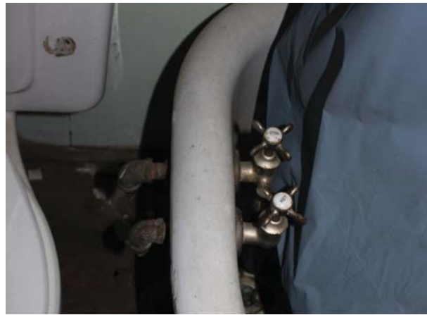
Figure 40: Room 104 tub faucets.
