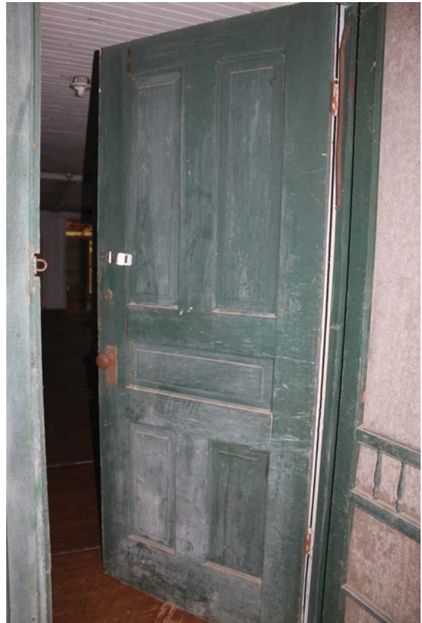
Figure 21: Front entrance door.
