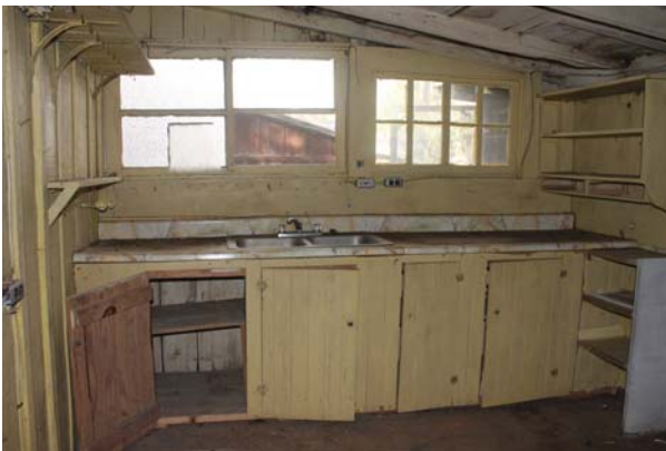
Figure 47: Room 108 looking north toward the cabinets and sink.
