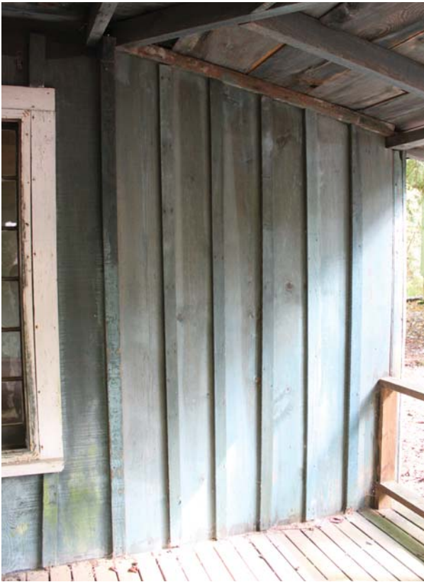
Figure 15: Front porch roof framing.
