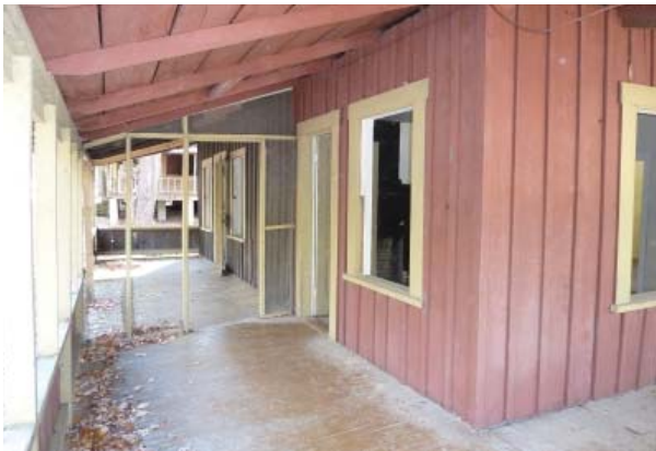
Figure 48. Front porch with remnants of screened panels.
