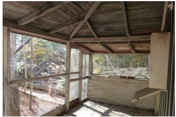
Figure 38. Roof framing at southwest porch.
