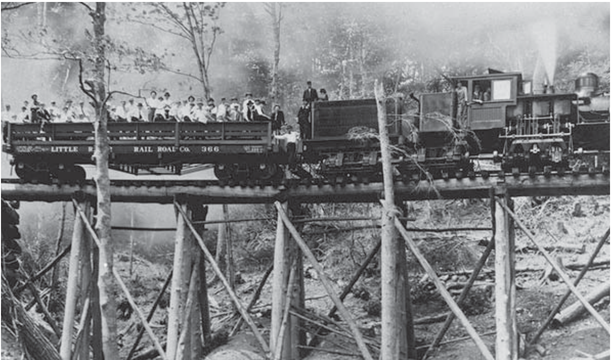
Figure 8. Little River Railroad Company observation car on wood trestle, undated photograph. (Little River Railroad and Lumber Company Museum)
