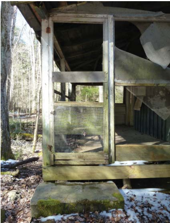
Figure 50. East elevation of south porch.
