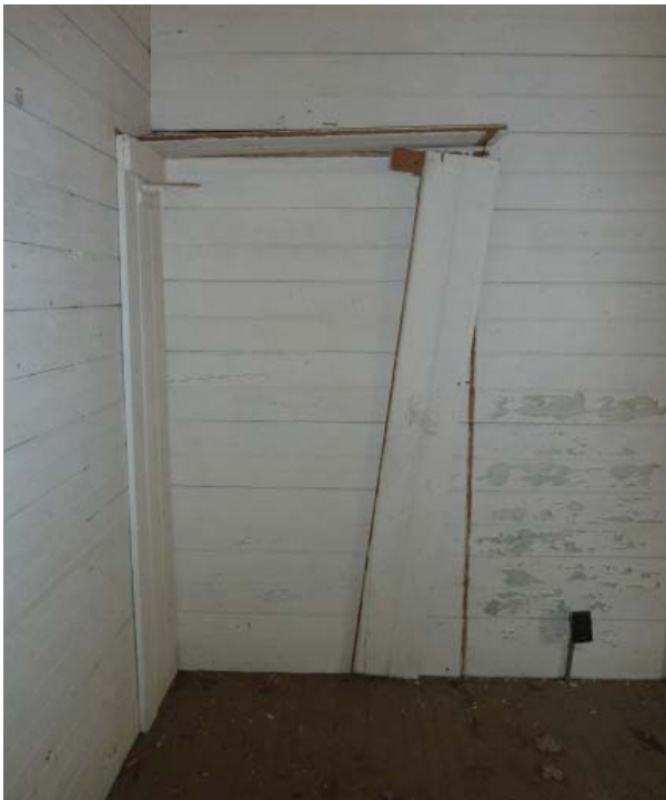
Figure 100. Closet on east wall of Middle Bedroom (Room 108).
