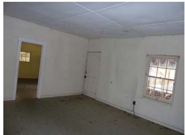
Figure 70. Northwest oblique of Northeast Living Room (Room 102).
