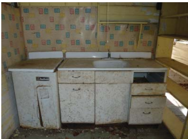
Figure 43. Sink in Kitchen (Room 106).
