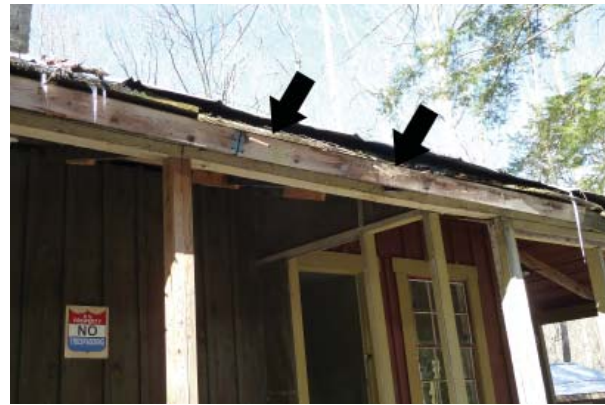
Figure 56. Supports for gutter at front porch.
