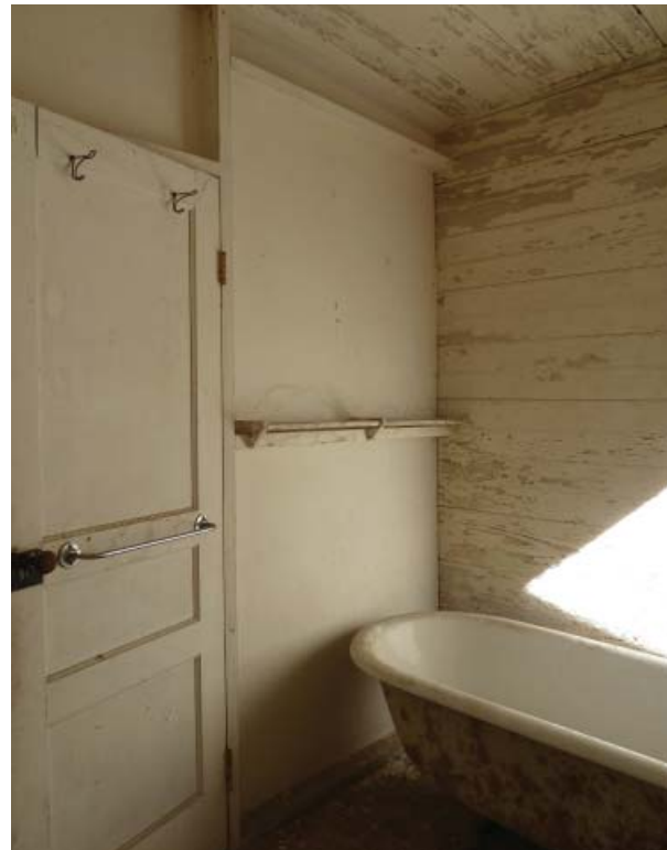
Figure 96. Northeast oblique of South Bathroom (Room 107b).
