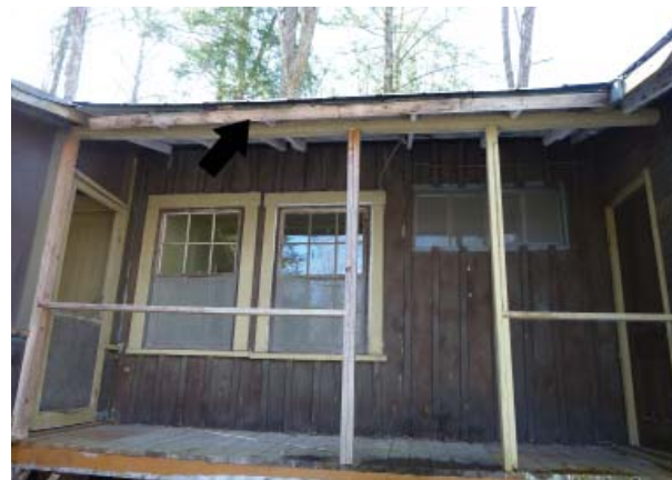
Figure 57. Supports for gutter at north porch.
