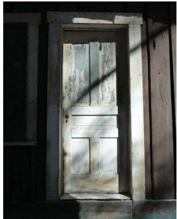
Figure 60. Five-panel door at south elevation.
