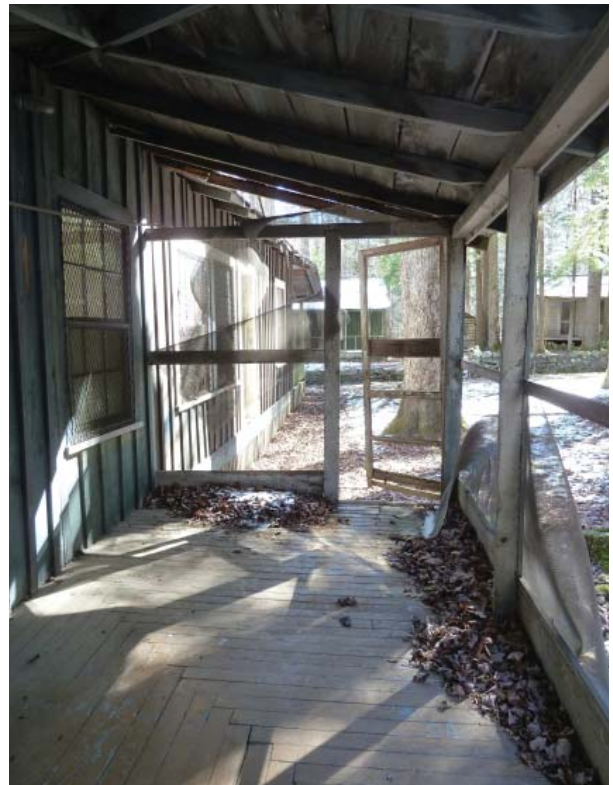
Figure 52. South porch looking east.
