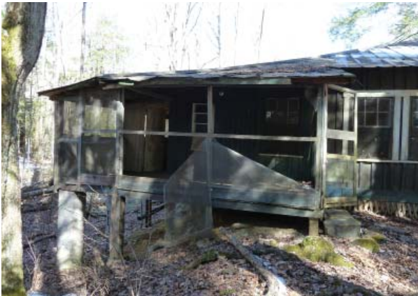
Figure 51. Southeast oblique of south porch.
