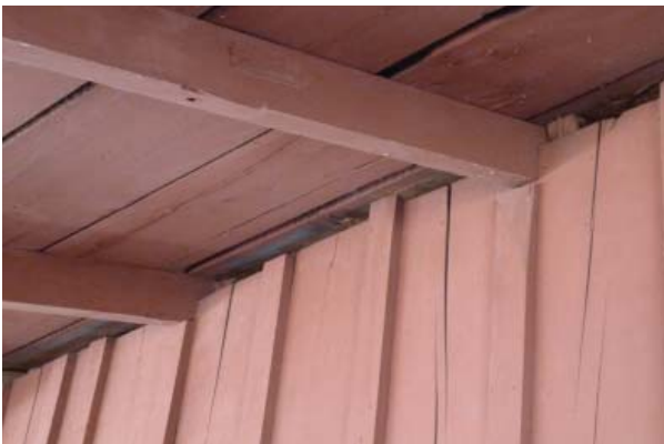
Figure 37. Front porch roof rafters are integrated into main block roof framing.
