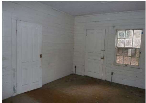
Figure 98. Southeast oblique of Middle Bedroom (Room 108).
