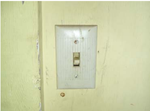
Figure 92. Light switch with plastic Bakelite plate.
