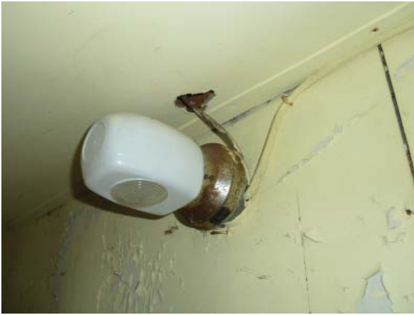
Figure 82. A 1950s-era light fixture mounted over the sink.
