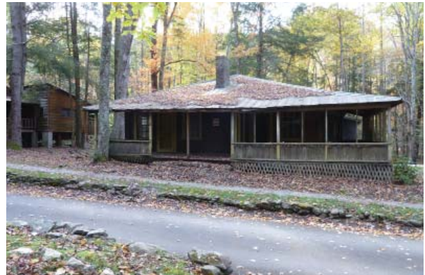
Figure 27. Front elevation of Smith Cabin from across Daisy Town Road.
