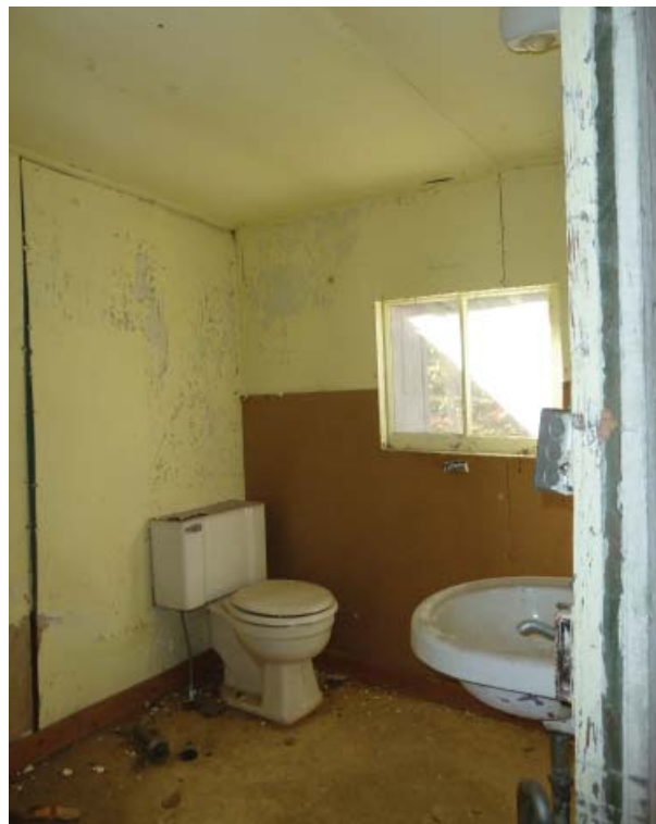
Figure 81. Southwest oblique of West Bathroom (Room 105).
