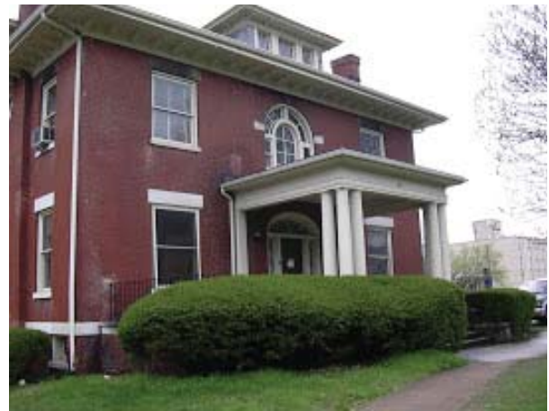
Figure 23. The Keller House before demolition. (Architectural salvage photographs, www.moretoknoxville.com/events/daily/2013/08/31/category:13 )
