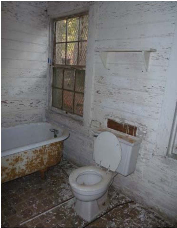
Figure 94. Southeast oblique of South Bathroom (Room 107b).
