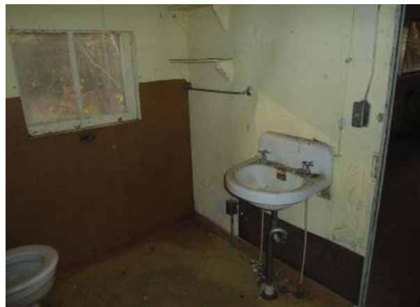
Figure 80. Northwest oblique of West Bathroom (Room 105).
