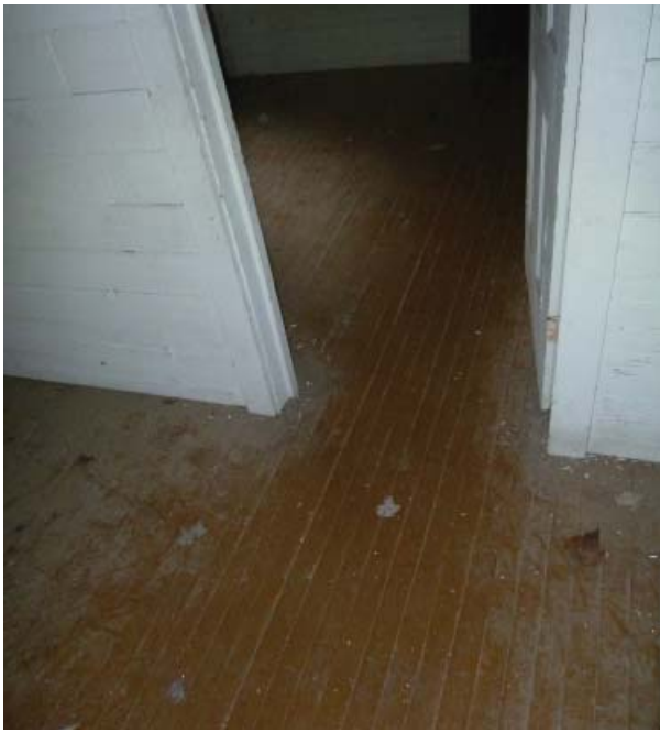
Figure 66. Flooring is continuous into Middle Bedroom (Room 108).
