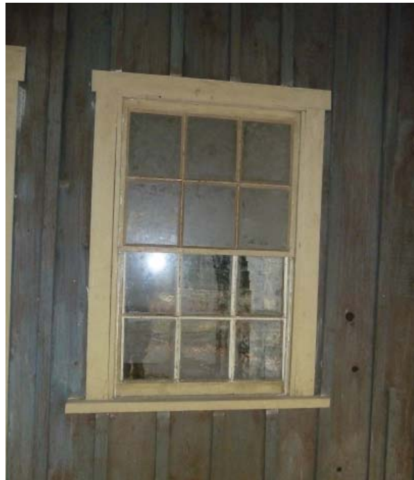
Figure 61. Typical six-over-six-light double-hung window.
