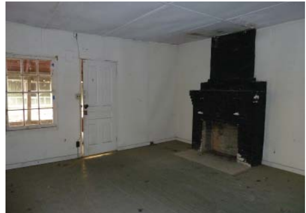
Figure 69. Southeast oblique of Northeast Living Room (Room 102).
