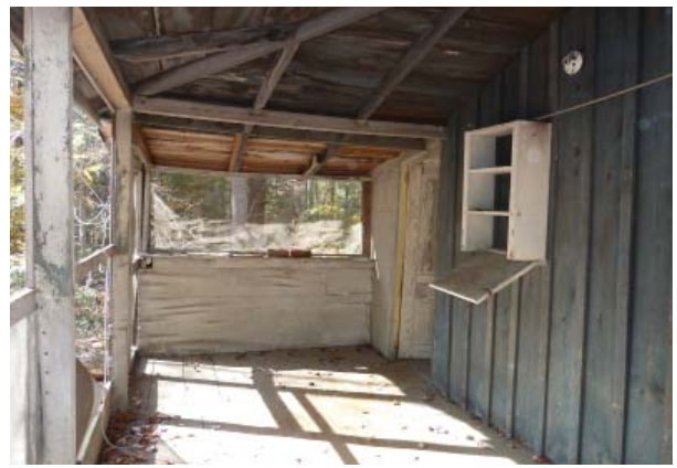
Figure 53. South porch looking west.
