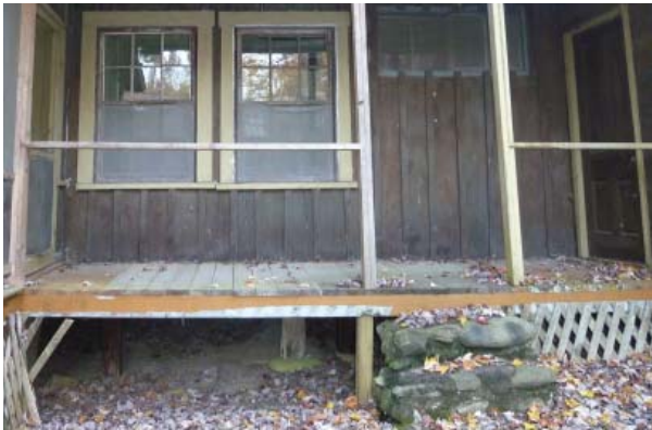
Figure 30. River stone steps at north porch.
