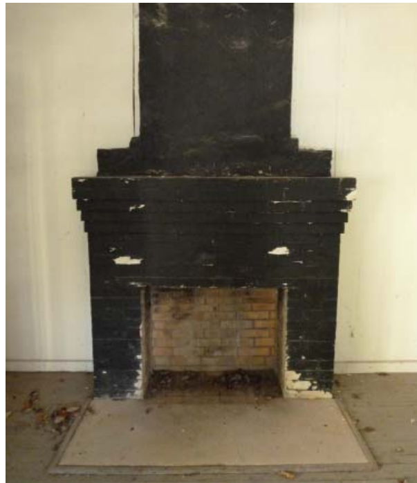
Figure 72. Fireplace and exposed chimney on south elevation.
