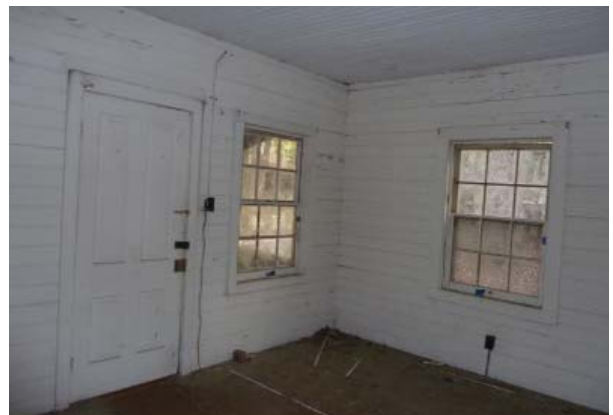
Figure 65. Southeast oblique of Southeast Primary Bedroom (Room 101).
