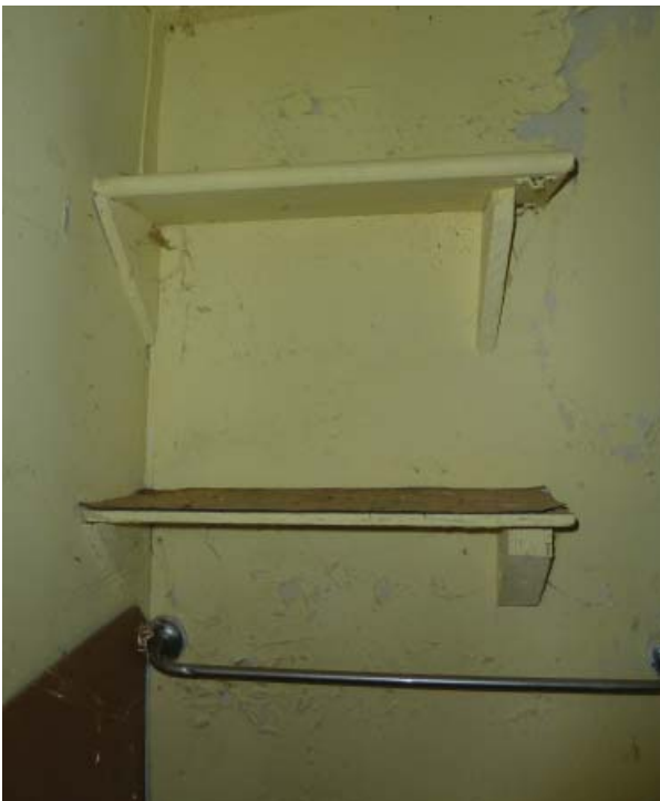
Figure 83. Wood shelves and chrome towel rack on the north wall.
