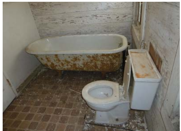
Figure 45. Toilet and tub in South Bathroom (Room 107b).
