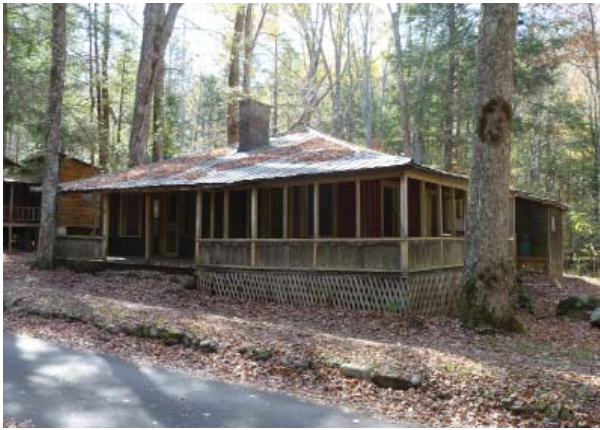
Figure 47. Northeast oblique of wraparound porch.
