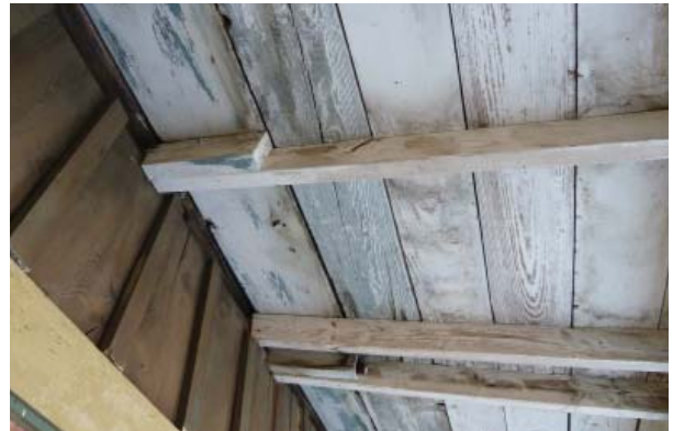
Figure 39. Roof framing of modern north porch.
