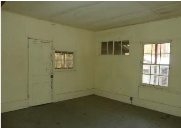
Figure 73. Northwest oblique of Northwest or Back Room (Room 103).
