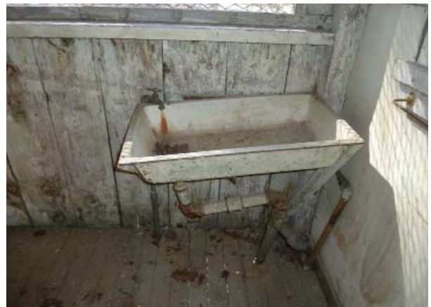
Figure 46. Sink in Enclosed Porch (Room 104).
