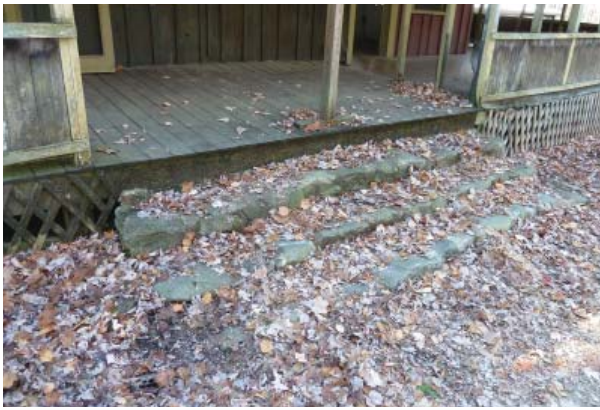
Figure 29. Fieldstone steps at front porch.
