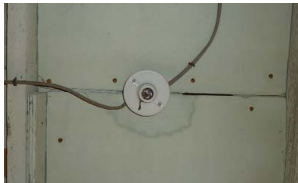
Figure 42. Typical ceramic lamp base mounted on ceiling.
