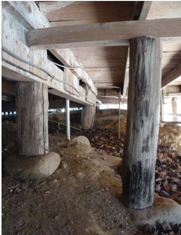
Figure 35. Unmilled posts of the main cabin block.
