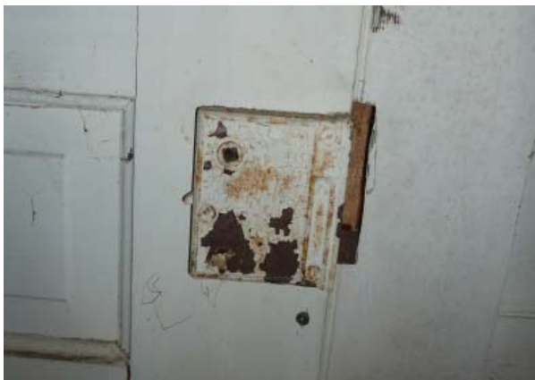
Figure 63. Typical door rimlock.
