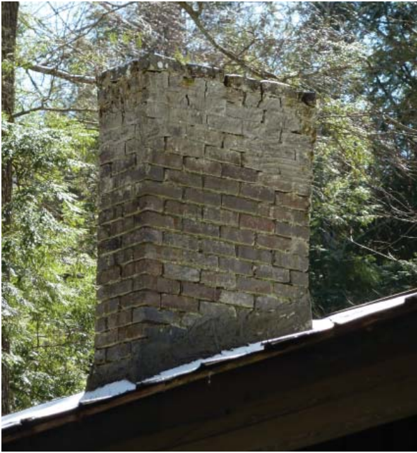
Figure 58. Brick chimney near east side of cabin.
