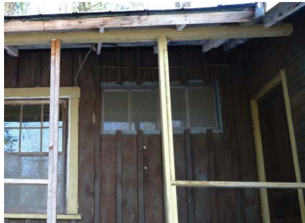
Figure 62. Pair of two-light sash on the north elevation that slide horizontally.
