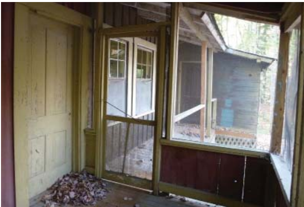
Figure 55. Screened door between wraparound porch and north porch.
