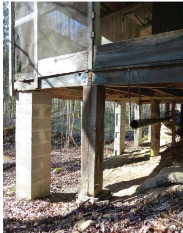
Figure 36. Square posts and CMU piers of the additions.
