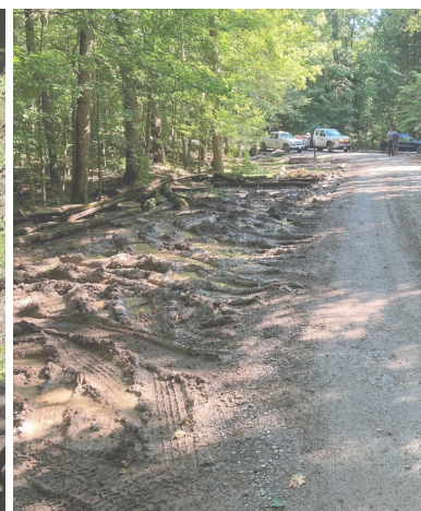
Muddy, rutted area along Big Creek Road.
