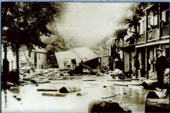
Flood damage on Shenandoah Street, 1889.
