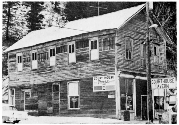
Photo: Arthur Hart, Idaho State Historical Society, 1978. Courtesy of the National Register of Historic Places.
