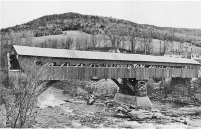
Photo: Hugh H. Henry, Vermont Division of Historic Sites. Courtesy of the National Register of Historic Places.
