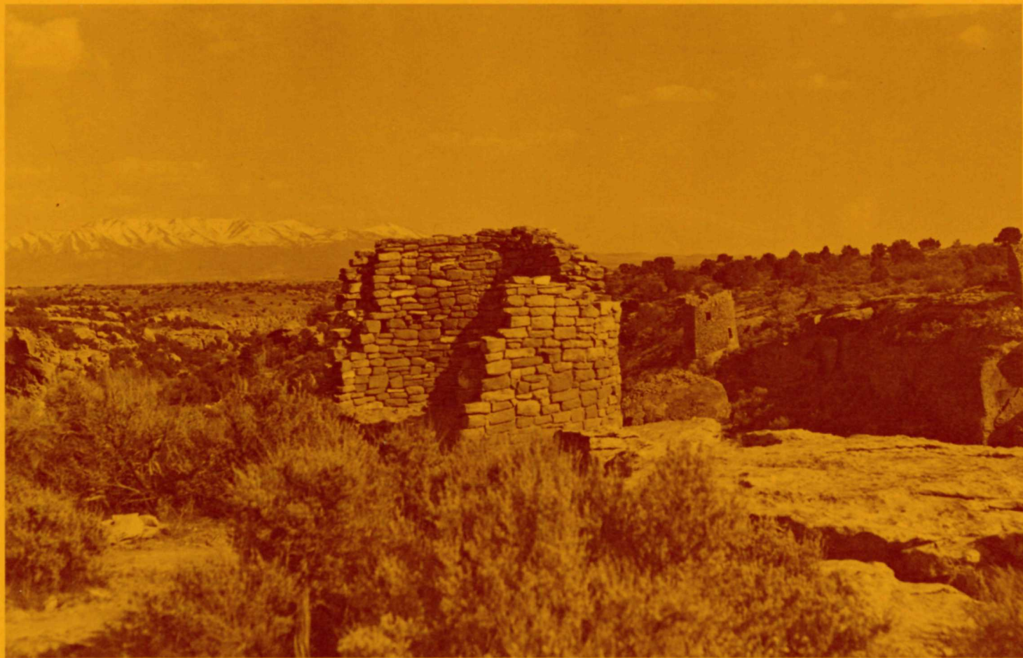
Tower at Tower Point
