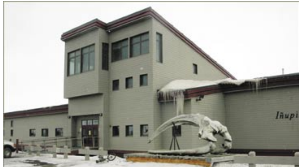
Exterior view of Iñupiat Heritage Center. NPS photograph
