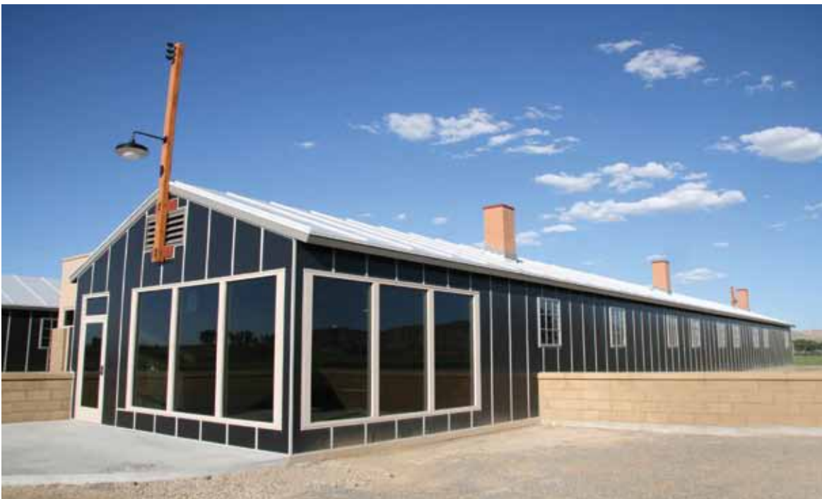
Side view of one of the Interpretive Learning Center buildings, the design of which is based on the Heart Mountain barracks. Photo courtesy: Heart Mountain, Wyoming Foundation.
