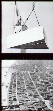
A derrick lifts a triangular section into place.
