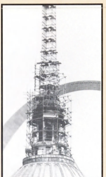
Courthouse in scaffolding
