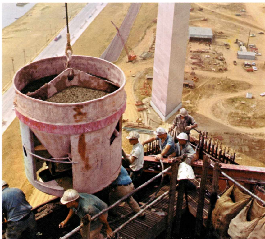
Concrete being poured to fill the void between inner and outer skins.
