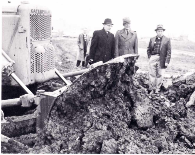
Excavation beginning for footings for 630-foot Gateway Arch.
