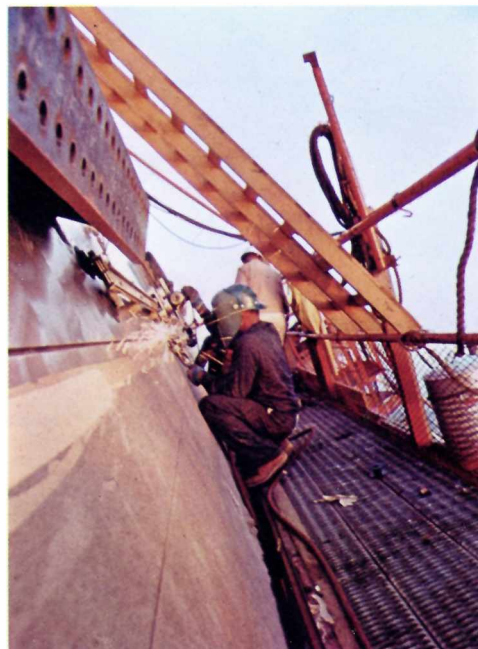
Welding stainless steel sections together.
