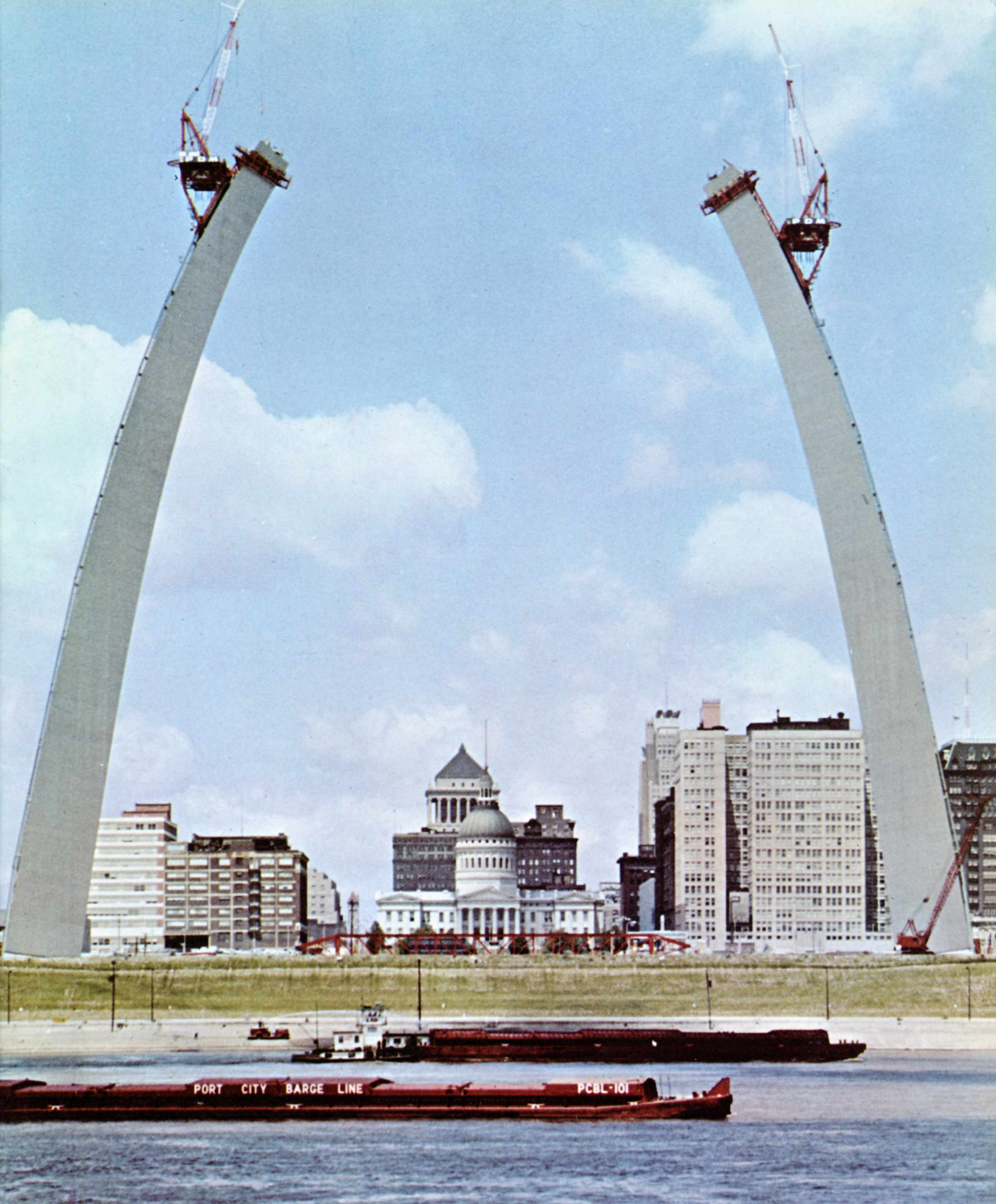
80-ton creeper derricks which lifted the temporary strut shown on the ground.
