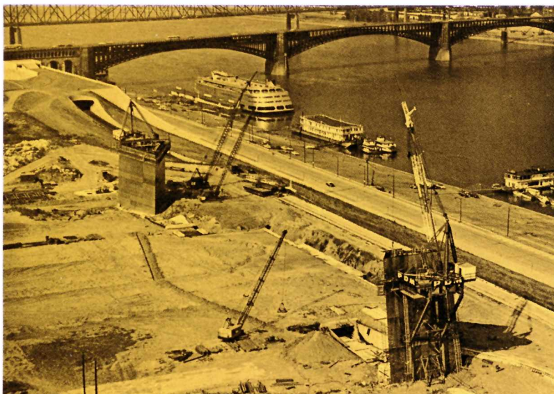
The "legs" of the Arch begin their ascent as the underground Visitor Center between them is covered with earth.
