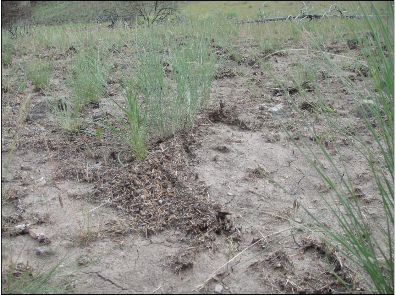
Figure 2. Debris and exposed bare ground from the late April thunderstorm that produced flash flooding and considerable erosion.
