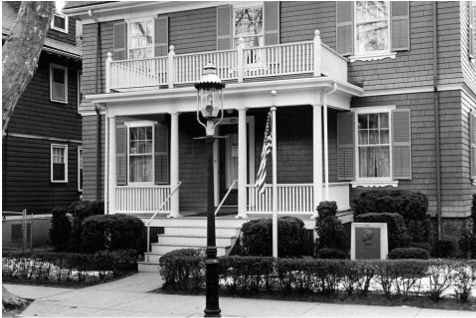
Figure 13. View of northwest elevation in January 1975. Most arborvitae have been transplanted to the side yard and additional yews have been planted. Note the gas light and flagpole (JOFI Management Records).
