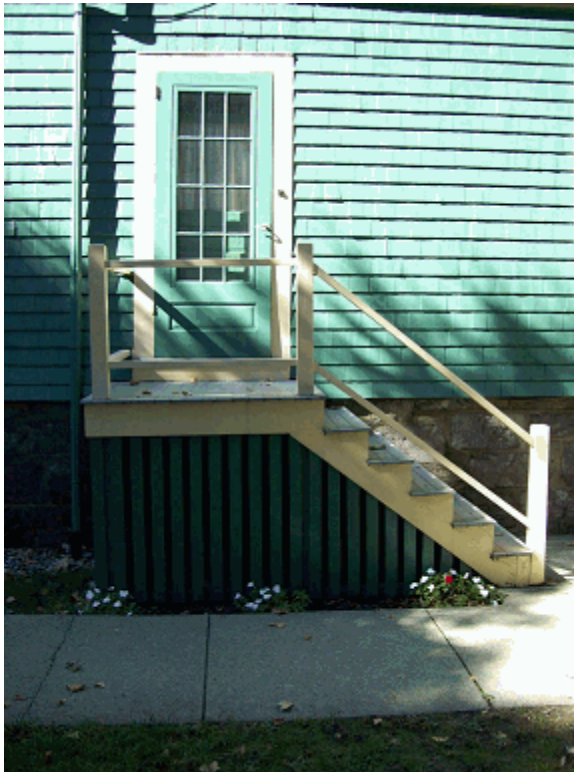
Figure 21. Wooden steps leading to rear entrance of the house (OCLP, 2008).
