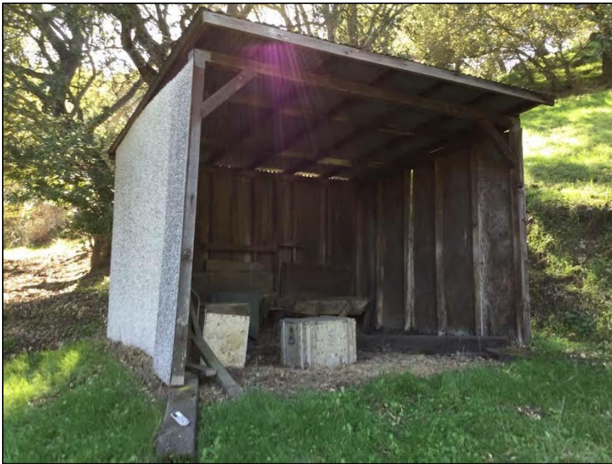
Buildings and Structures #1. View of three-sided wood-framed shed, view south (NPS, March 2024).
