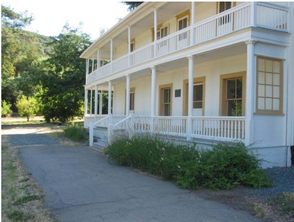
Circulation #6: The remains of the Martinez Adobe driveway. Just past the stairs, the paving is replaced with gravel. (OCLP, 2003)
