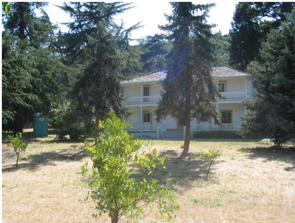
Buildings and Structures #1: View of the Martinez Adobe from the front, including several spruce trees, a redwood, and a quince. (OCLP, 2003)
