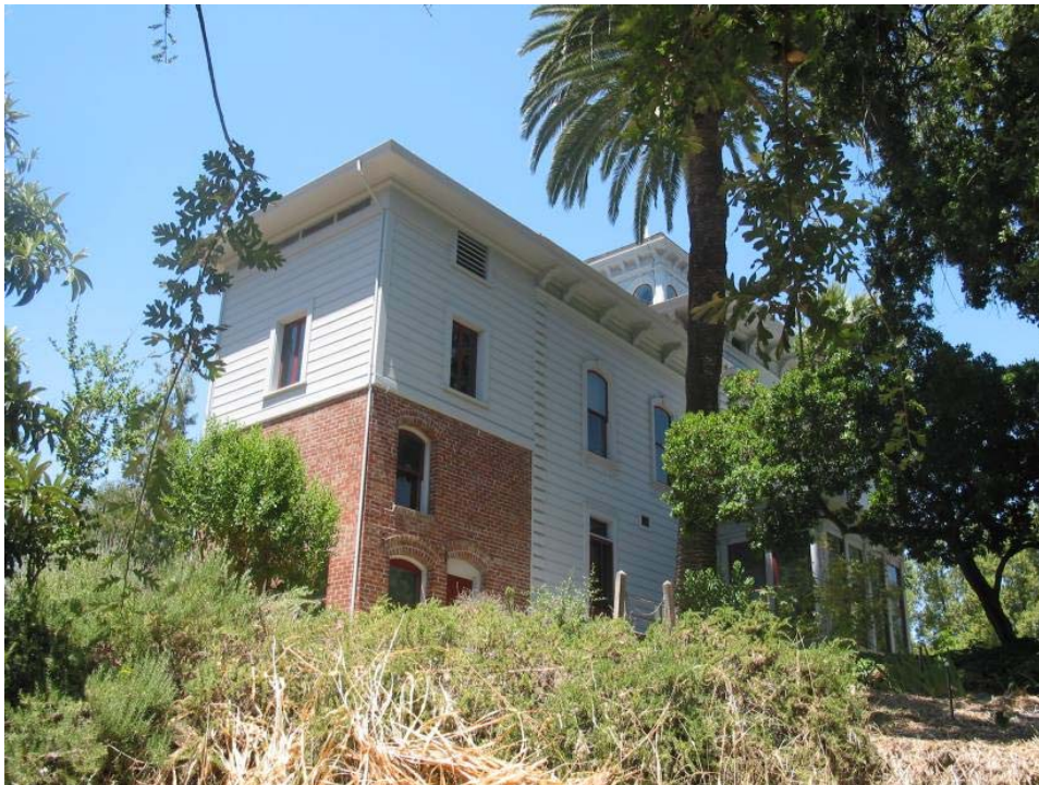
Buildings and Structures #3: A view of the kitchen addition at the rear of the Muir House. A Canary Island palm is located right of center. (OCLP, 2003)
