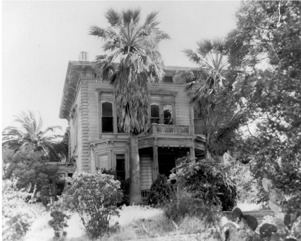
History #16: View looking south at the northwest porch of the Muir House, in 1960. (HABS, CAL-1890, 7-MART, 1-6, by Jack Boucher)
