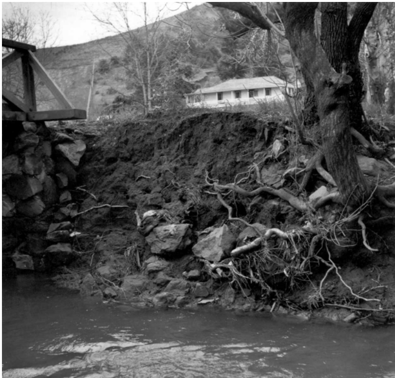
History #19: Flood damage along Franklin Creek in 1970. (Photographer and catalog number unknown. From Historic Structures Report: Franklin Creek Bridge. JOMU)
