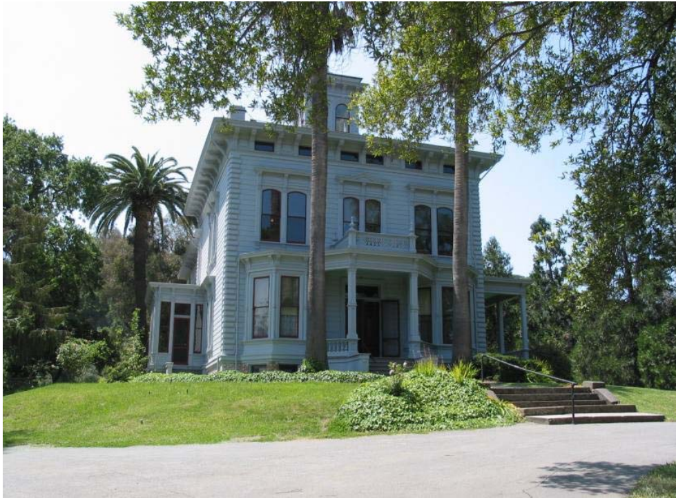
Buildings and Structures #2: Front view of the Muir House, including two California fan palms flanking the entrance and the southern part of the Carriage Drive-Loop. (OCLP, 2003)
