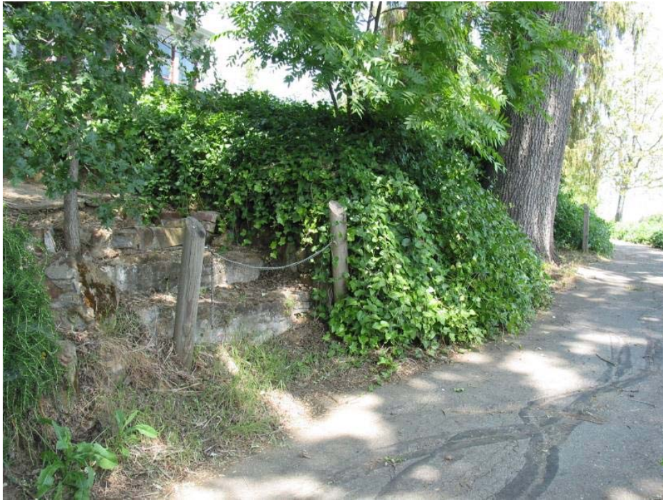
Circulation #7: View of the stone/brick walls and stone steps southeast of the Muir House. (OCLP, 2003)
