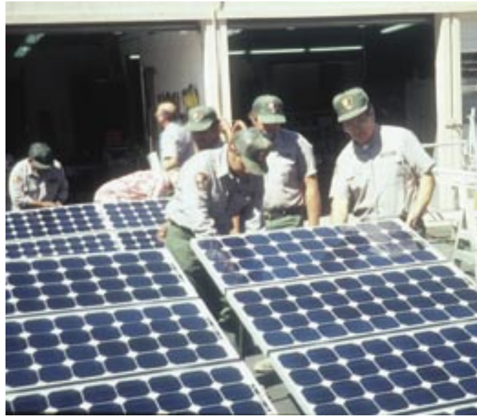
Maintenance staff preparing solar panels for the Cottonwood Spring photovoltaic installation.
