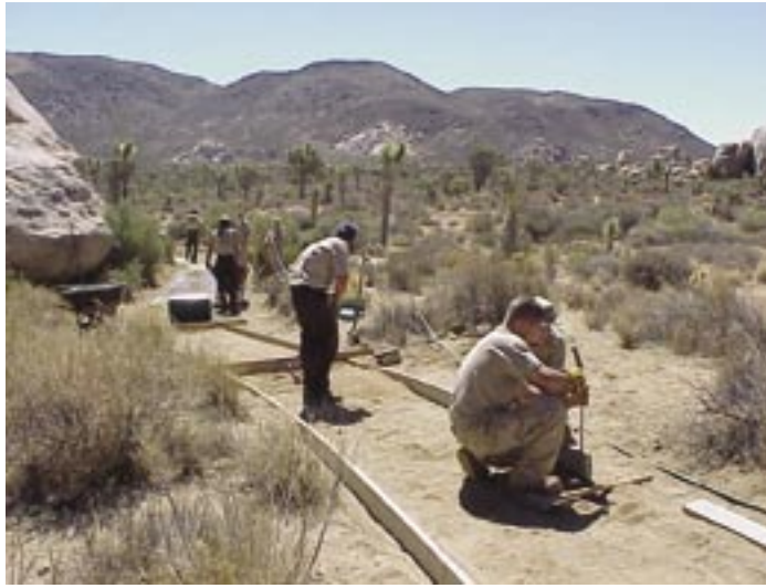
The park's trail crew worked with CCC and YCC youth groups to rehabilitate the handicapped-accessible Cap Rock Nature Trail.
