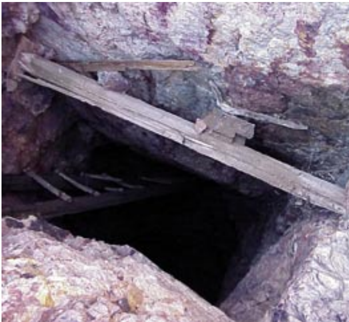
Abandoned mine sites pose a threat to visitor safety.
