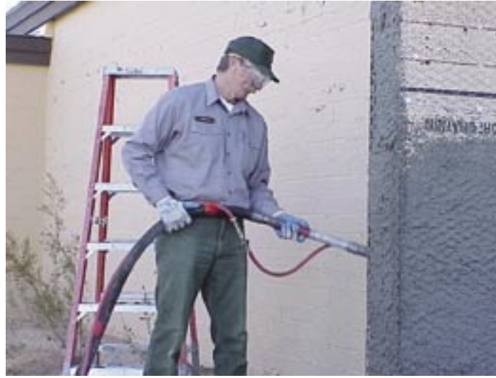
Resurfacing park buildings with stucco reduces heating and cooling costs.
