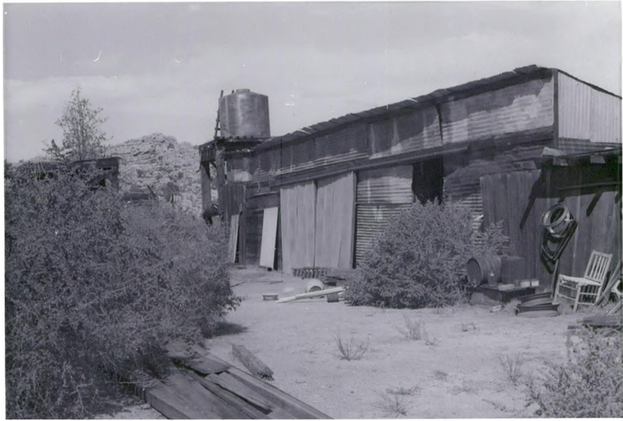
(Building O - Machine Shop)
