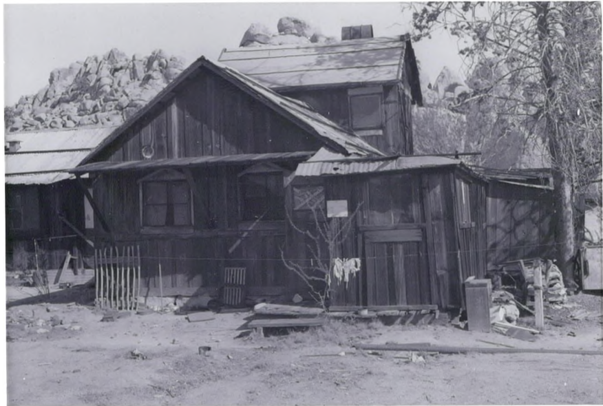
(Building A - Main Ranch House South Side)
