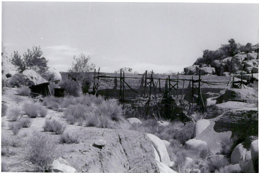
(Structure V - Dam, Downstream Side)
