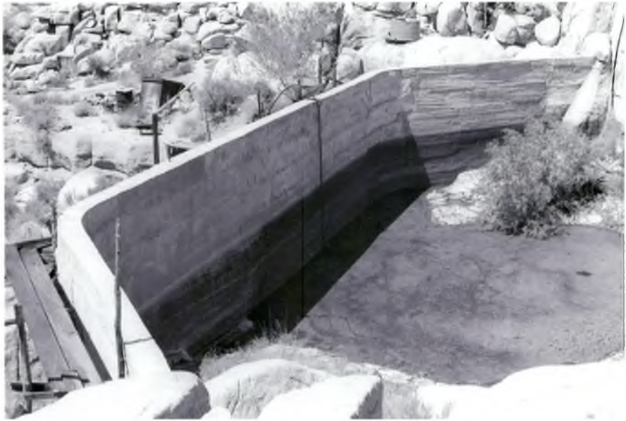
(Structure V - Dam, Upstream Side)
