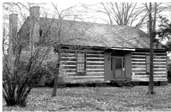
Kolb Farmhouse, post-restoration
