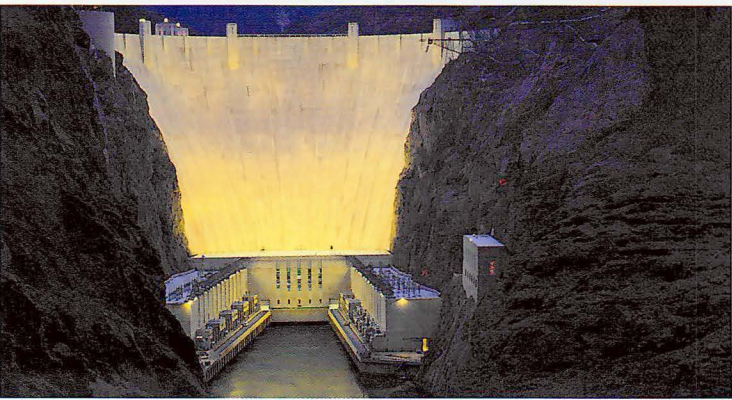
Hoover Dam's 45-foot-thick crest and 660-foot-thick base hold back Lake Mead.
