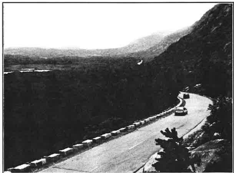
Historic Motor Road, Acadia National Park. The Olmsted Center has prepared a number of studies for the Motor Road including design guidelines for Federal Highways Administration rehabilitation work.
