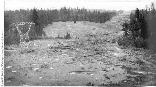
OPPOSITE PAGE, TOP: Line clearing operations and tower erection were among the first steps in building a Bonneville transmission line.
