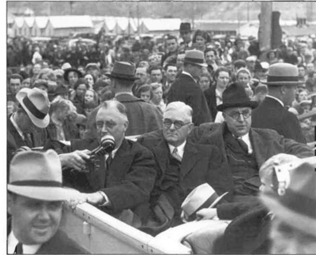
Franklin D. Roosevelt (behind the microphone), who visited the Grand Coulee Dam site in 1934, was an avid supporter of the dam project, public power, and irrigation of arid lands.
