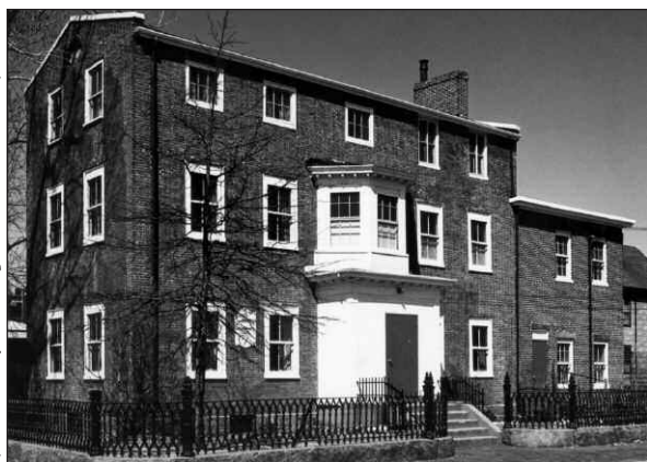
Cambridge Neighborhood House, 79 Moore St., demolished 1973
