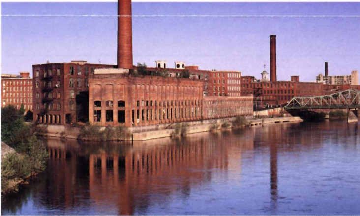
Massachusetts mills, in the foreground, and Boott Mills, beyond the bridge over the Merrimack.
