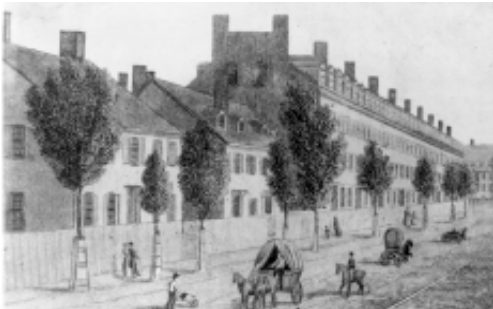
Merrimack Manufacturing Company boardinghouses, 1848.
