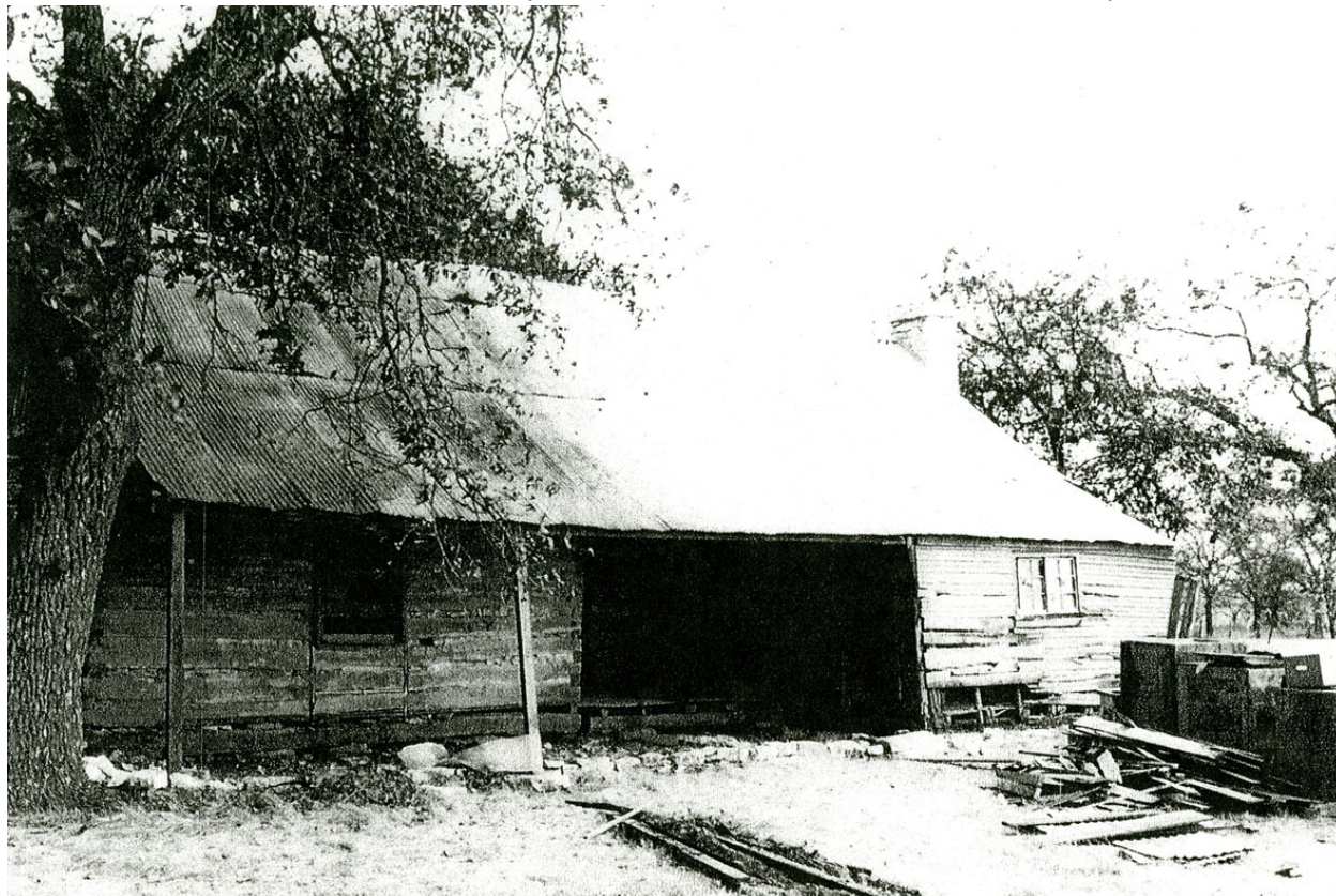
Johnson log cabin (HB-7), south elevation, prior to restoration, circa 1970-1971 (Source: LBJ National Historical Park Archives).
