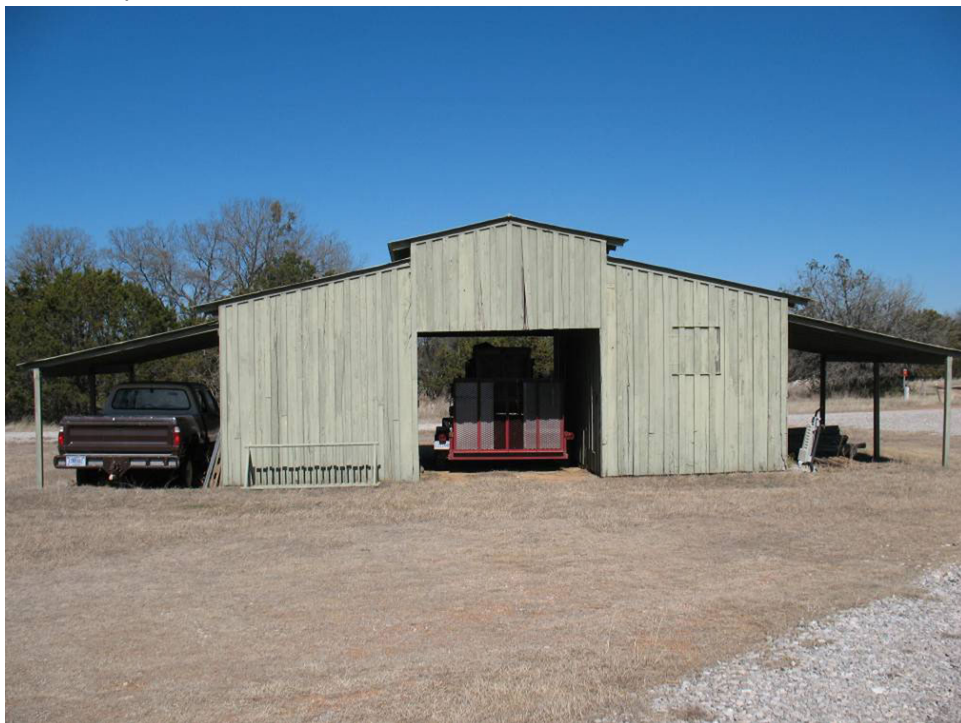
"Back 40" tack and feed storage building (BLDG-56), facing north (Source: Author).
