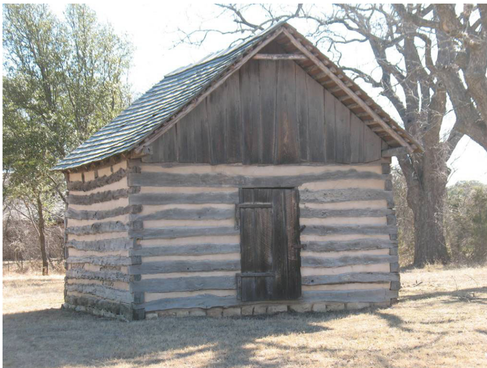
Reconstructed Johnson smokehouse (HB-8), facing north (Source: M. Frisbie).
