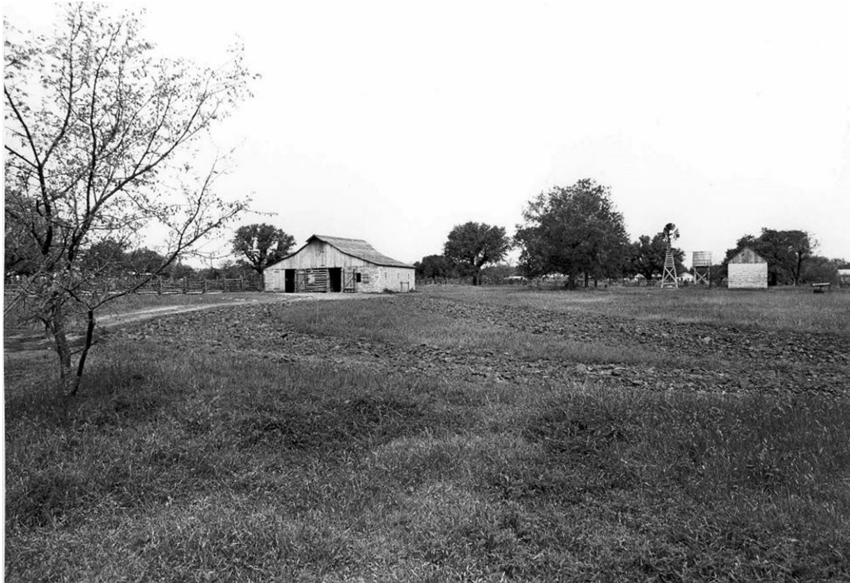
Restored James Polk Johnson barn (HB-11) and reconstructed fences with restored windmill (HB-78), water tank (HB-79), and restored well house (HB-12) in background, 1970s (Source: LBJ National Historical Park Archives).
