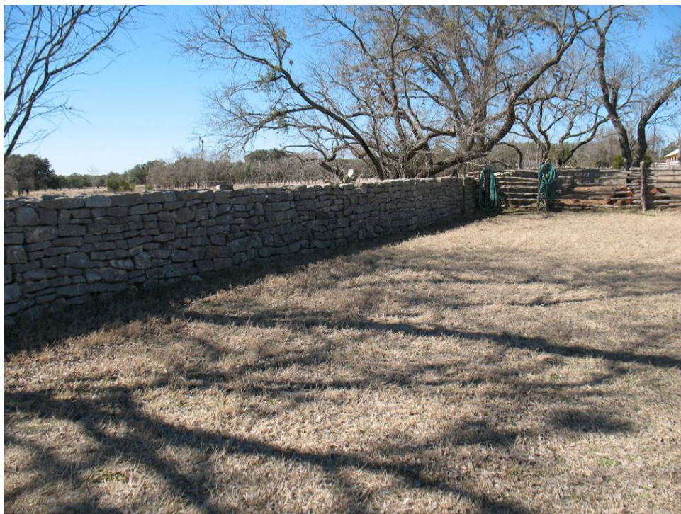
Reconstructed stone wall adjacent to the James Polk Johnson barn, facing southwest (Source: M. Frisbie).
