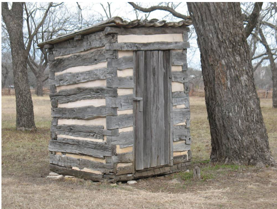
Reconstructed Johnson privy (HB-9), facing northeast (Source: M. Frisbie).
