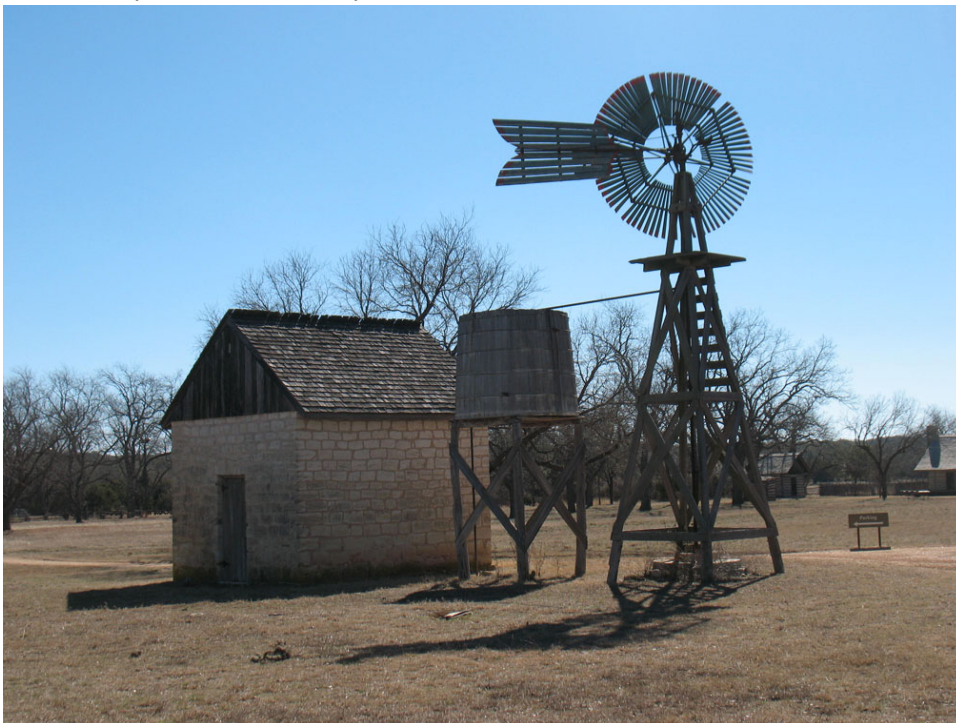
The architectural forms of the N.T. Stubbs well house (HB-12), water tank (HB-79), and windmill (HB-78) are important cultural traditions of the area, facing southeast (Source: M. Frisbie).
