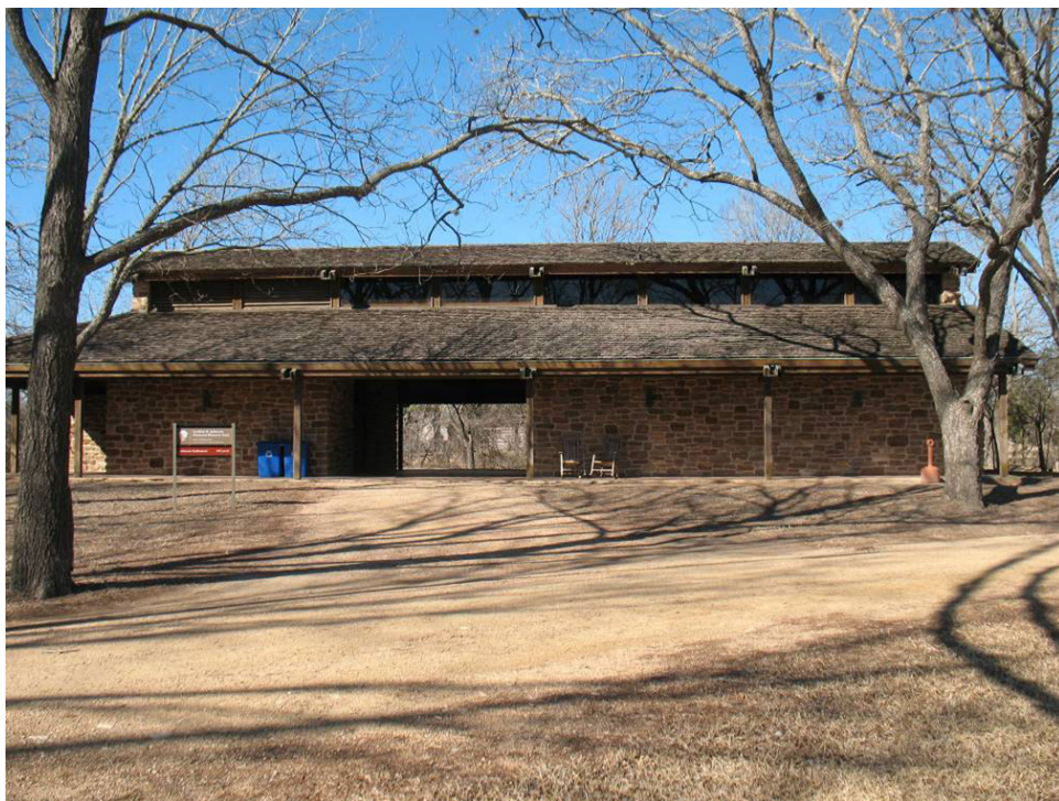
Johnson Settlement Area Exhibit/Event Center (BLDG-45), facing west (Source: M. Frisbie).
