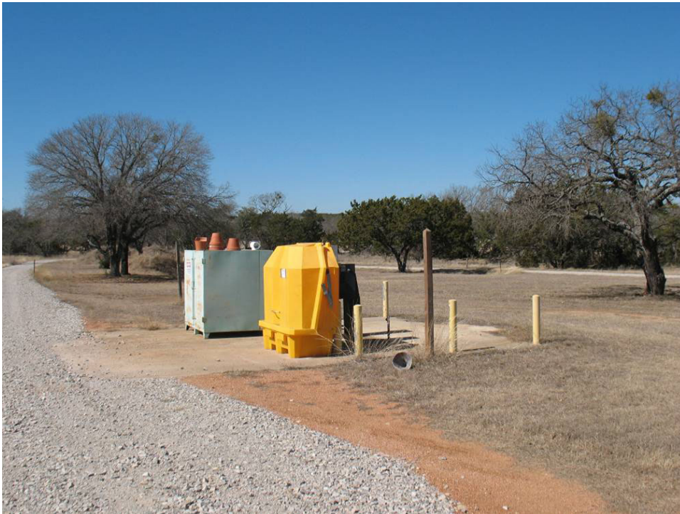
Utilities in the "Back 40" Area, facing west (Source: M. Frisbie).
