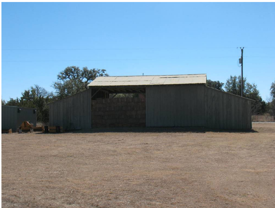
"Back 40" area maintenance building (BLDG-49), and small shed to the east, facing south (Source: M. Frisbie).
