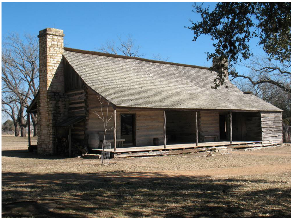
Restored Johnson log cabin (HB-7), facing northeast (Source: M. Frisbie).
