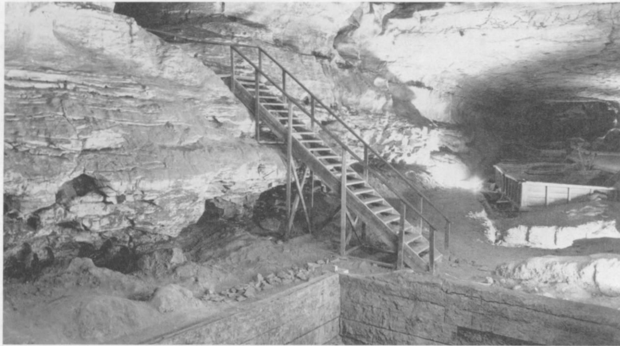
Figure 3—The Second Hoppers in Booth's Amphitheatre contain seven rectangular hoppers. The sump tank for the pump tower is located at the 2:00 o'clock position out from the base of the stair casing. Legs for the pump tower are used for a fence railing seen in the far right of the photograph. Photograph by Diana Emerson George.
