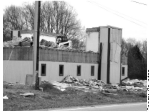
A bobcat clears the second floor at Chaumont.
