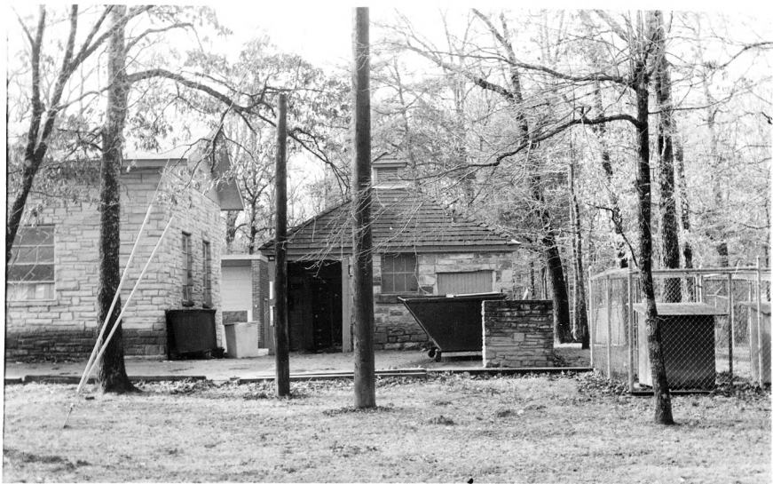
3. Paint Shed (060), Maintenance Area Mammoth Cave National Park, Kentucky
