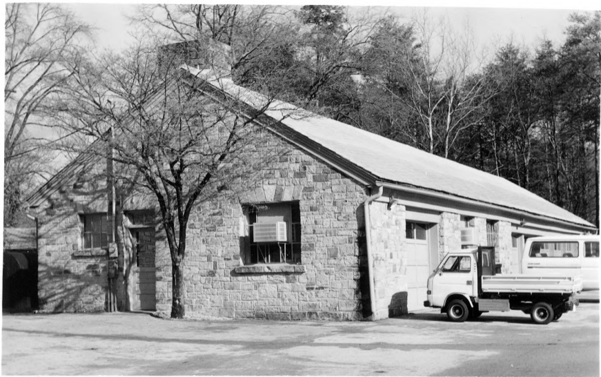
5. Repair shop (059), Maintenance Area Mammoth Cave National Park, Kentucky
