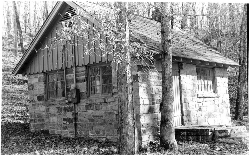
2. Three Springs Pump House (024) Mammoth Cave National Park, Kentucky
