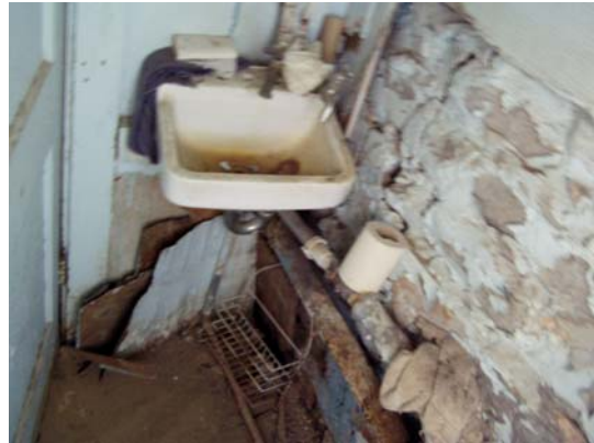
Downstairs basement bathroom
