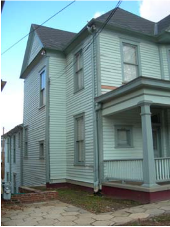
West elevation, looking north
