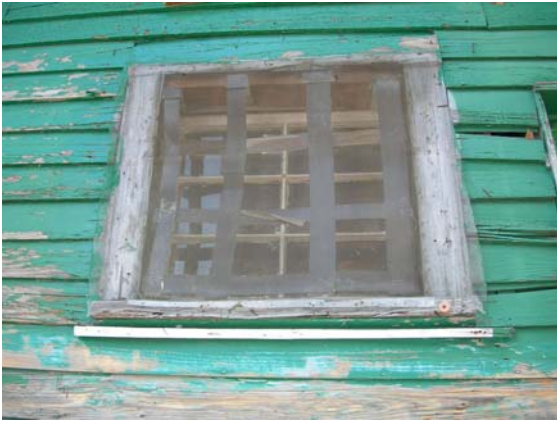
North window on west elevation, 2008
