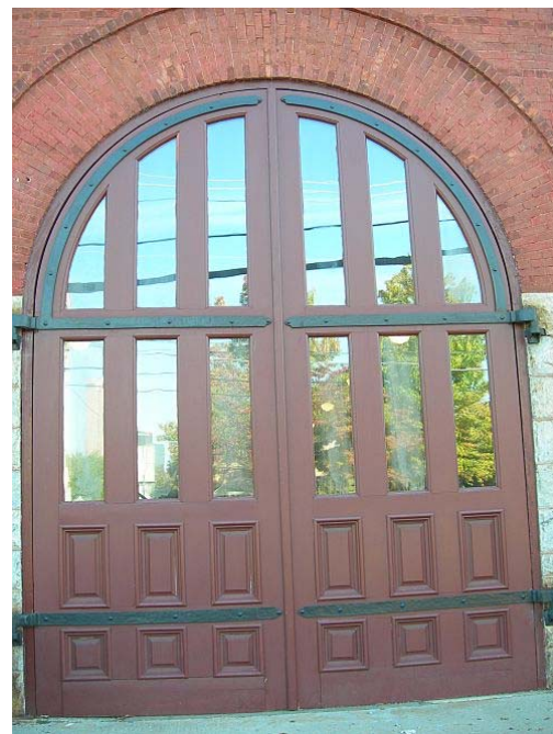
Fire truck doors on west elevation
