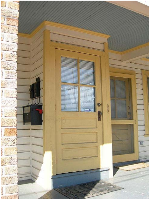
Eastern first floor entrance to staircase to second floor
