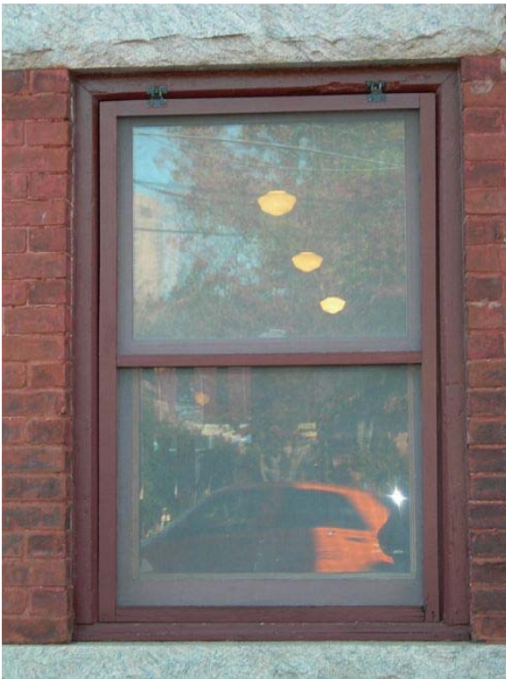
Window south of fire engine doors, showing typical screen construction
