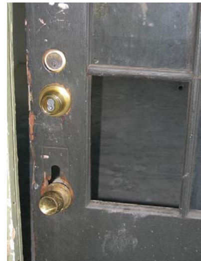
Detail of front door locksets and door handle
