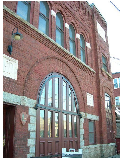
West elevation detail showing masonry details, doors, and windows
