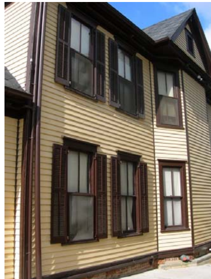
Typical windows on east elevation
