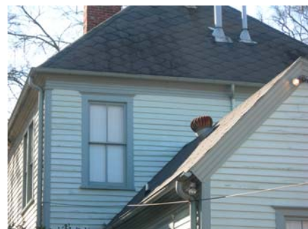
Second-story window, north elevation of main body of house
