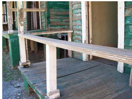
Typical front porch railing and flooring
