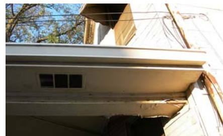
Porch soffit, vent, and gutter
