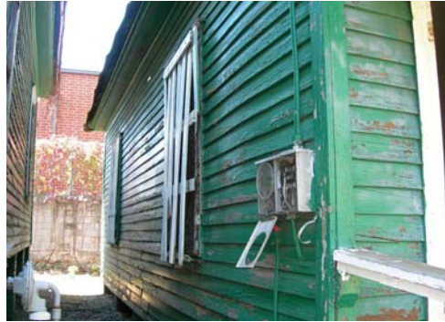
South elevation, looking west. Note wooden lattice window covers
