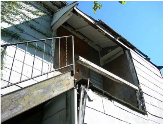
Detail of metal stairway attachment to south elevation of building
