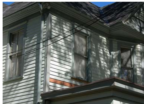
Typical windows and trim.
