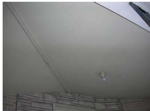
Front porch ceiling and light fixture
