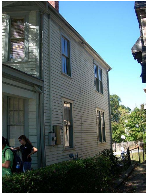
East elevation of house, looking north
