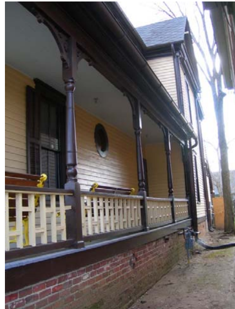
Detail of porch balustrade along west elevation
