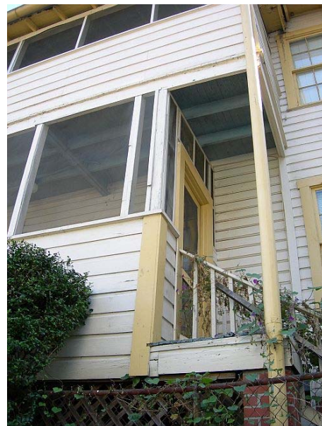
South elevation of first floor porch on west elevation
