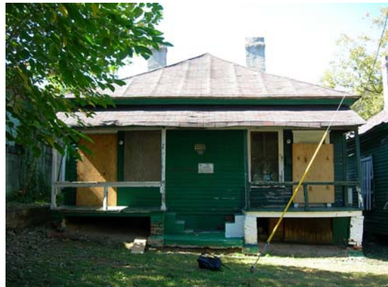
Alley House C Exterior, October, 2008, original site investigation
