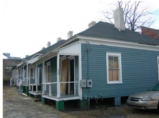
Work proceeding on Alley Houses, January, 2009
