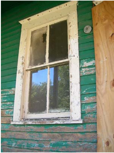
Typical window, east elevation
