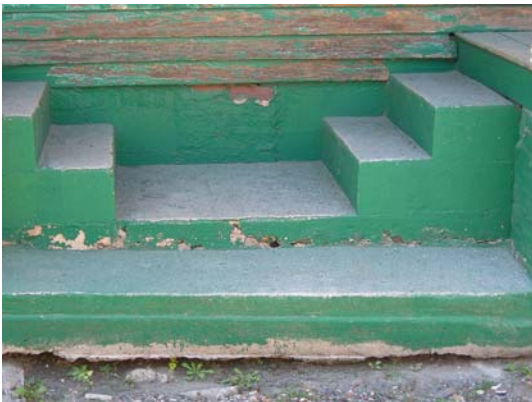
Access to front porches shows original grade of Reid's Alley
