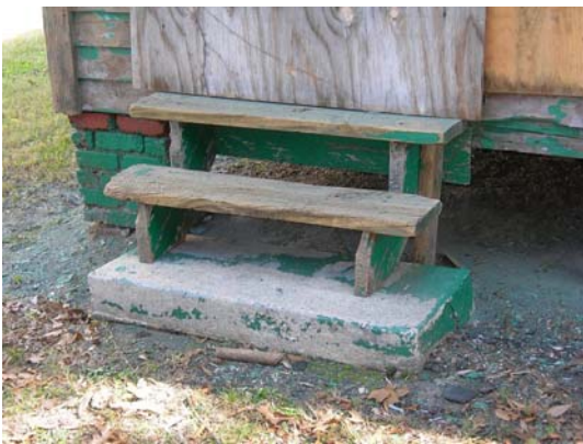
Stair to Unit 1, west side of building
