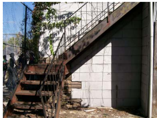
Back fire stairway to second story apartments.
