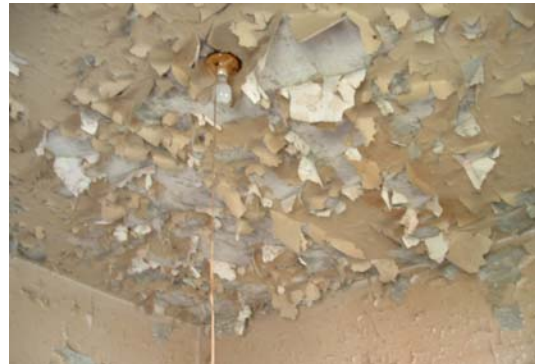
Typical ceiling condition with typical metal light fixture
