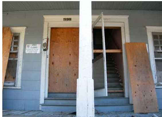
Entrance doors to upstairs apartments
