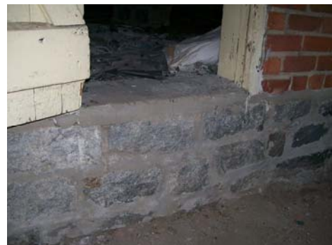
Stone foundation base at entrance to crawlspace
