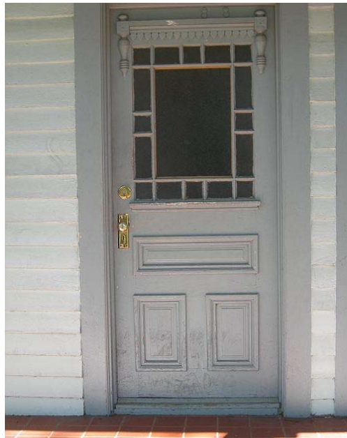
Front door, south elevation
