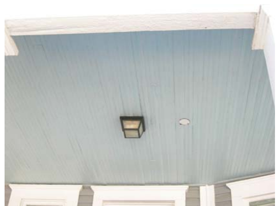
Wood single-bead board porch ceiling and modern light fixture
