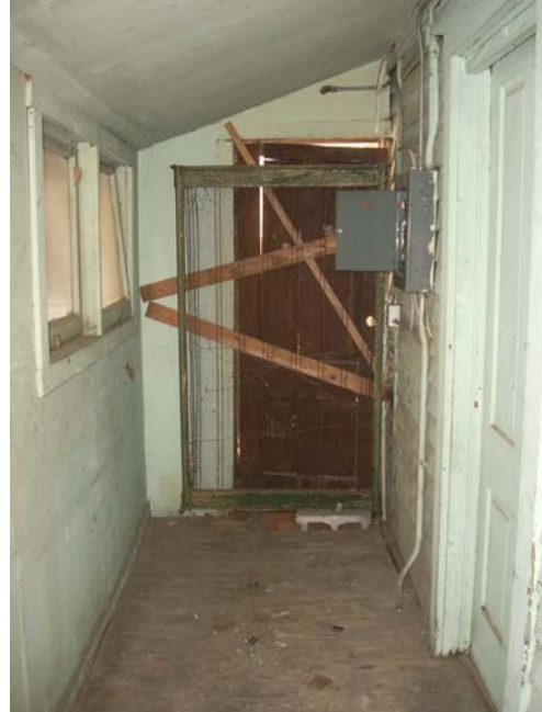
Enclosed back porch, looking east
