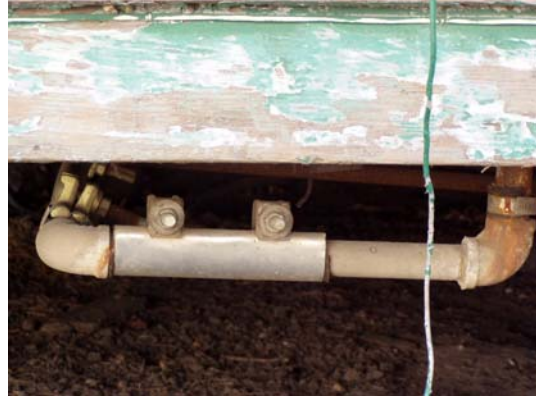
Repair of gas pipe beneath the building, west side
