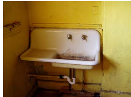
Kitchen sink in first-floor apartment
