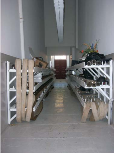
Fire hose chase, looking west from second floor to first floor door
