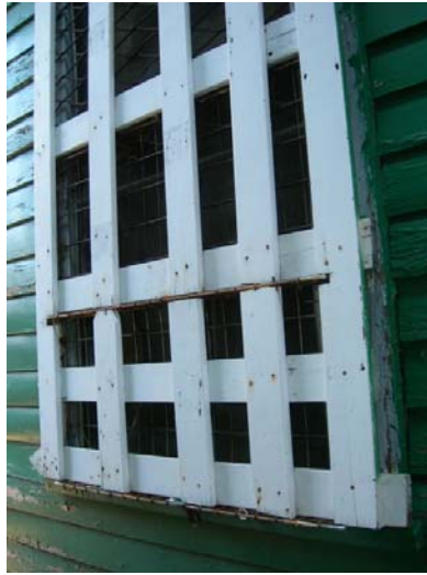
Wood lattice and wire mesh over window on south elevation, 2008.
