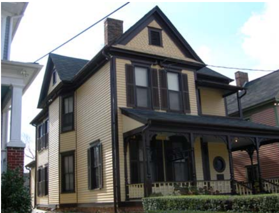
North and east elevations
