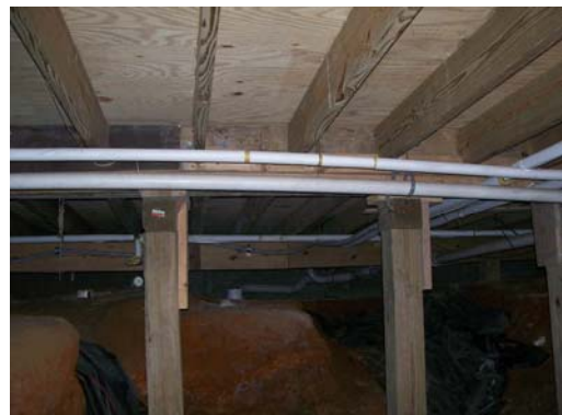
Supplementary floor supports in partial basement
