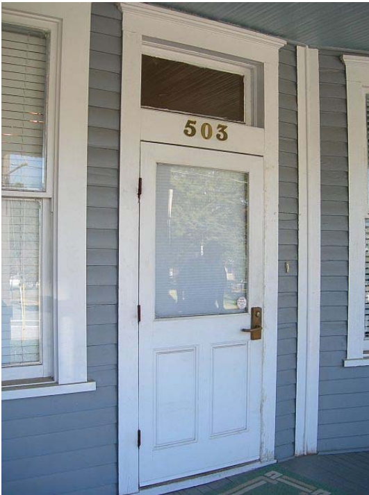
Front door and transom and typical door and window trim
