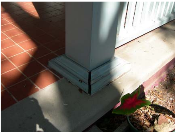
Detail of column base and porch balustrade
