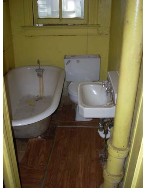
First floor bathroom
