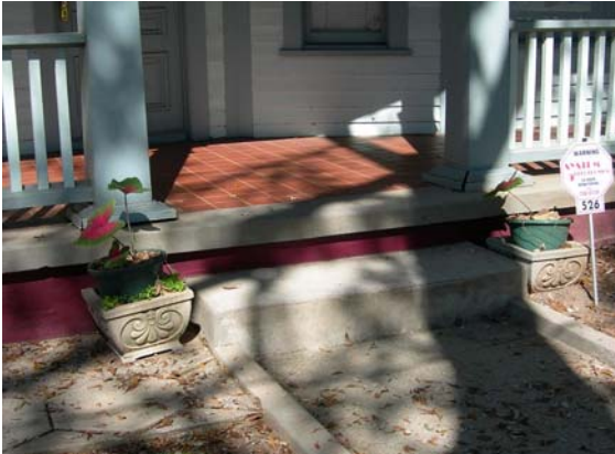
Front porch step, columns, and balustrade
