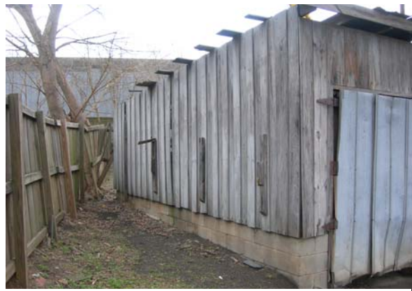
Remnants of former construction on northeast elevation of building
