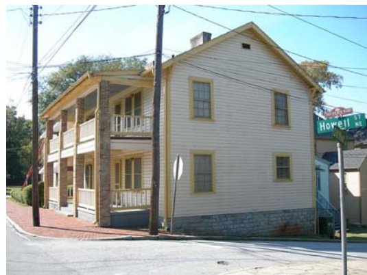
North and east elevations
