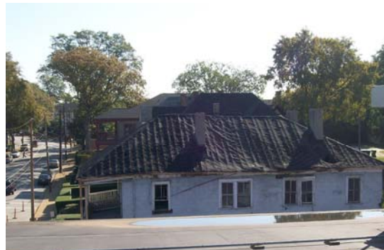
Roof, west elevation
