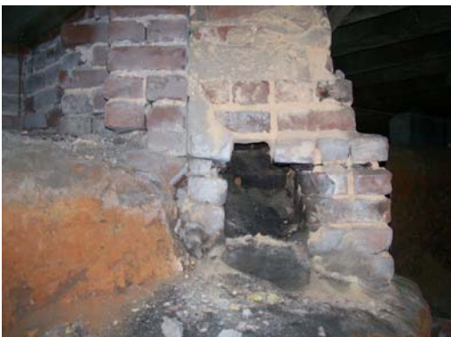
Ash-trap in partial basement is a historic feature
