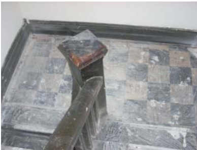
Tile floor on stair landing
