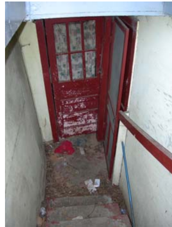
Lower level of stairway to basement
