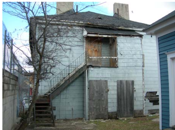
South elevation with metal fire stairs
