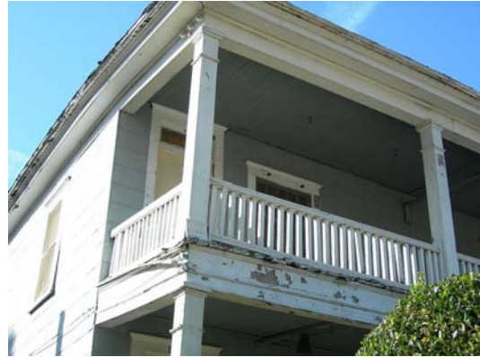
Second floor front porch railing
