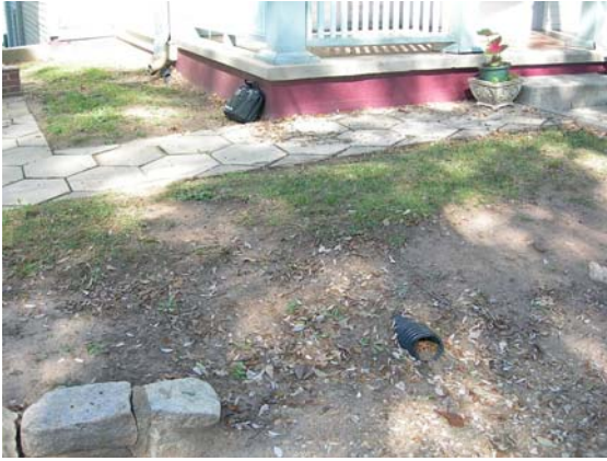
Front yard west of house.
