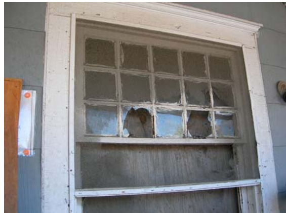
Typical fifteen-over-one double-hung windows with combination storm/screens in north elevation
