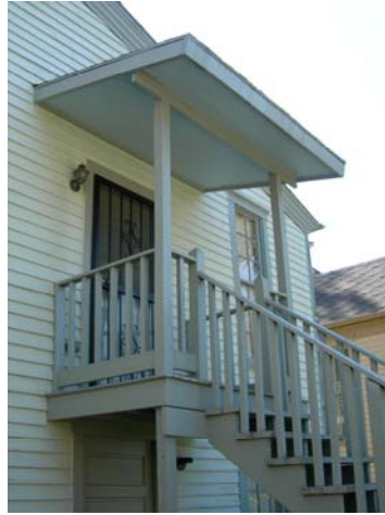
Upper level security door and covered entrance deck
