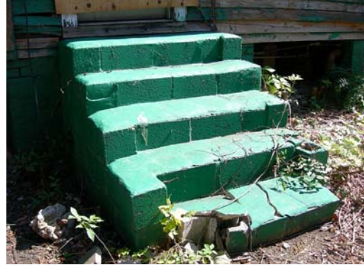
CMU stairs to Unit 5 on west elevation
