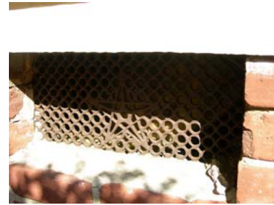
Basement vent grille in south elevation
