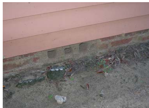
CMU crawl space vents on east elevation
