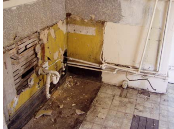
Former kitchen area
