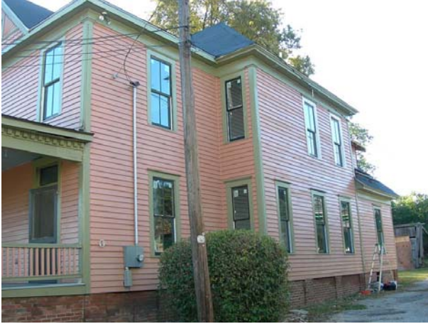
West elevation of building
