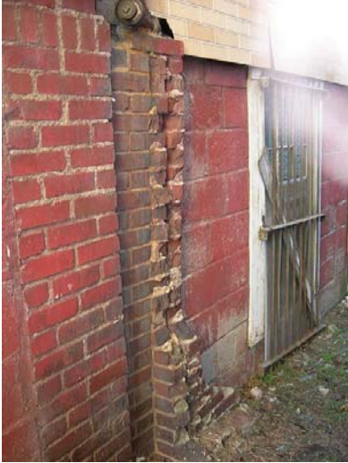
Construction of basement, north elevation
