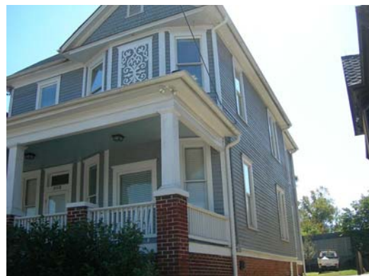
North and west elevations
