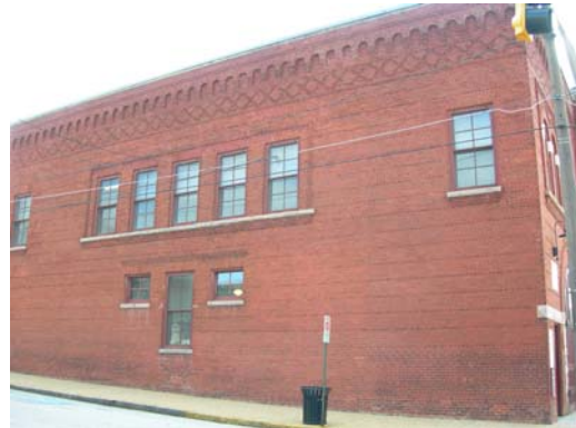
North elevation of Fire Station #6
