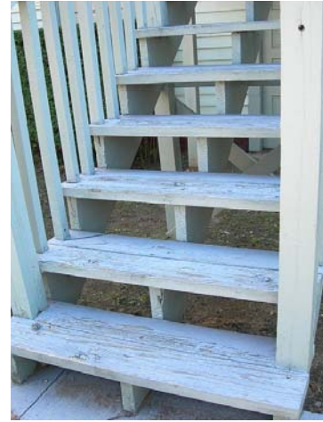
Wood stairs to upper level entrance deck
