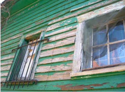
Windows on west elevation, 2008
