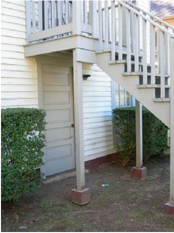
Typical exterior five-panel door and rear entry support posts
