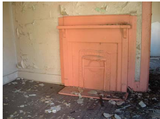
Fireplace in Unit 1
