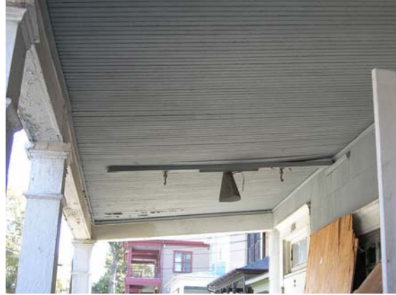
First floor ceiling, light, and porch swing brackets.
