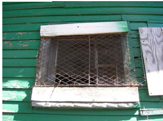
North window on west elevation, 2008
