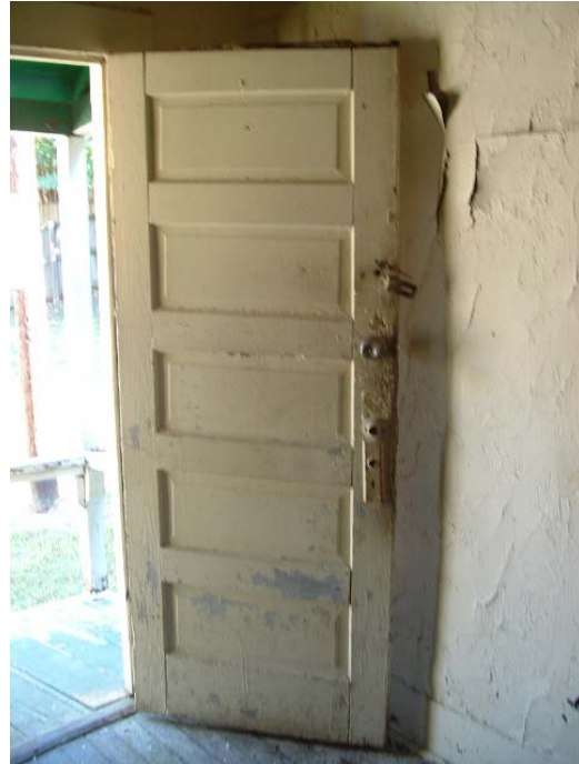
Typical five-panel exterior door
