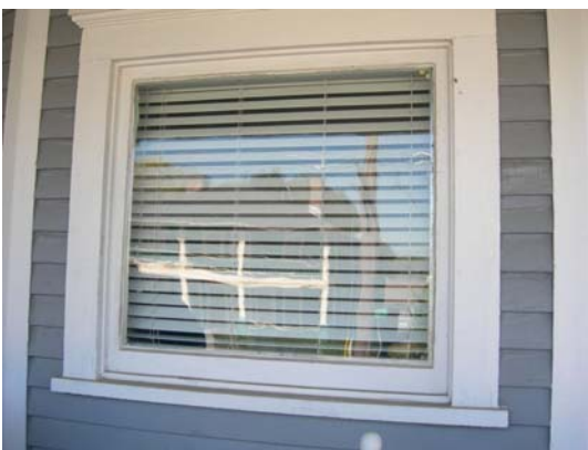
Single-light, fixed pane window on north elevation cut-away bay, first story
