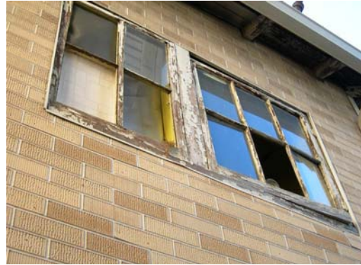
Windows on west addition, north elevation
