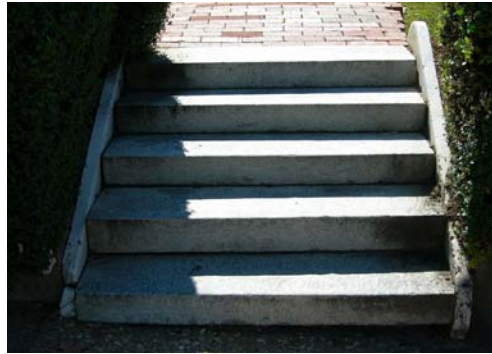
Granite approach stairs with marble cheekwalls
