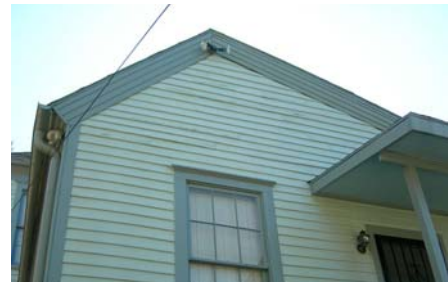
Detail of trim beneath roof on north elevation of rear addition
