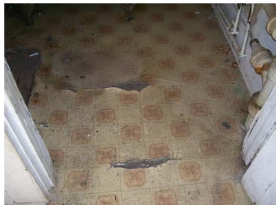
Rolled linoleum flooring
