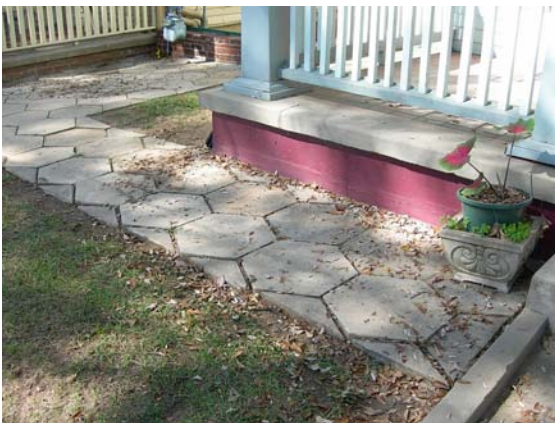
Walkway to west of front porch
