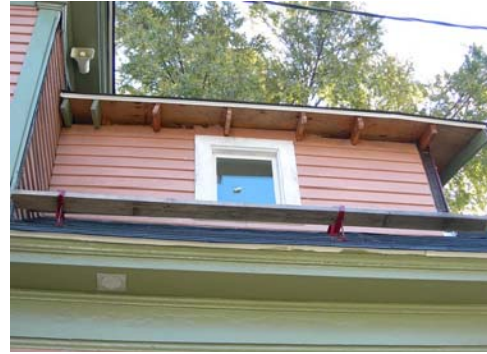
Unfinished work on rear addition dormers
