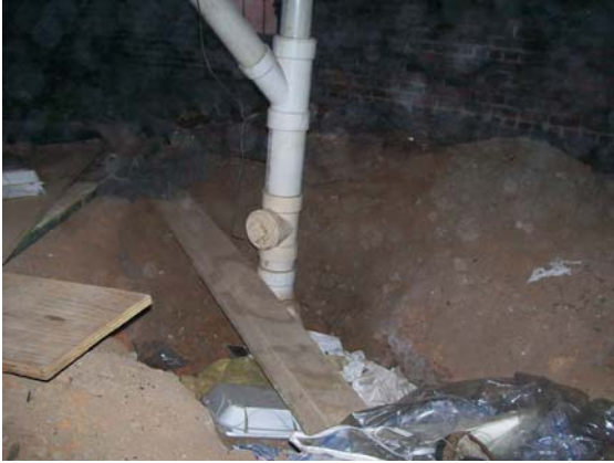
Replace excavated dirt at pipe installation
