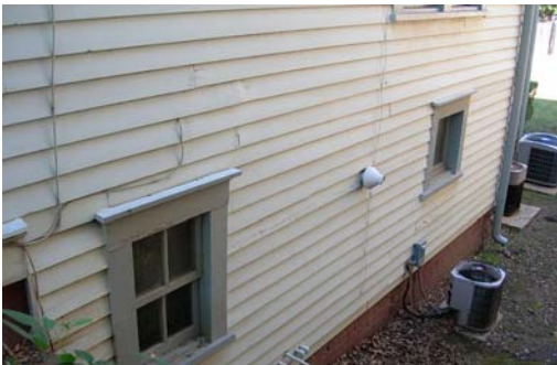
Basement windows, main body of house, east elevation
