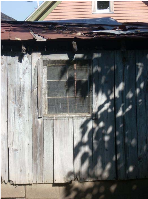
West window on southeast elevation
