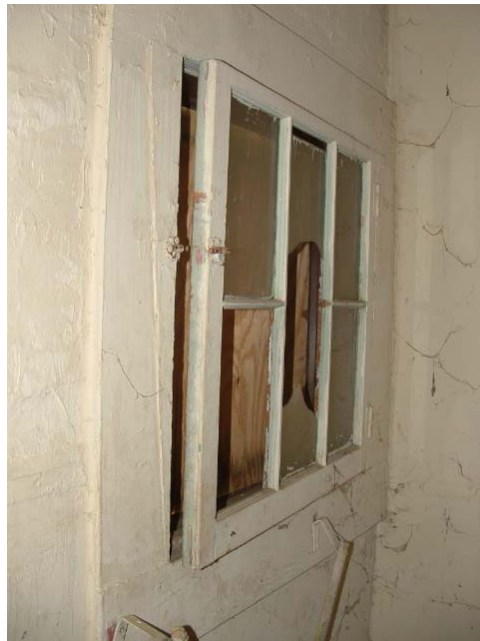
Typical bathroom window
