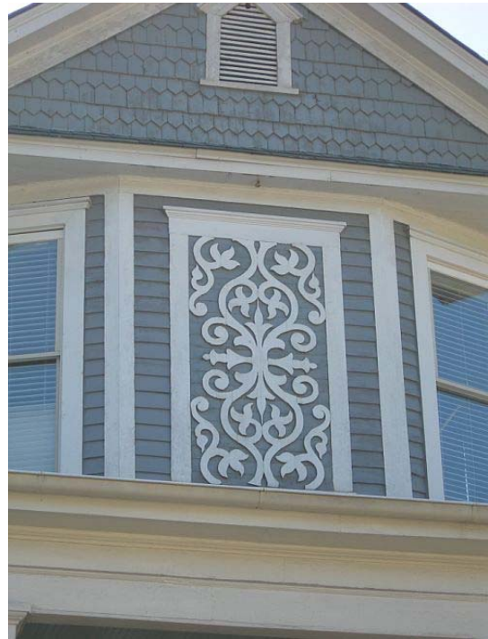
Patterned shingles, attic vent, and panel of “carpenter’s lace” on north elevation cut-away bay, second story
