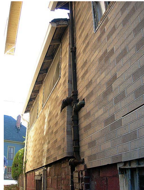
North elevation, showing cast iron sanitary piping on exterior
