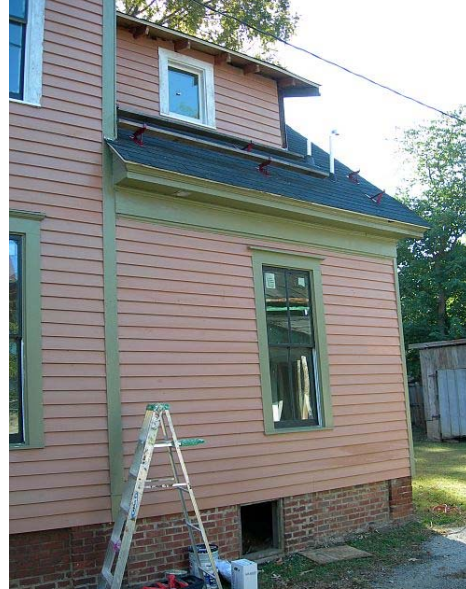
West elevation of gabled projection
