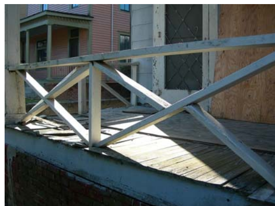
First floor porch floor and balustrade
