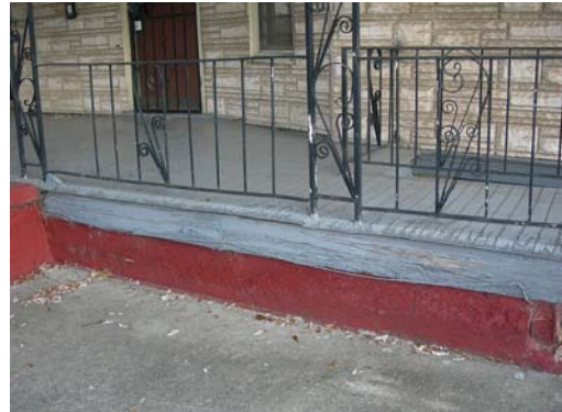
Front porch foundation, wood framing, and wrought-iron railing and porch supports
