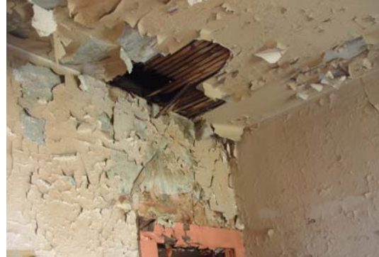
Typical wall and ceiling conditions
