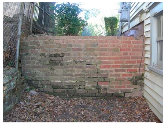
Brick retaining wall east of building
