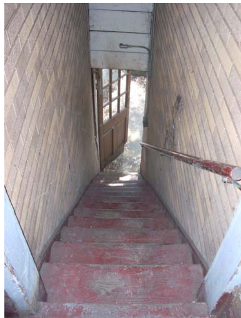
Stairs from second floor apartment to ground level
