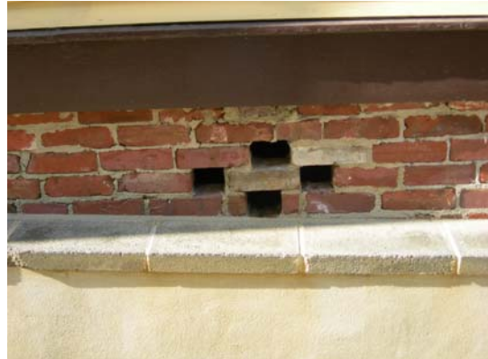
Vents in brick foundation wall on east elevation only
