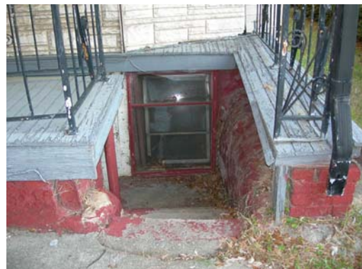
Entrance to basement apartment
