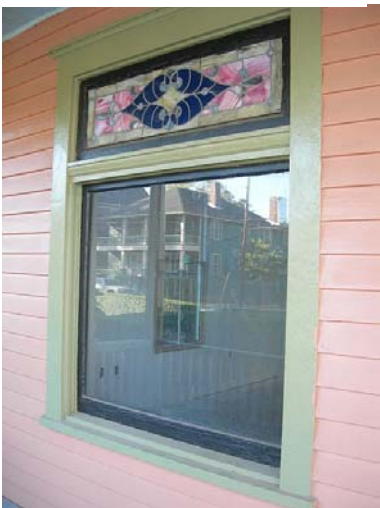
Historic window on north elevation
