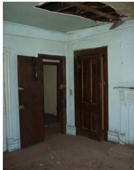
Typical trim and finishes
