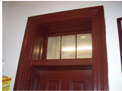
Original door, transom, and trim
