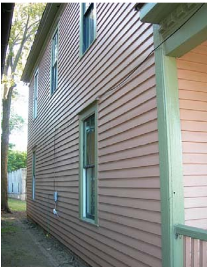
East elevation of building
