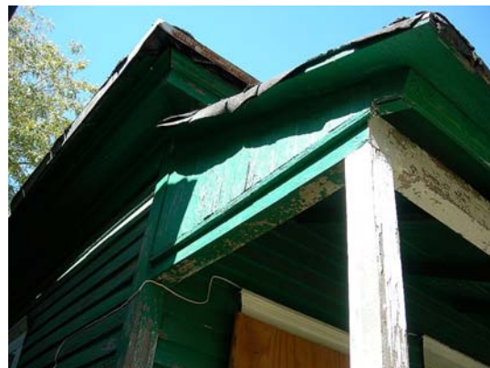
Detail of shed roof of front porch
