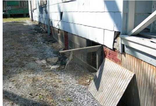
Detail of east foundation, crawlspace entrance, and composition shingle siding
