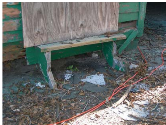
Stair to Unit 2, west side of building
