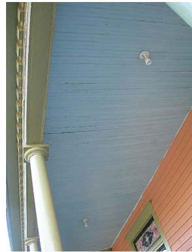
Dentil molding, round porch columns, and single-bead board porch ceiling
