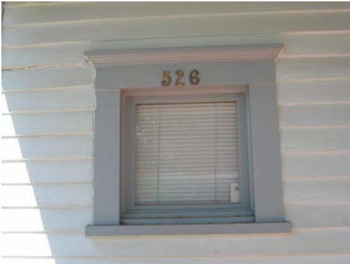
First floor window on west side of south elevation
