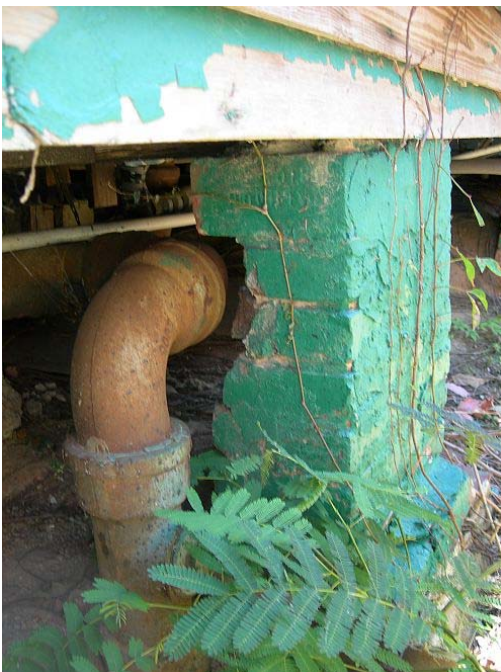
Brick pier modified for sanitary piping
