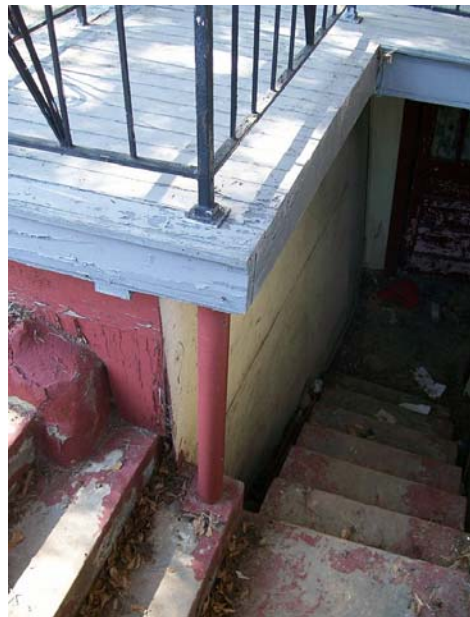
Tubular steel support of front porch at basement access
