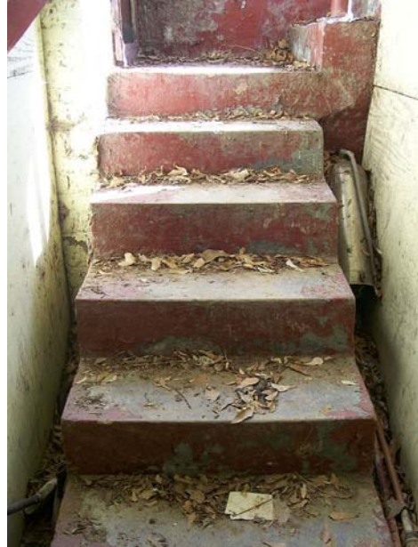
Access stairs to basement apartment, south side of building
