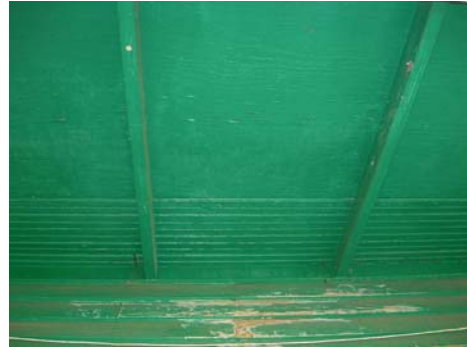
Typical porch roof decking
