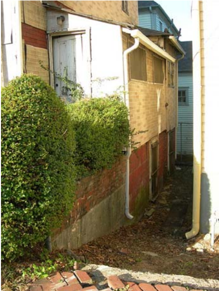
North elevation, showing retaining wall and single-story extensions with basement
