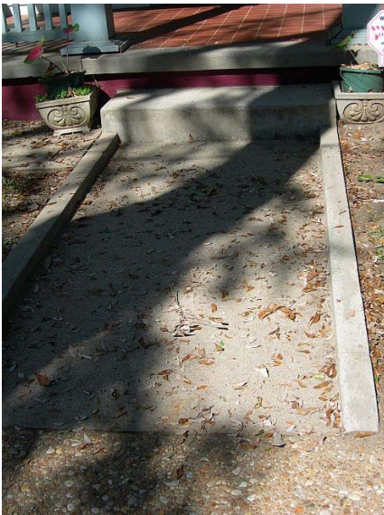
Concrete-edged concrete walkway to front porch
