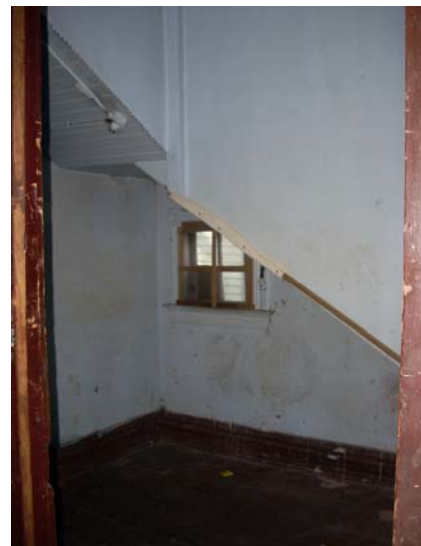
First floor room with added stairway to second floor
