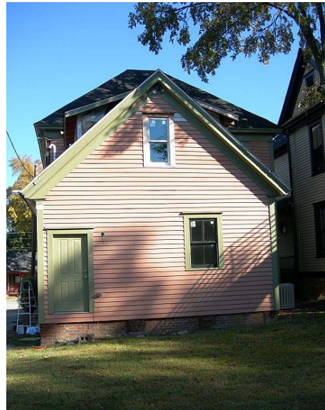
South elevation of building and view of rear yard
