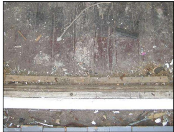
Figure 8 – Detail of furring strip in room 101
