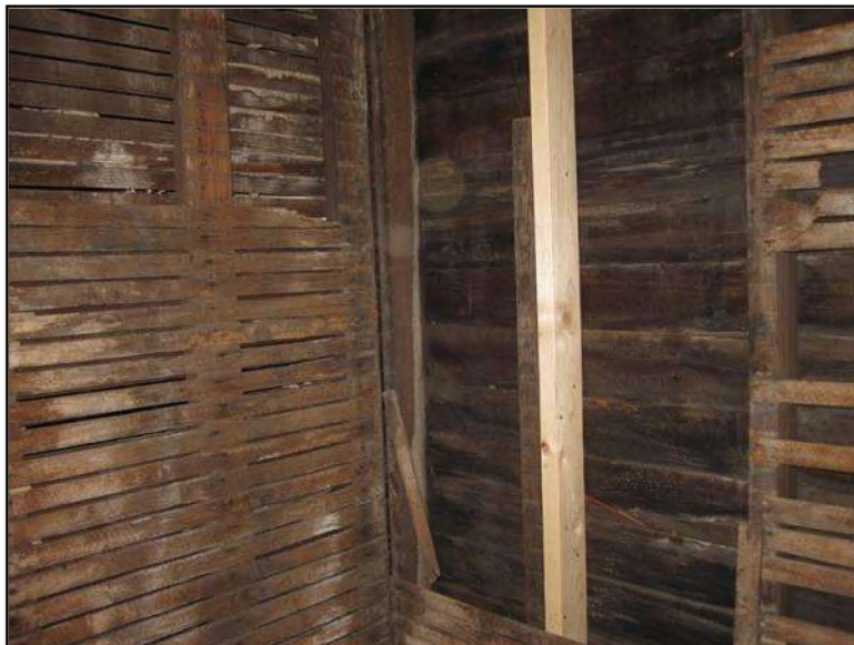
Figure 1 – Clapboard installed without sheathing, room 207, southwest (courtesy of Adam Archual)
