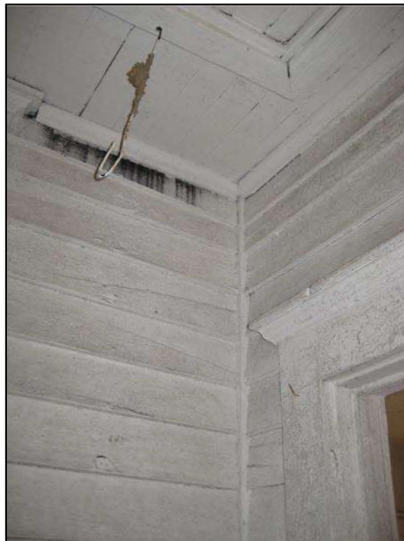
Figure 4 – Historic clapboard shown in room 205, northwest
