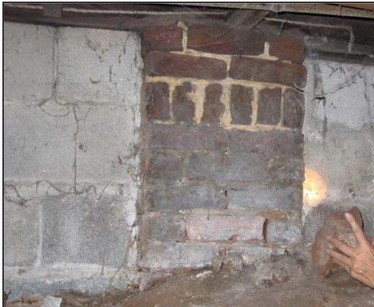
Figure 3 – Brick pilasters and CMU viewed from within crawlspace, looking east
