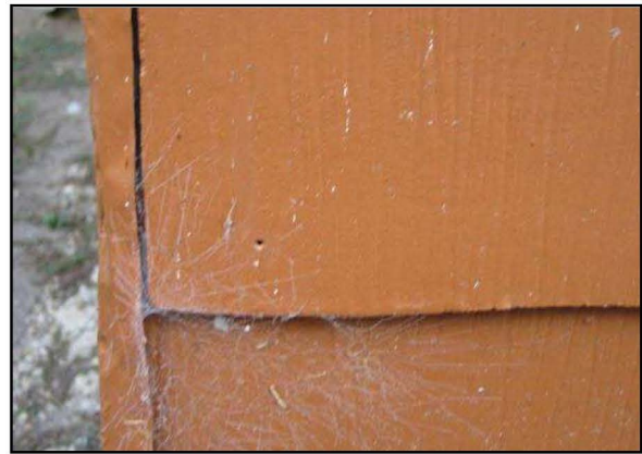
Figure 16 – Detail of nail holes, southeast corner
