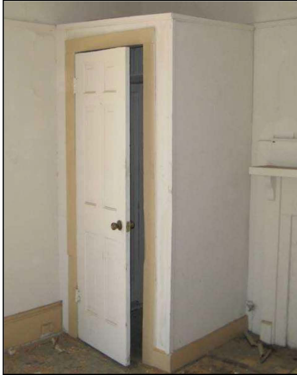
Figure 22 – Non-historic closet in room 201, southeast
