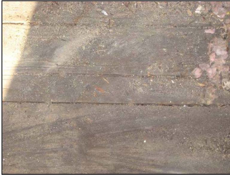
Figure 6 – Detail of typical tongue-and-groove wood, room 202
