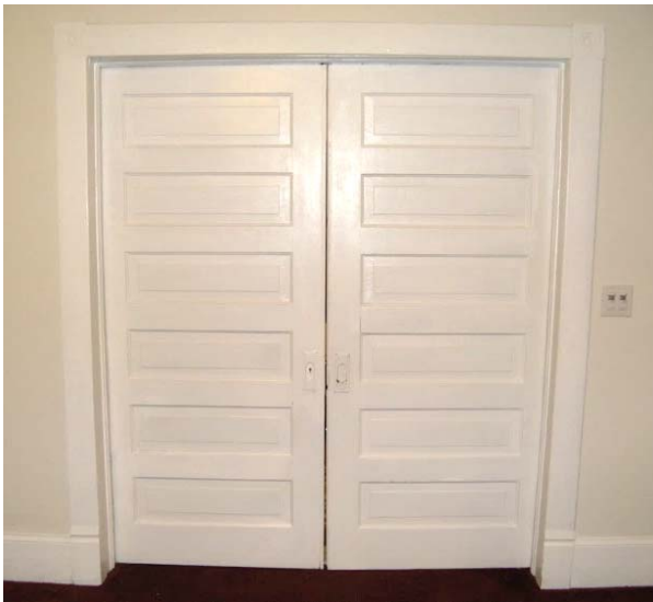
FIGURE 72. Remaining pair of pocket doors.
