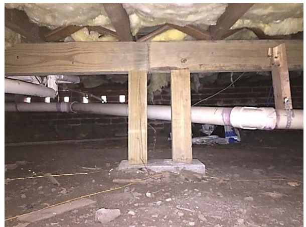
FIGURE 97. Replacement support posts at floor beam.
