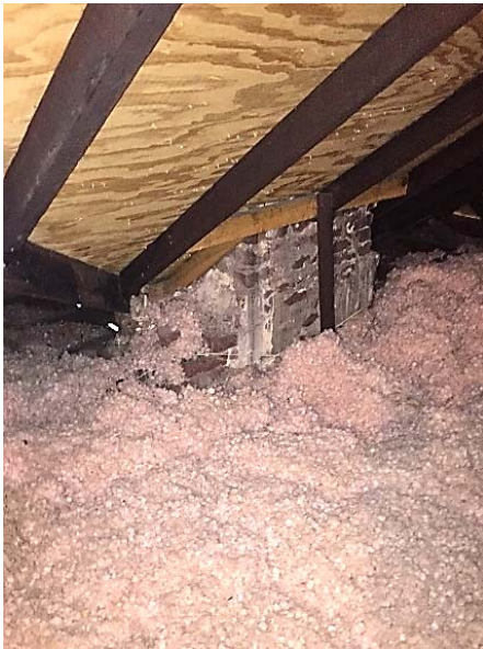
FIGURE 99. Ceiling framing has been covered with blown-in insulation.
