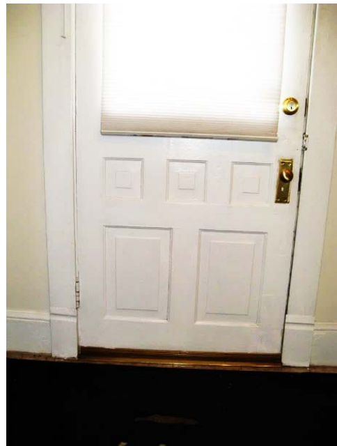
FIGURE 71. Interior side of primary front door.
