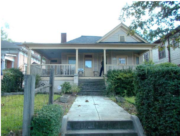
FIGURE 14. The concrete walk that extends from the sidewalk.
