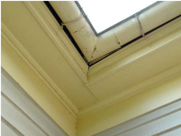
FIGURE 26. Roof eave with wood fascia and profiled trim.
