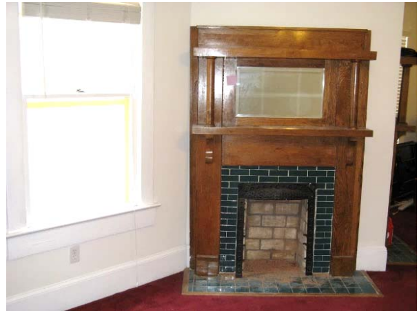
FIGURE 89. Fireplace in meeting room.
