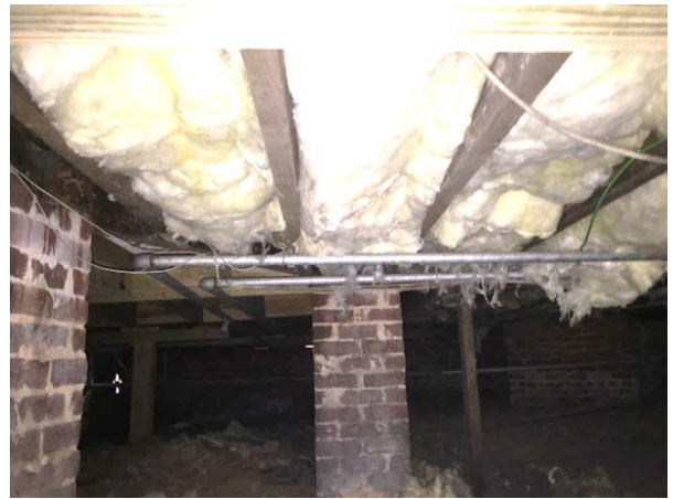
FIGURE 96. Overview of wood joints with batt insulation between joists.
