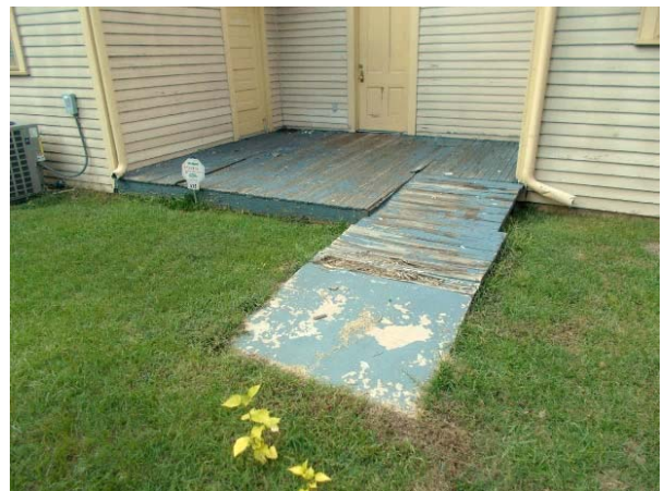
FIGURE 31. Overview of the south patio with concrete and wood access ramp and wood-framed platform.
