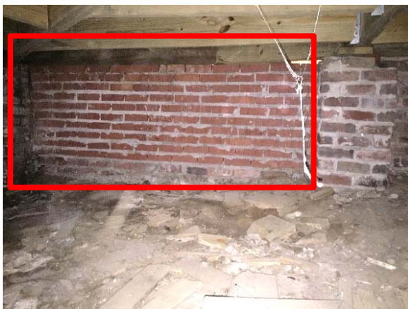
FIGURE 23. Infill brick between pier supports at foundation below north porch.
