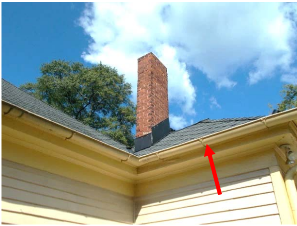
FIGURE 44. Typical gutter with gutter straps (arrow).
