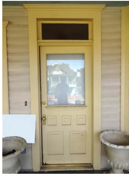
FIGURE 32. Main entrance door at north elevation, accessed from porch.
