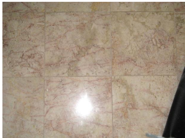
FIGURE 75. Tile flooring in foyer, installed in the early 2000s.
