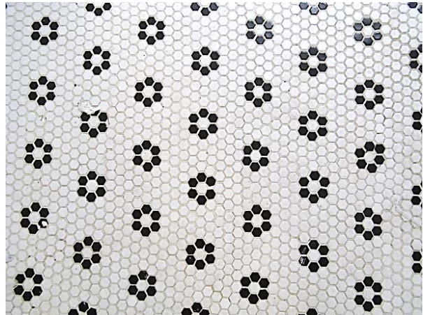
FIGURE 92. Ceramic mosaic tile floor in south bathroom. Note "daisy" pattern.
