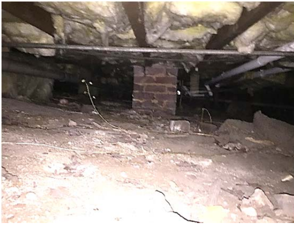
FIGURE 22. Brick pier foundation at center portion of house.
