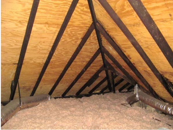
FIGURE 86. Attic with plywood roof sheathing and loose fill insulation.
