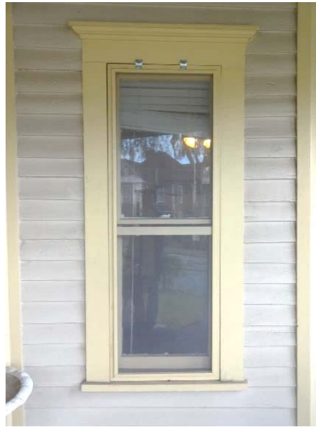
FIGURE 39. Typical window at north elevation.
