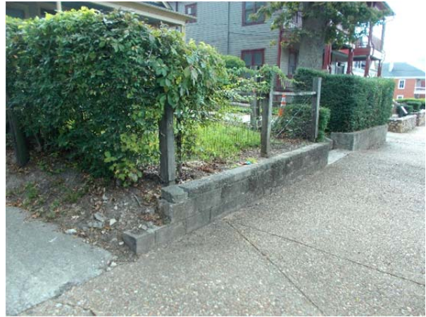
FIGURE 16. The retaining wall and wood-frame fence along the north edge of the property.
