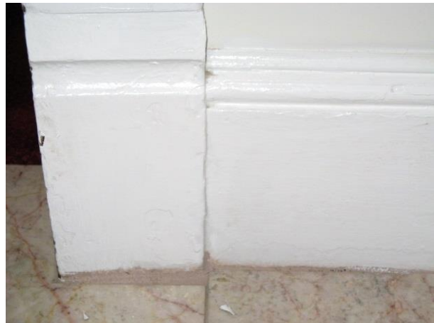
FIGURE 74. Typical plinth block and baseboard.
