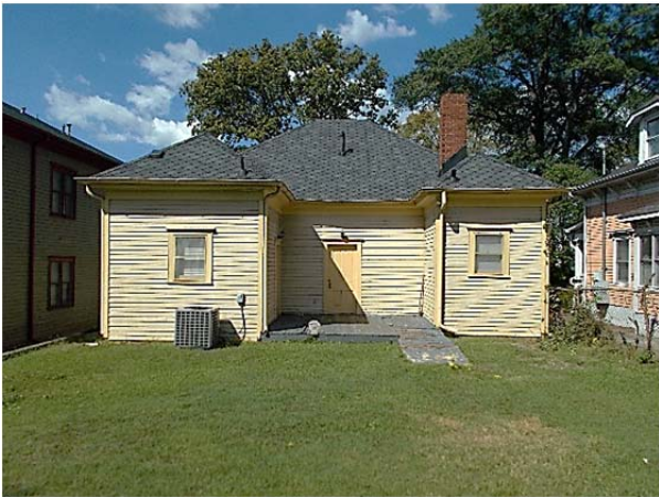
FIGURE 21. South elevation of the building.
