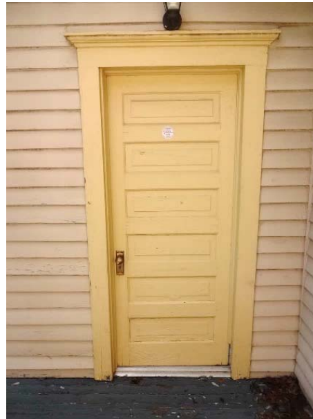
FIGURE 36. Door opening at west side of south elevation, accessed from patio.
