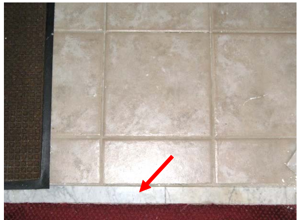
FIGURE 94. Porcelain tile floor in kitchen and laundry. Note marble threshold.
