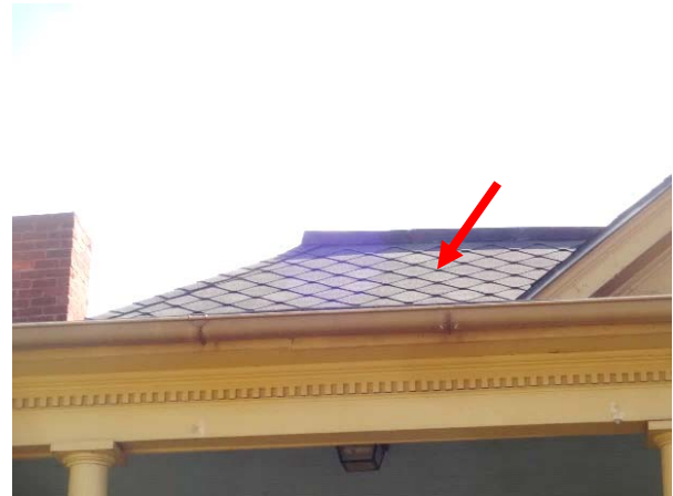
FIGURE 42. Roofing with asphalt-shingle diamond-shaped pattern.
