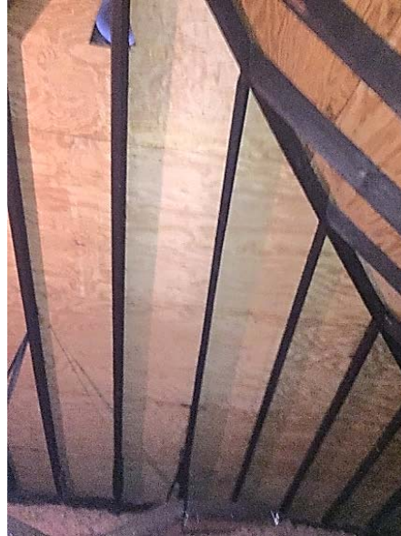
FIGURE 100. Overview of roof framing.
