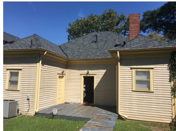
FIGURE 5. Rear, south facade, 515 Auburn Avenue, showing steep, complex roof line, decorative window and door moldings, and 1/1 windows.
