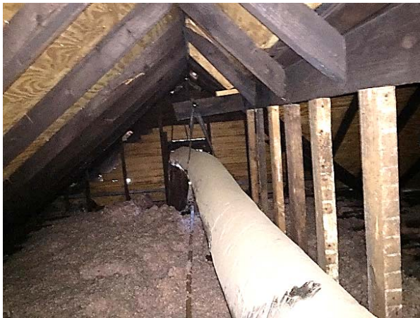
FIGURE 102. Overview of gable roof framing.
