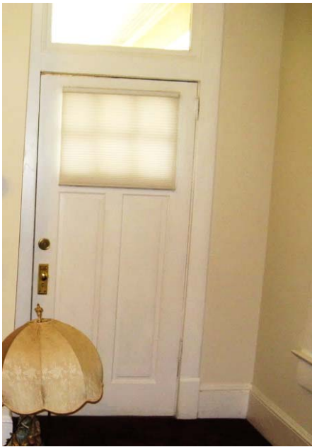
FIGURE 81. Secondary front porch entry door in north office.
