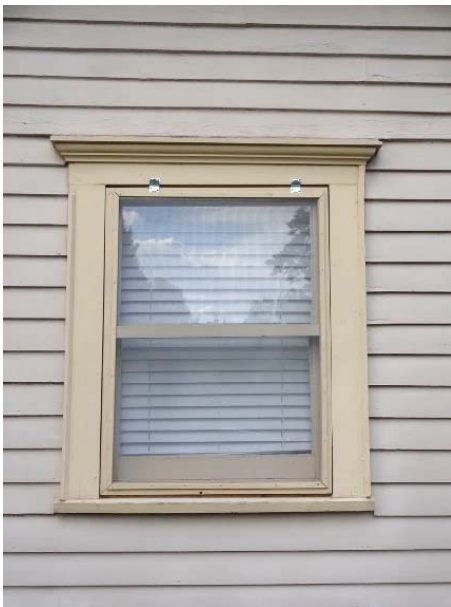
FIGURE 38. Typical window at south elevation.
