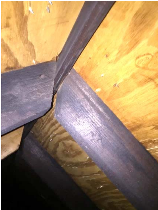
FIGURE 103. Detail of rafter-to-ridge beam interface.
