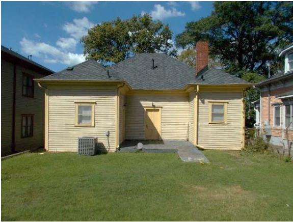
FIGURE 70. Rear elevation facing south. Note two subordinate hipped-roof projecting rooms.
