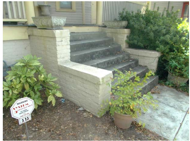
FIGURE 30. Concrete stair with brick cheek walls at main entrance porch.
