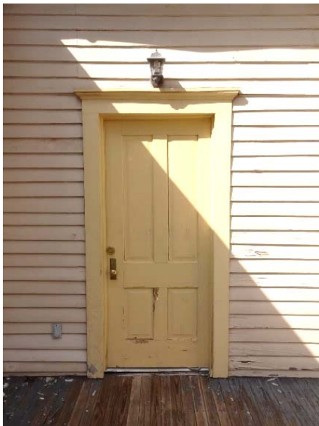
FIGURE 35. Door opening centered on south elevation, accessed from patio.
