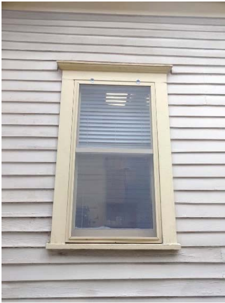
FIGURE 37. Typical window at east and west elevations.
