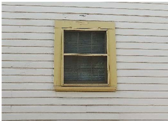
FIGURE 45. Modified six-over-six double-hung window at kitchen.
