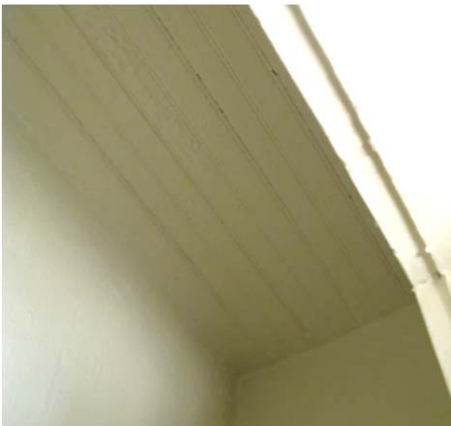
FIGURE 79. Textured plaster and beaded ceiling at upper unit closet.
