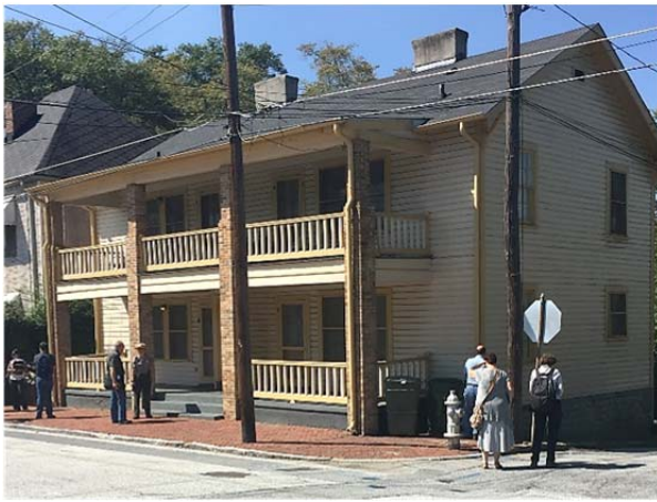
FIGURE 47. Overview of building showing gable roof with shed roof at the front porch.
