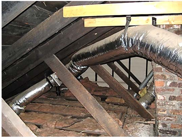
FIGURE 113. Overall view at attic.
