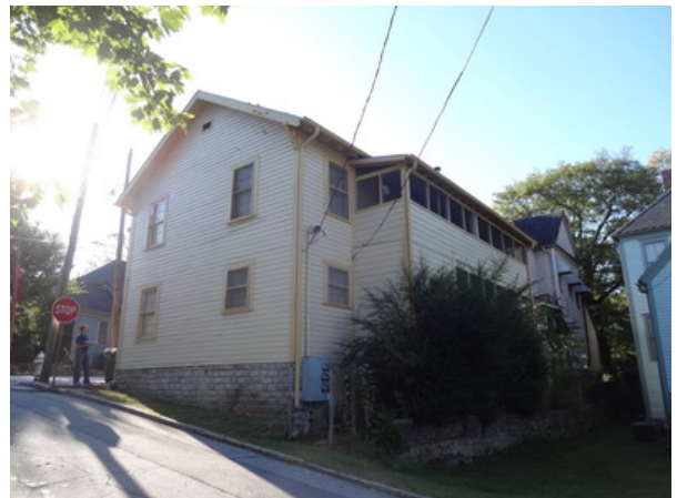
FIGURE 10. Overall view of the building looking southeast.
