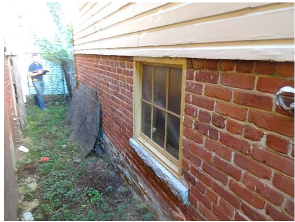
FIGURE 46. Fixed window unit at south elevation of basement.
