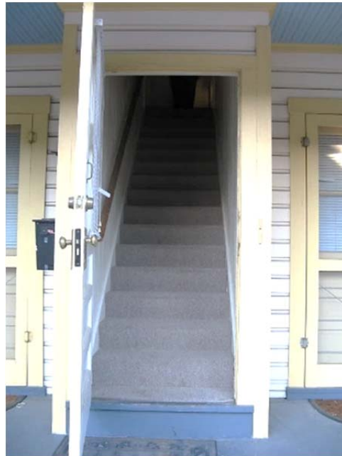
FIGURE 86. Front stair vestibule.
