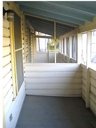
FIGURE 77. Demising wall at second-floor rear porch.
