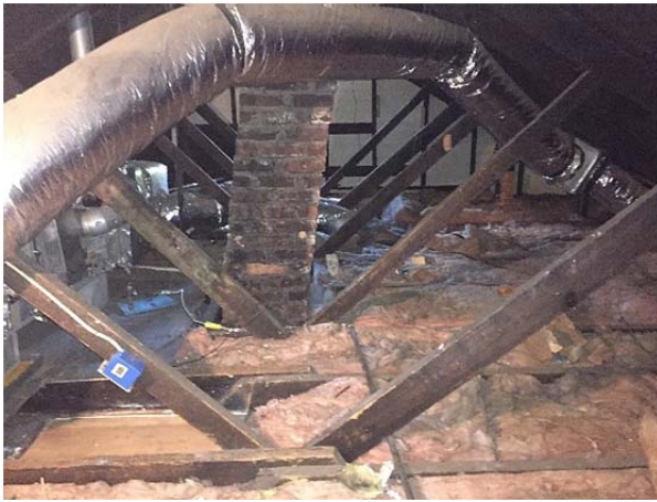
FIGURE 126. Overview of roof framing.
