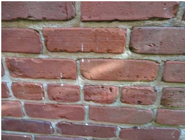
FIGURE 19. Red clay brick foundation visible from west and south elevations.
