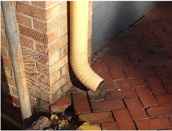
FIGURE 52. The circular sheet-metal downspouts discharge at grade.
