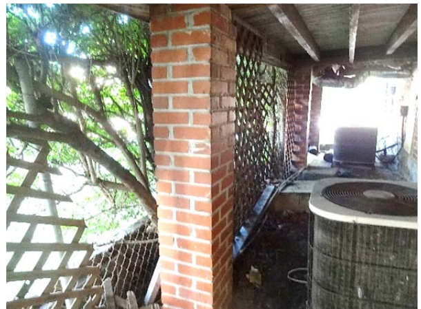
FIGURE 130. Typical brick pier that supports the rear porch.
