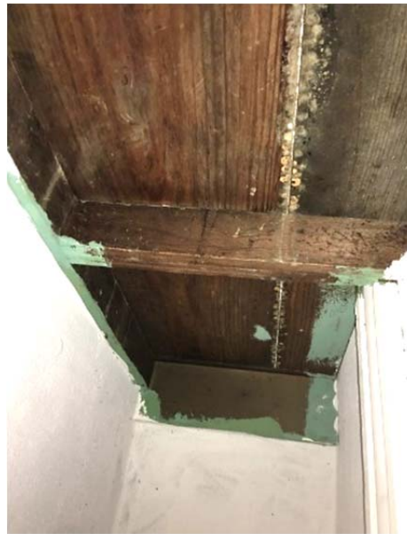
FIGURE 96. Underside of cabinet at dining room.
