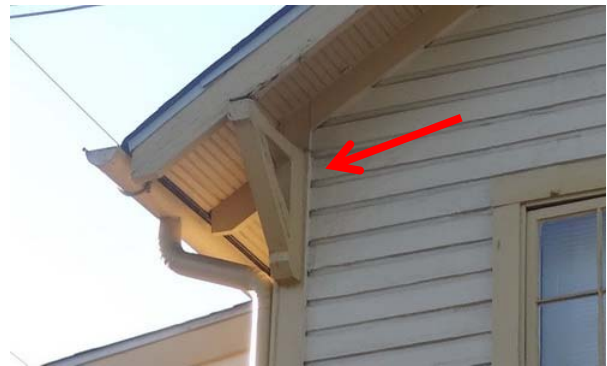
FIGURE 25. Wood brackets at gable roof eaves.
