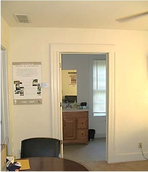
FIGURE 111. Non-original door to the bathroom from the living room of the north apartment.
