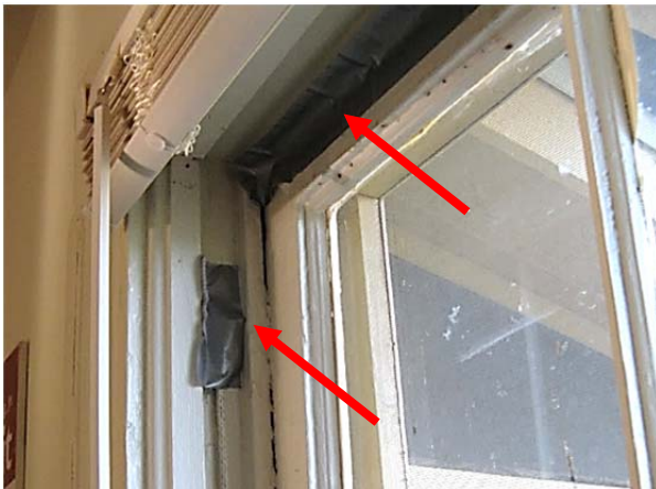
FIGURE 120. Tape covering points of air infiltration at perimeter of sash.
