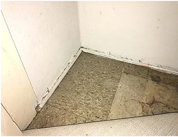
FIGURE 97. Original plaster wall and non-original VCT flooring at cabinet interior.
