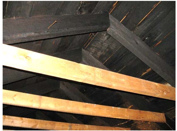
FIGURE 129. Non-original collar ties at roof framing.
