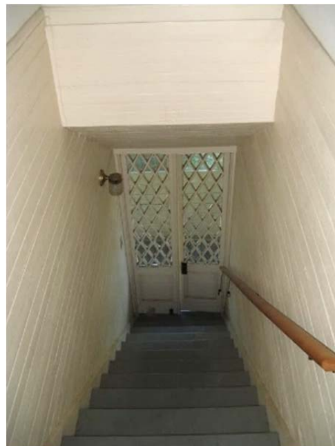
FIGURE 89. Rear stair with horizontal beaded siding and diamond lattice lights at doors below.
