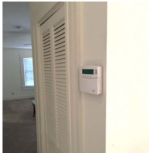
FIGURE 91. Reworked closet below front stair at connection between north and south lower units.
