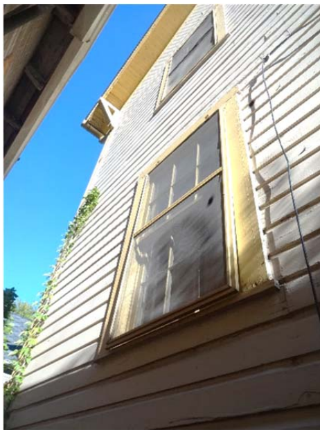
FIGURE 17. Partial view of the south elevation.
