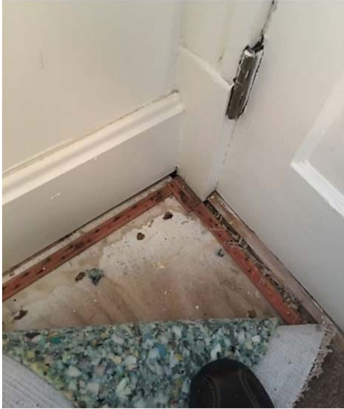
FIGURE 81. Plywood subfloor with carpet at the lower unit.
