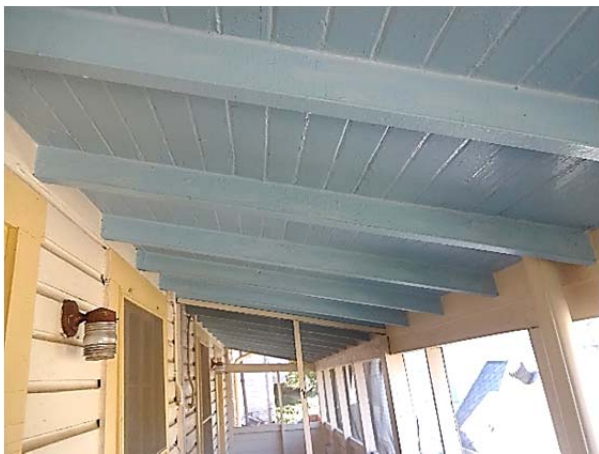
FIGURE 132. Wood roof framing for the rear porch is exposed to view.
