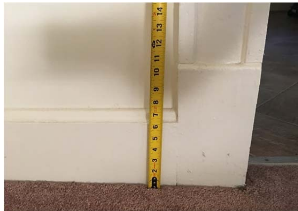
FIGURE 80. Typical baseboard and door plinth at first floor.
