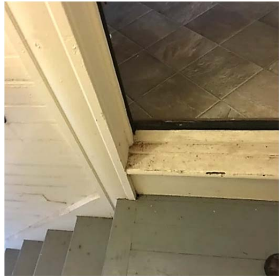
FIGURE 88. Threshold at kitchen door to rear stair.
