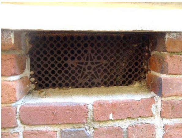
FIGURE 20. Decorative cast-iron vent grate at south elevation of foundation.
