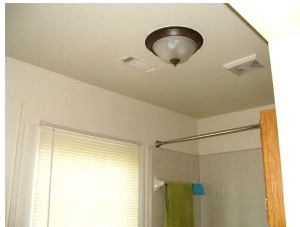
FIGURE 112. Non-original ceiling and fixtures at the north apartment bathroom.
