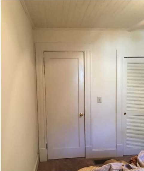
FIGURE 99. The relocated bedroom door (left) and remodeled closet (right) at south bedroom.
