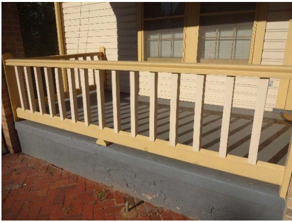
FIGURE 31. Wood balusters at front entrance porch.
