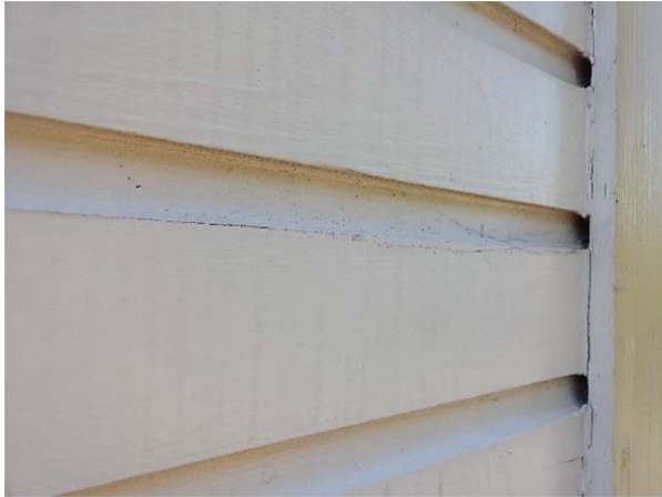
FIGURE 23. Typical horizontal shiplap wood siding at main portion of building.
