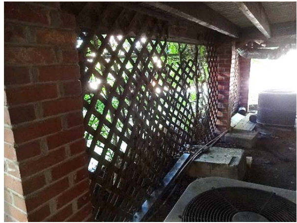
FIGURE 32. Wood lattice at enclosed rear porch.
