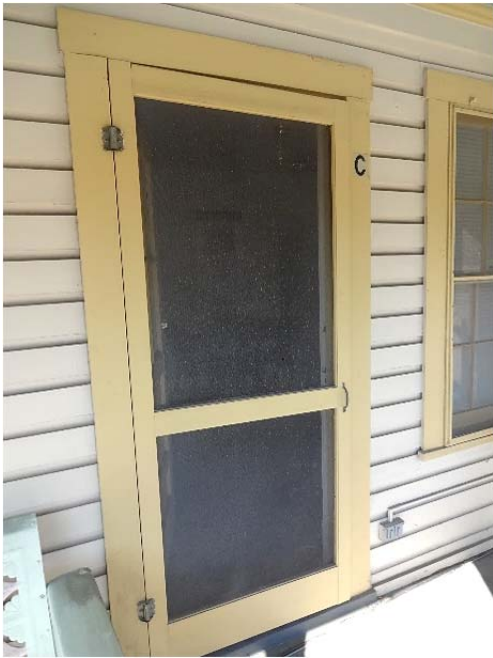
FIGURE 37. Typical screen door at exterior entrances.
