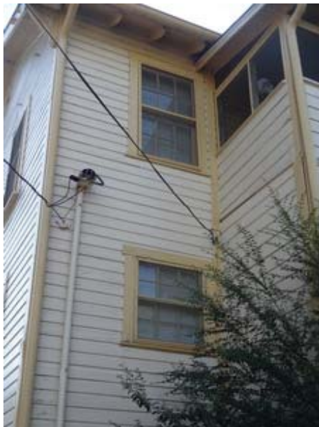
FIGURE 24. Corner between main building (left) and partially enclosed rear porch (right). Note differences in width of siding.
