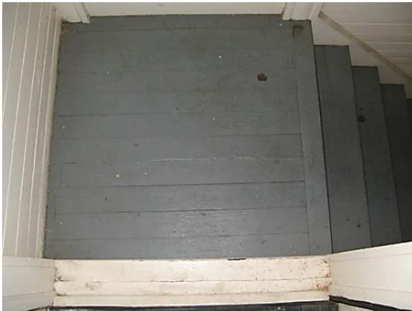
FIGURE 82. Painted tongue-and-groove wood flooring at rear stair landing.
