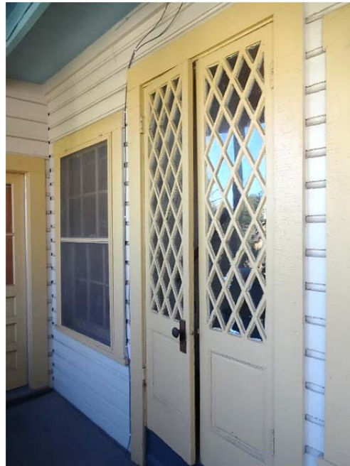
FIGURE 40. Wood-framed double door with diamond-shaped glazing at west elevation of the building.
