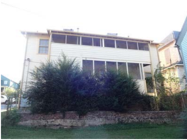
FIGURE 16. West elevation with the two-story partially enclosed porch.
