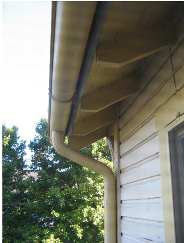
FIGURE 5. Exposed, dog-eared rafter tails on 54 Howell Street.
