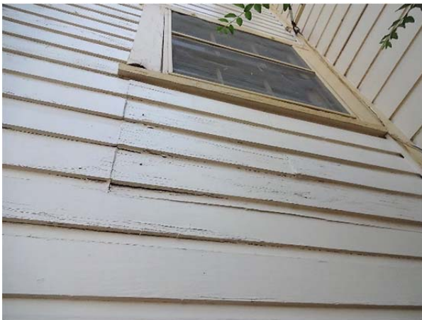
FIGURE 72. Infill siding below kitchen window opening.
