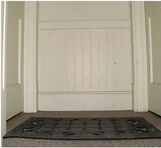
FIGURE 87. Wainscot at upper landing of front stair.
