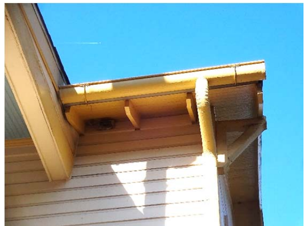
FIGURE 51. View of half-round hanging gutter and downspout.
