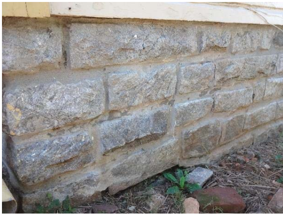
FIGURE 18. Coursed ashlar granite foundation at north elevation of building.
