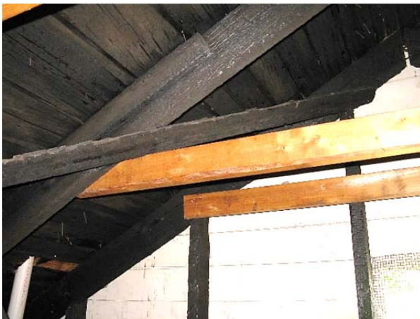
FIGURE 127. Diagonal cross bracing at roof framing.
