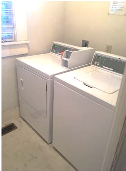
FIGURE 102. Coin-operated washer and dryer in the shared laundry.
