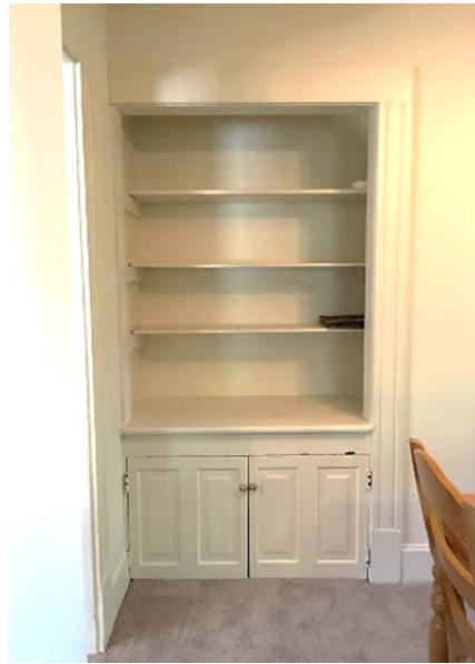
FIGURE 95. Original built-in shelving and cabinet at dining room.
