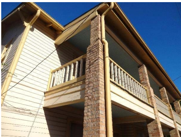
FIGURE 28. Brick piers at front entrance porch.
