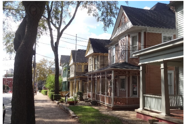
FIGURE 9. Overview of the Auburn Avenue streetscape looking west at the Martin Luther King, Jr. National Historical Park.
