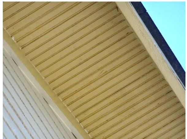
FIGURE 49. Underside of the eaves with the non-original bead board decking exposed to view.
