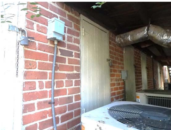
FIGURE 42. Wood-plank access doors to basement area.
