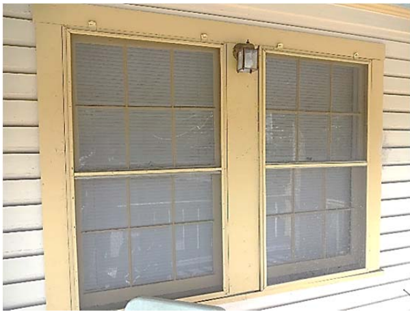
FIGURE 43. Typical paired six-over-six double-hung window on the building.
