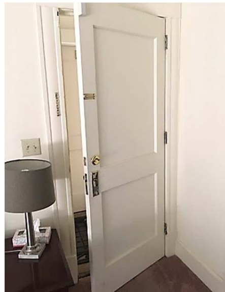
FIGURE 104. Two-panel door at entry to north apartment from the central stair.
