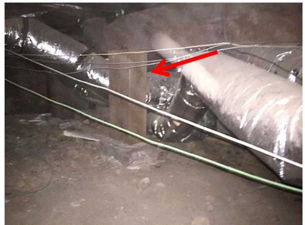
FIGURE 22. Wood posts on concrete cap provide supplemental support of the floor beams.
