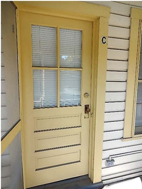
FIGURE 38. Typical wood-framed exterior doors at the east elevation of the building.
