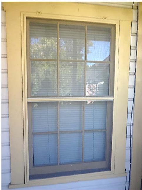
FIGURE 44. Typical six-over-six single double-hung.
