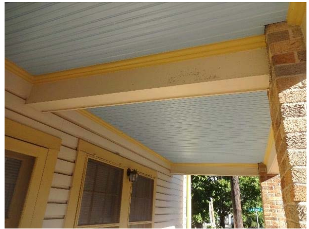
FIGURE 29. First-floor ceiling, including wood box beam, at front entrance porch.
