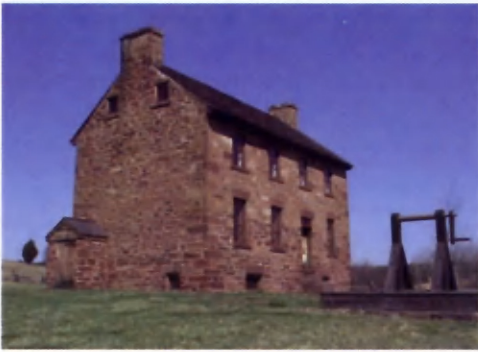
Stone House, tour stop 2 NPS/ Frank Harrell
