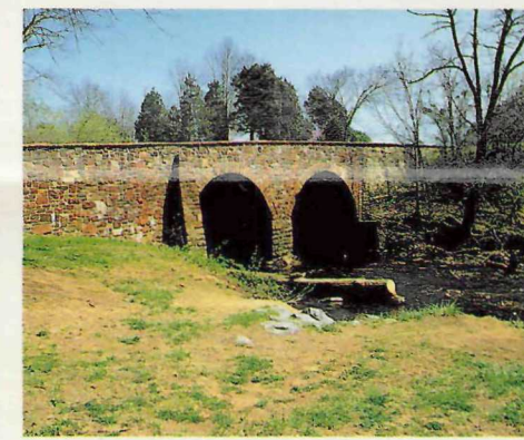
Stone Bridge, tour stop 12
