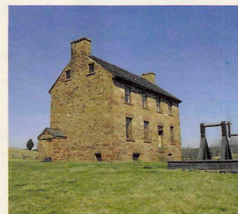
Stone House, tour stop 3
