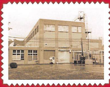
Building 9731, known as the "Pilot Plant," is the oldest process building at Y-12.
