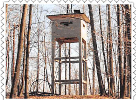
The last of the historic guard towers, built in 1948, stands on Pine Ridge, the north boundary of Y-12.
