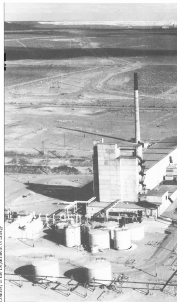
REDOX facility, early 1950s.
