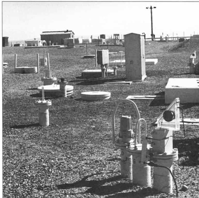
BELOW: Because the tanks themselves are six to ten feet below ground, the only parts visible on the surface are access covers, monitoring equipment and ventilation systems. Hanford technicians use equipment inserted through the access pipes to take samples of the waste in each tank, an important step in the program to ultimately empty the tanks—which were not designed for permanent storage—and convert the waste into a form safe for permanent disposal.
