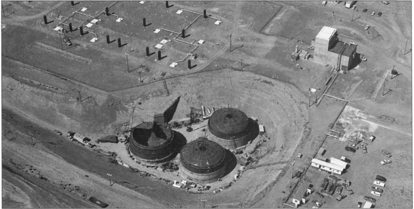
ABOVE: Hanford's best-known waste tank, 101-SY, is closest to the bottom of this 1974 photograph. It has received much attention in the past few years because of concerns that gases generated by and accumulated within the waste might be flammable. Solving this issue is the United States Department of Energy's top priority.
