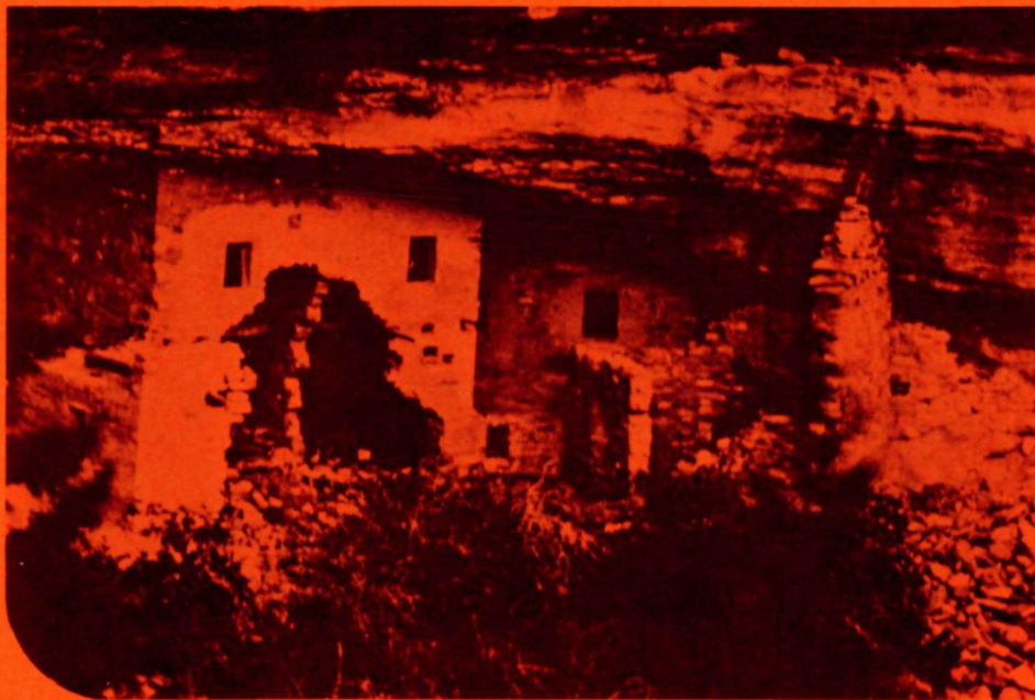
Courtyard wall before reconstruction.
