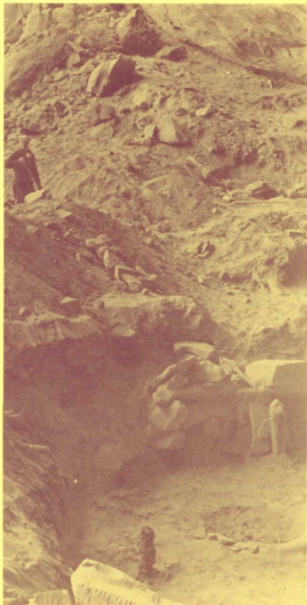
1926 excavation in Step House under the direction of Supt. Jesse Nusbaum.
