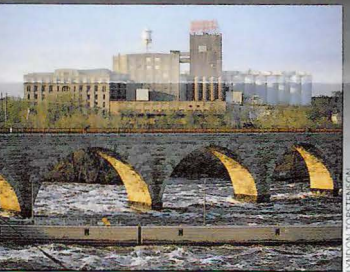
Stone Arch Bridge is a National Engineering Landmark and part of the Saint Anthony Falls Heritage Trail. It offers pedestrians, bicyclists, and joggers magnificent views of the falls. Waterpower from the falls made Minneapolis the nation's milling capital from 1880 to 1930.
